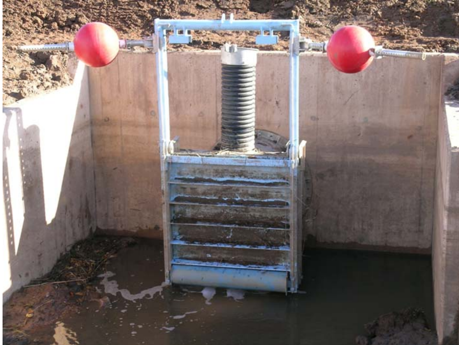
Figure D.18 Self regulating tidegate imported from the USA (copyright AJ Bellamy)
