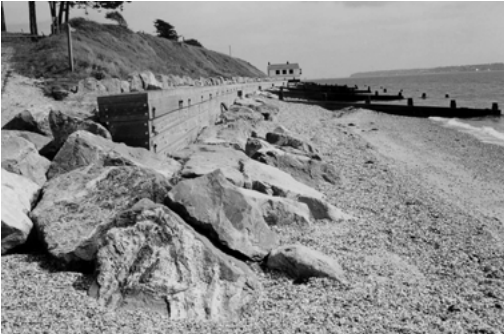
Figure 8.8. Timber bulkhead with rock toe protection at Lepe, Hampshire (courtesy HR Wallingford)
