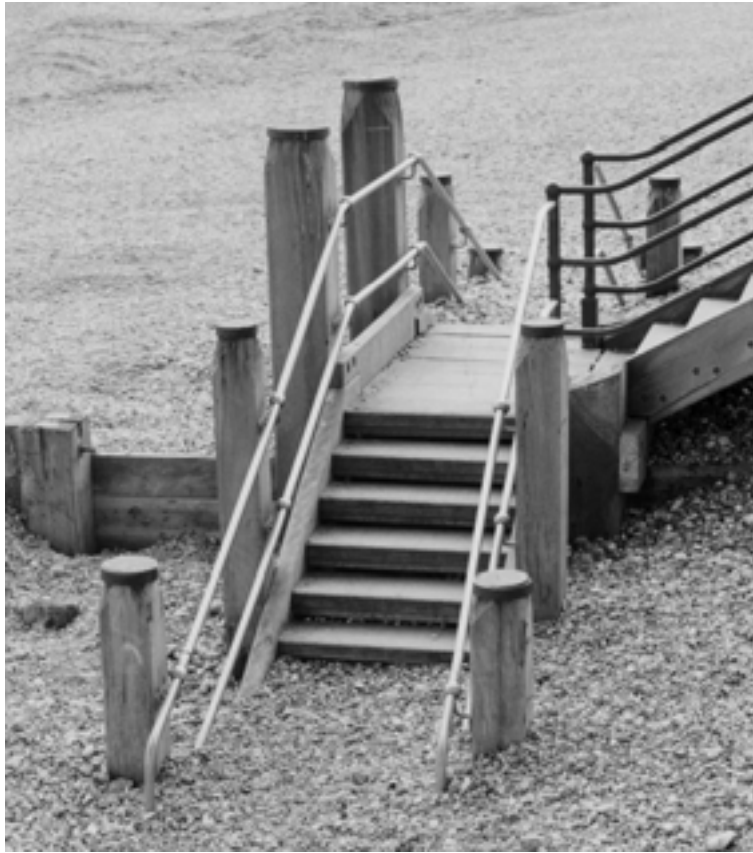
Figure 8.21. Purpleheart access steps at Eastbourne, East Sussex (courtesy HR Wallingford)
