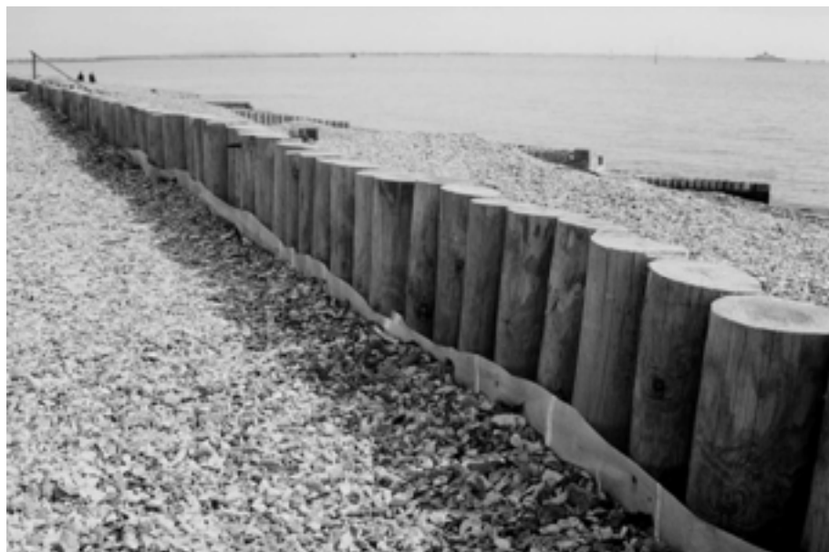
Figure 8.13. Low cost revetment with geotextile at Calshot, Kent (courtesy HR Wallingford)
