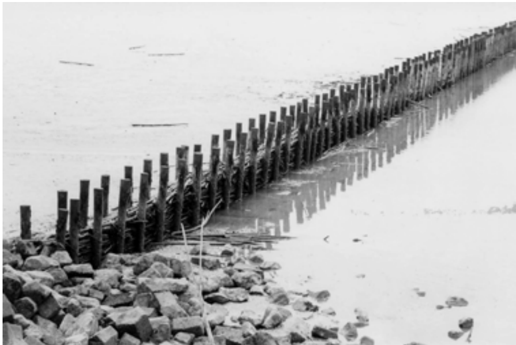
Figure 8.31. Accreting faggot, Holwerd, The Netherlands (courtesy HR Wallingford)
