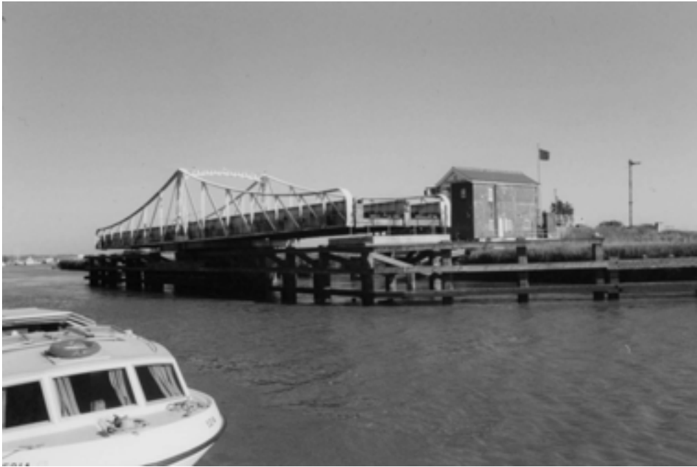
Figure 8.24. Timber piled lead-in structure to protect bridge pier at Reedham, Norfolk (courtesy Clive Orbell-Durrant)
