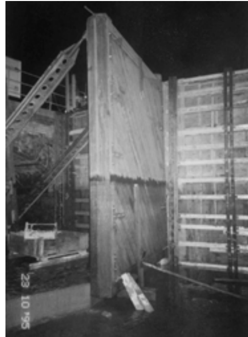
Figure 8.29. Vertically-hinged, twin-leaf gate (courtesy Babtie Group)
