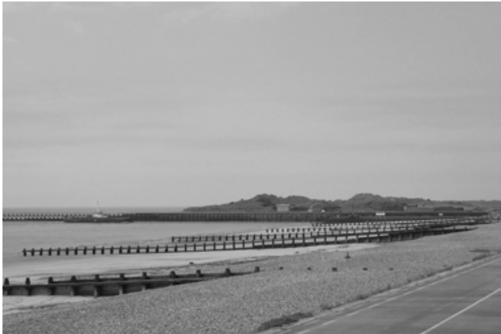
Figure 8.1. Conventional impermeable timber groyne field (courtesy Arun District Council)
