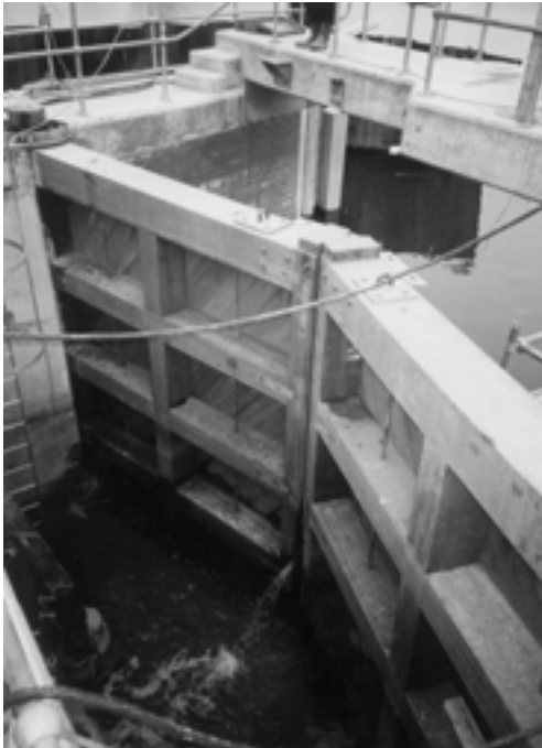
Figure 8.28. Lymington tidal flap gate (courtesy Babtie Group)
