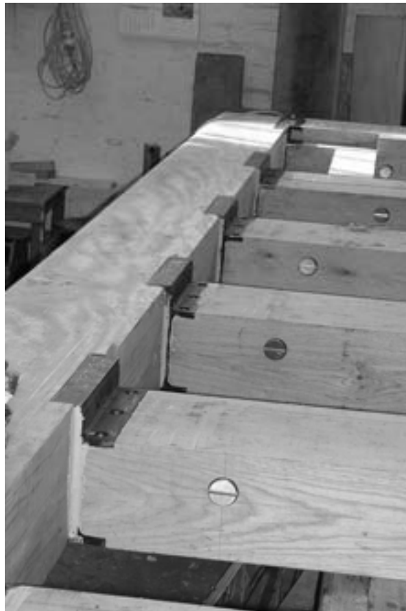
Figure 8.27. New joint for timber lock gates developed by British Waterways (a) joint detail and (b) as implemented in a lock gate in the workshop (courtesy British Waterways)
