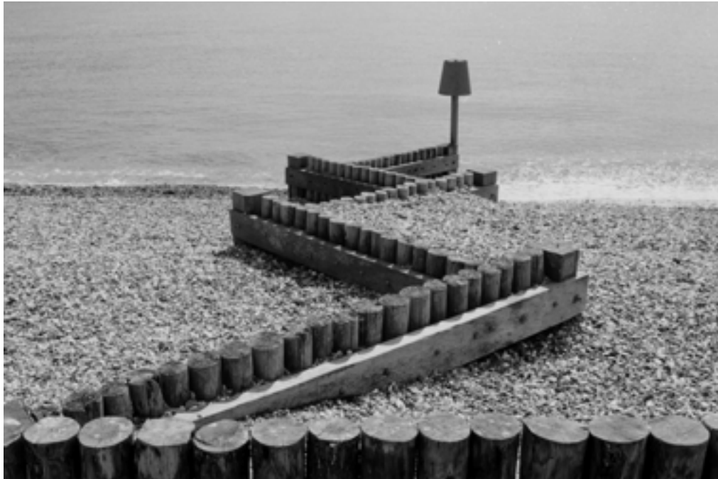
Figure 8.3. Low cost groyne, Calshot, Hampshire (courtesy HR Wallingford)
