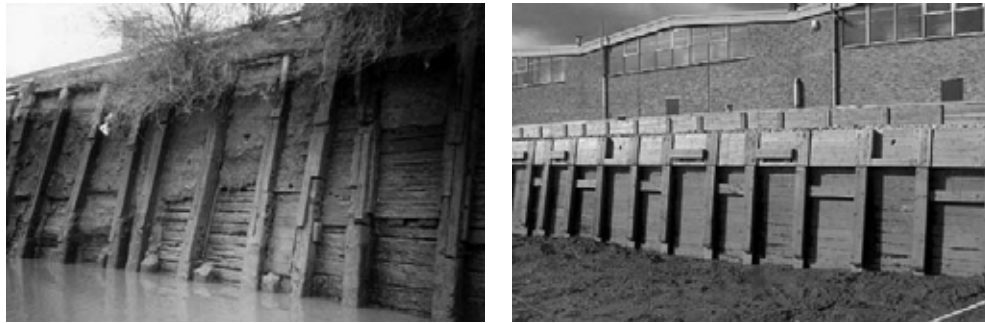
Figure 8.38. Deptford Creek frontage before (left) and after (right) (courtesy Babtie Group)
