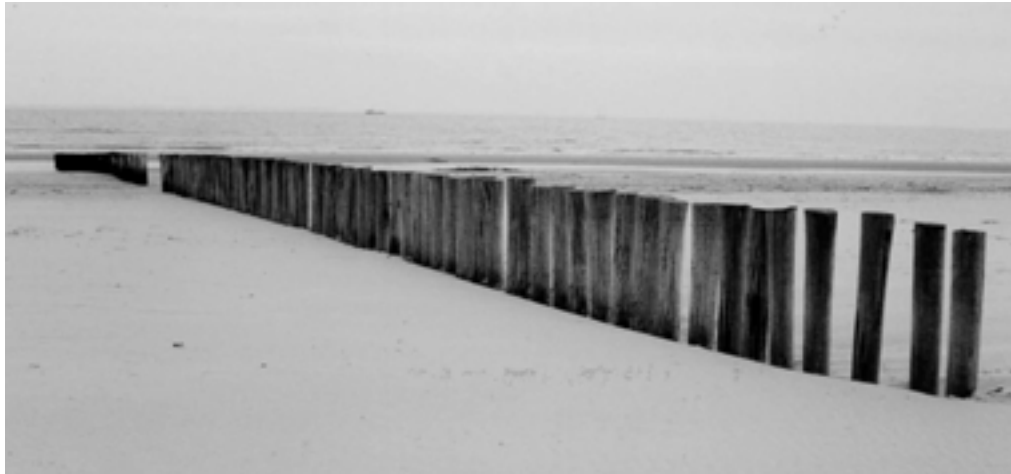
Figure 8.2. Pile groyne at Ameland, The Netherlands (courtesy HR Wallingford)
