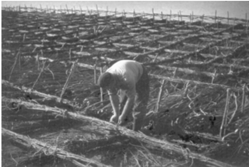
Figure 8.30. Construction of a fascine mattress (courtesy Henk Jan Verhagen)
