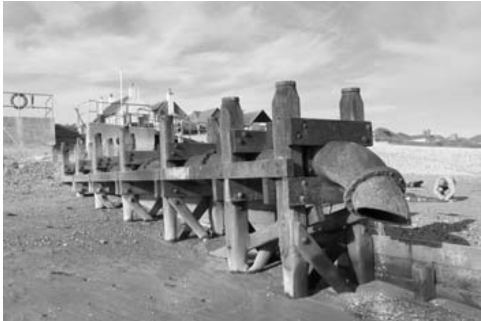
Figure 8.18. Support trestle for outfall, East Wittering, West Sussex (courtesy Posford Haskoning)
