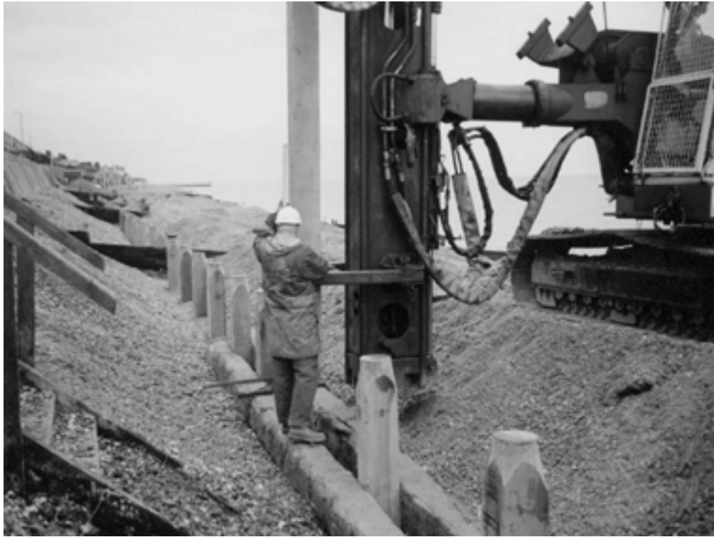
Figure 8.9. Construction of a timber breastwork (courtesy Mackley Construction)
