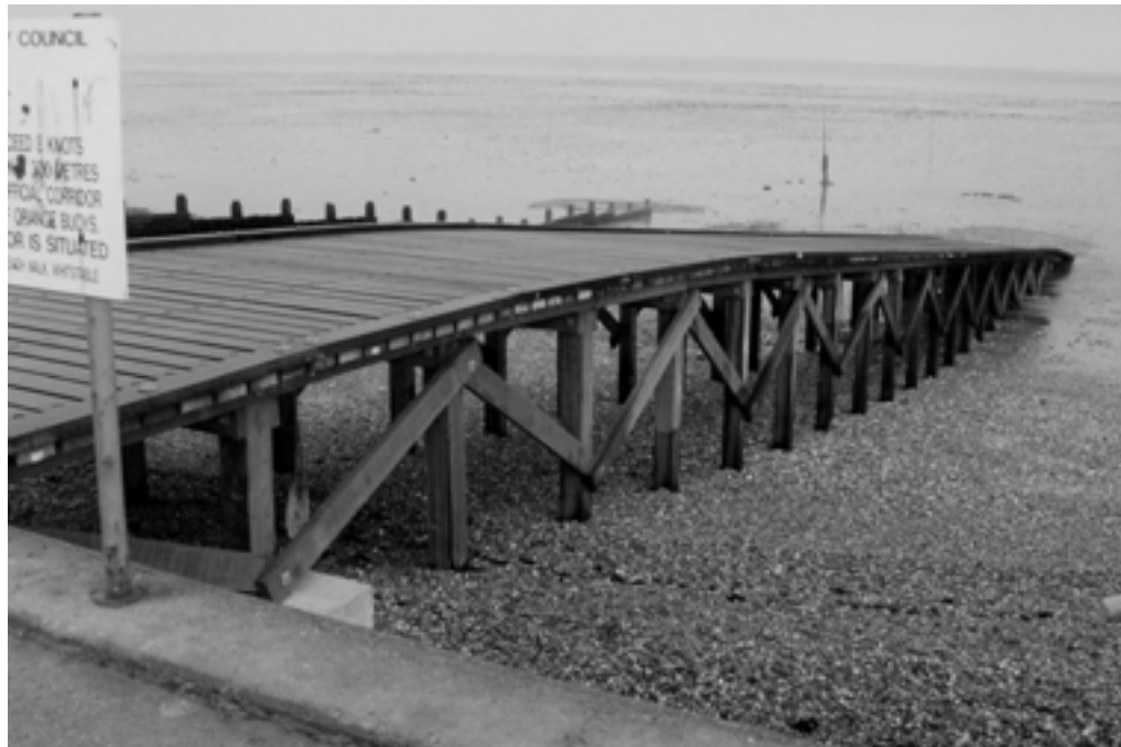
Figure 8.20. Ekki boat ramp at Tankerton, Kent (courtesy Mackley Construction)
