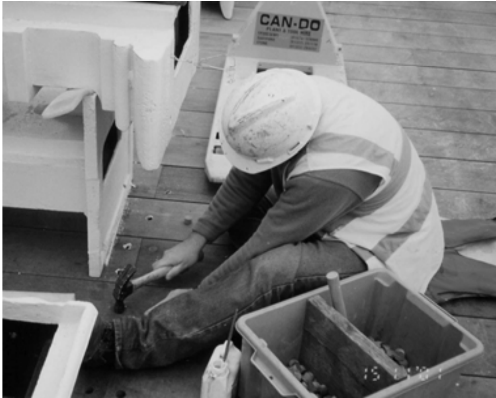
Figure 8.17. Covering decking fixings with wooden plugs (courtesy HR Wallingford)
