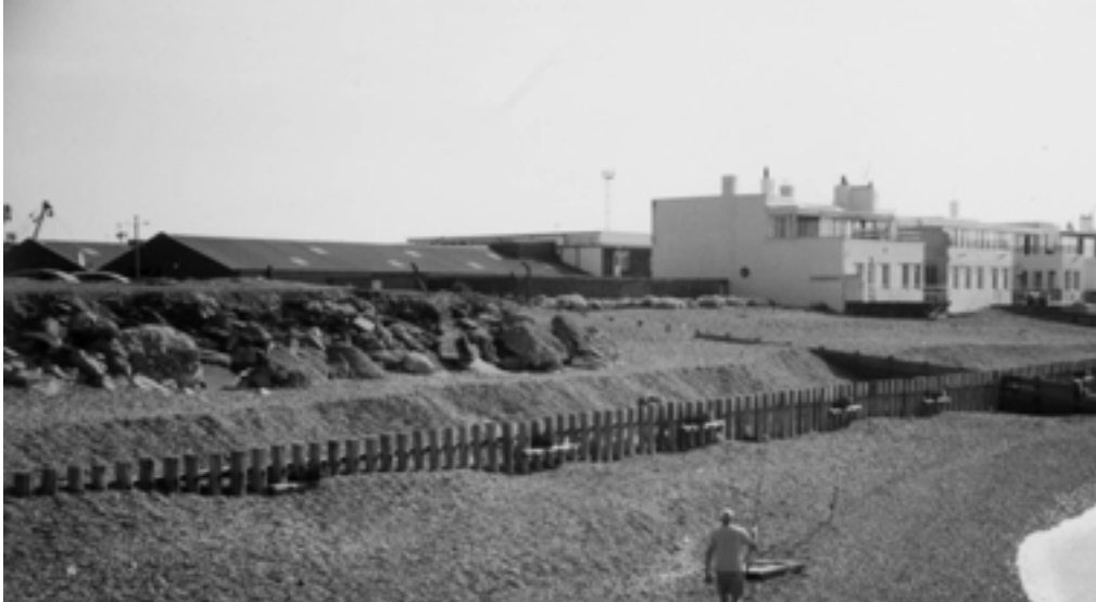
Figure 8.11. Vertical breastwork at Shoreham, West Sussex (courtesy Shoreham Port Authority)
