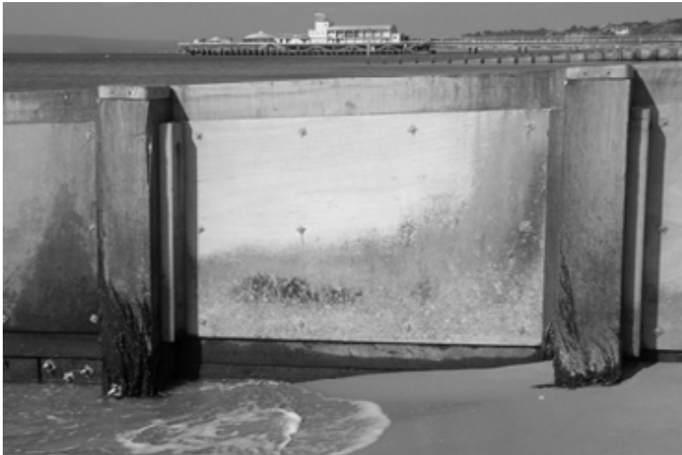
Figure 10.2. Use of plywood backing to groyne planks at Bournemouth (courtesy Bournemouth Borough Council)
