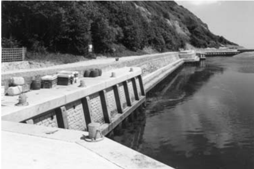
Figure 8.23. Timber fenders at Axmouth Harbour (courtesy Posford Haskoning)
