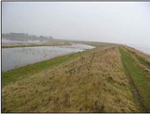
Landward embankment face
