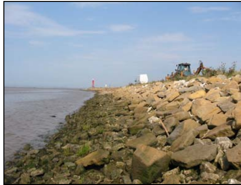
Seaward embankment face
