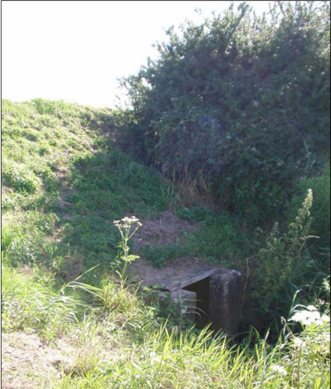
Plate A2.33 Typical small culvert structure passing through embankment
