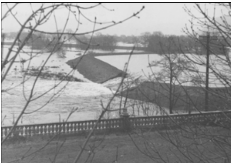
Plate D11.2 Breaching of flood embankment along the River Conway
