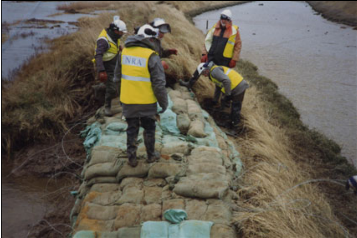
Plate D11.3 Breach repair on River Blyth in 1993
