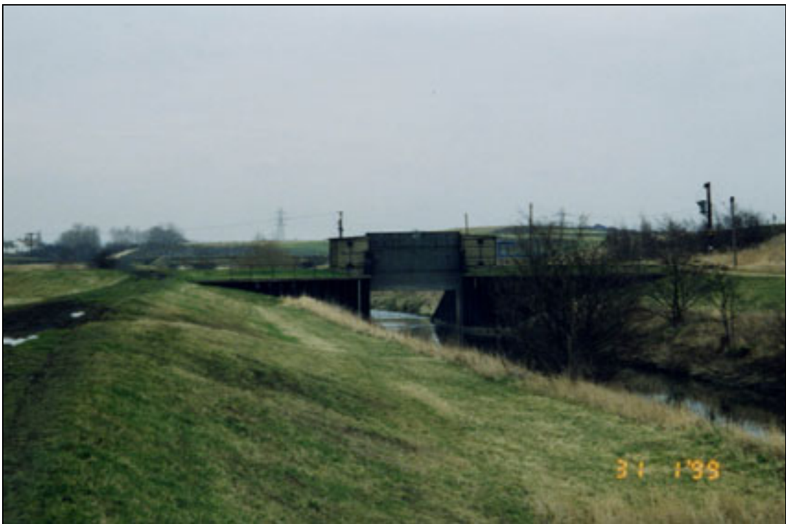
Plate A2.39 Control structure across entire channel
