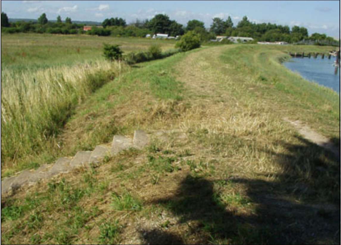
Plate A2.46 Stepped access on outward face of embankment
