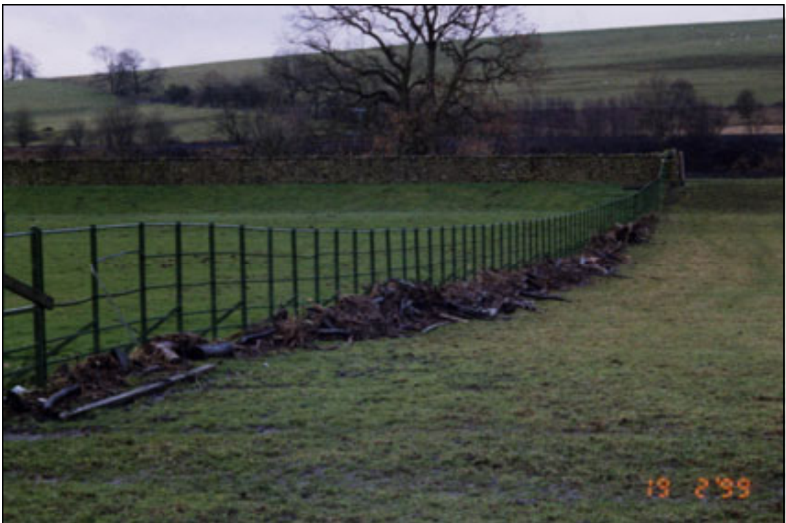
Plate A2.50 Fencing constructed across washland spillway
