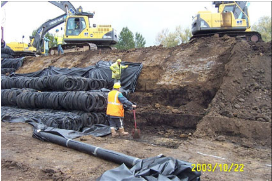
Plate B4.1 Excavation and placing of tyre bales
