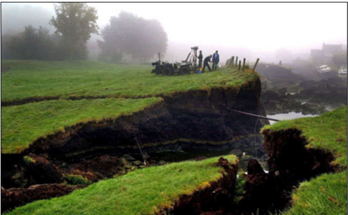
Plate B3.19 Translational block failure of embankment
