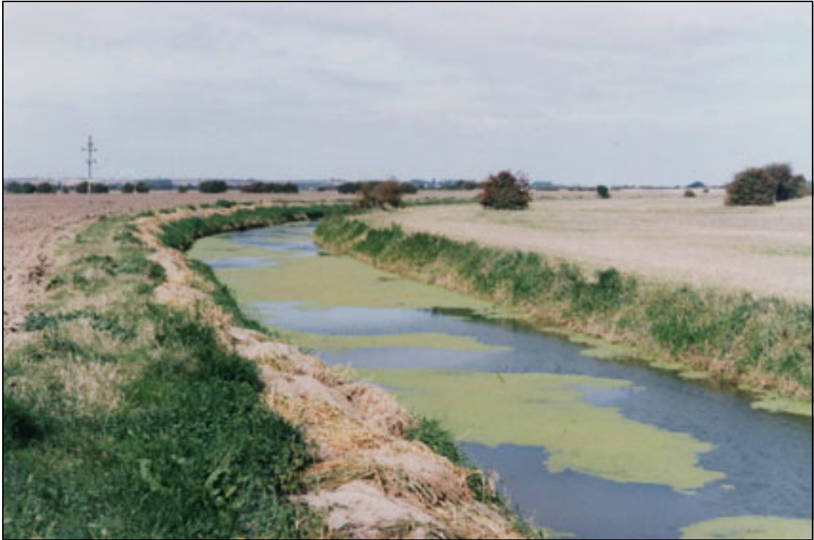
Plate B2.6 Weed cuttings dumped on inward face of embankment
