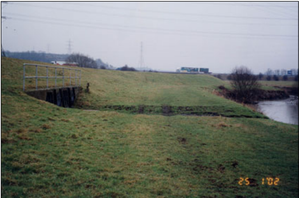
Plate A2.31 Outfall structure – inward face
