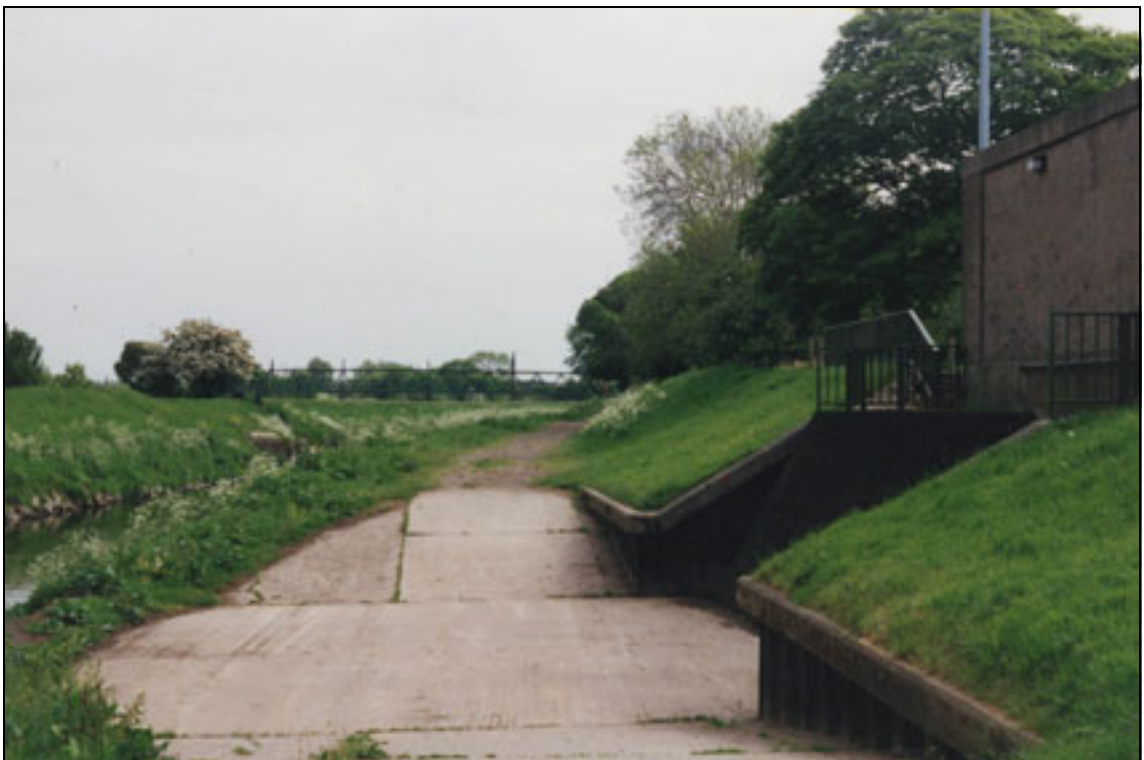
Plate A2.7 Control structure linking offline storage to main river
