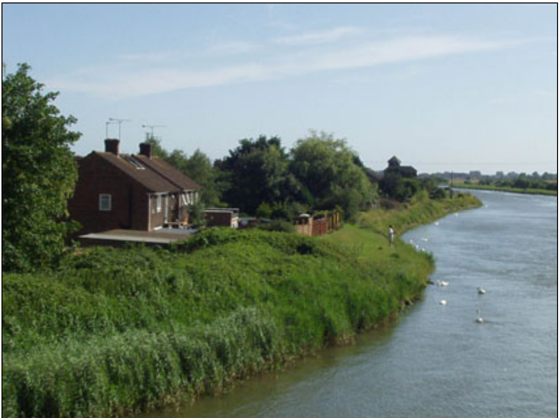
Plate A2.54 Housing constructed immediately behind embankment; garden extended across the embankment
