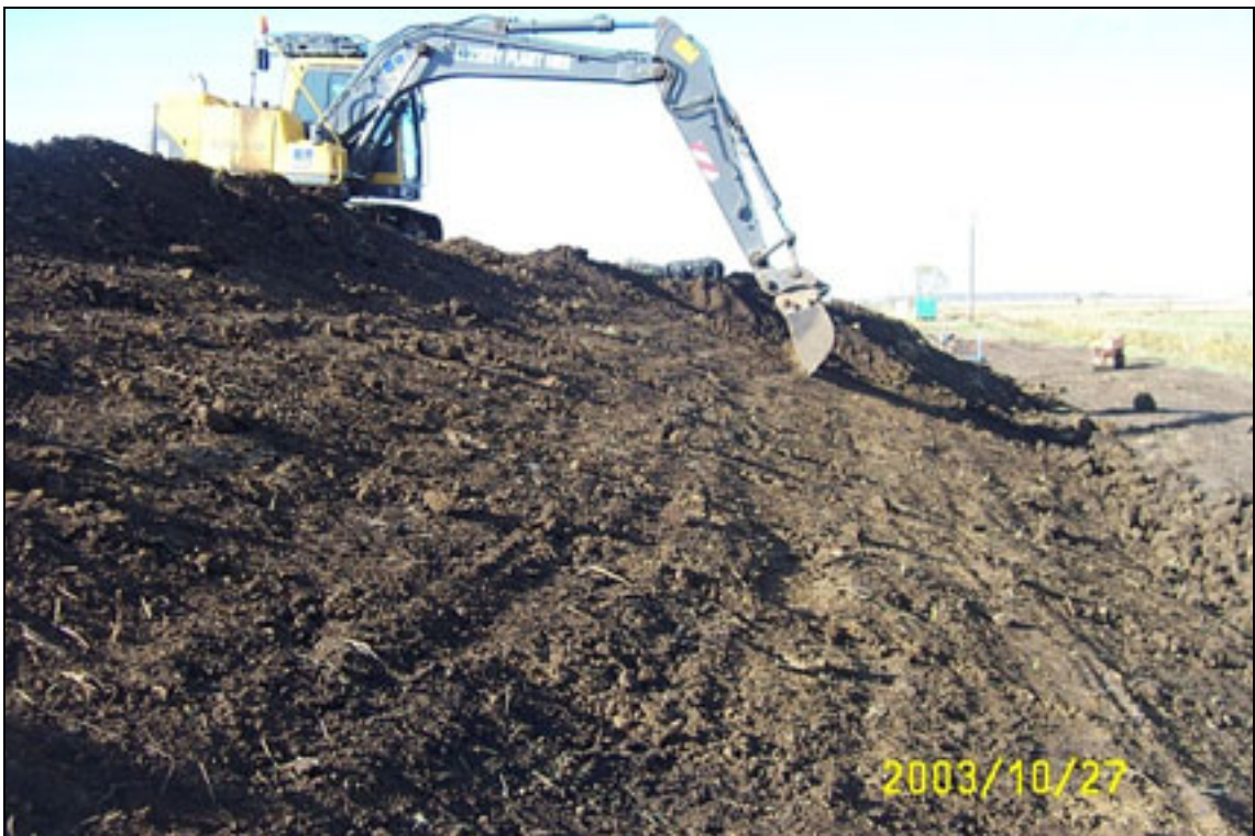
Plate B4.2 Embankment face covering tyre bales
