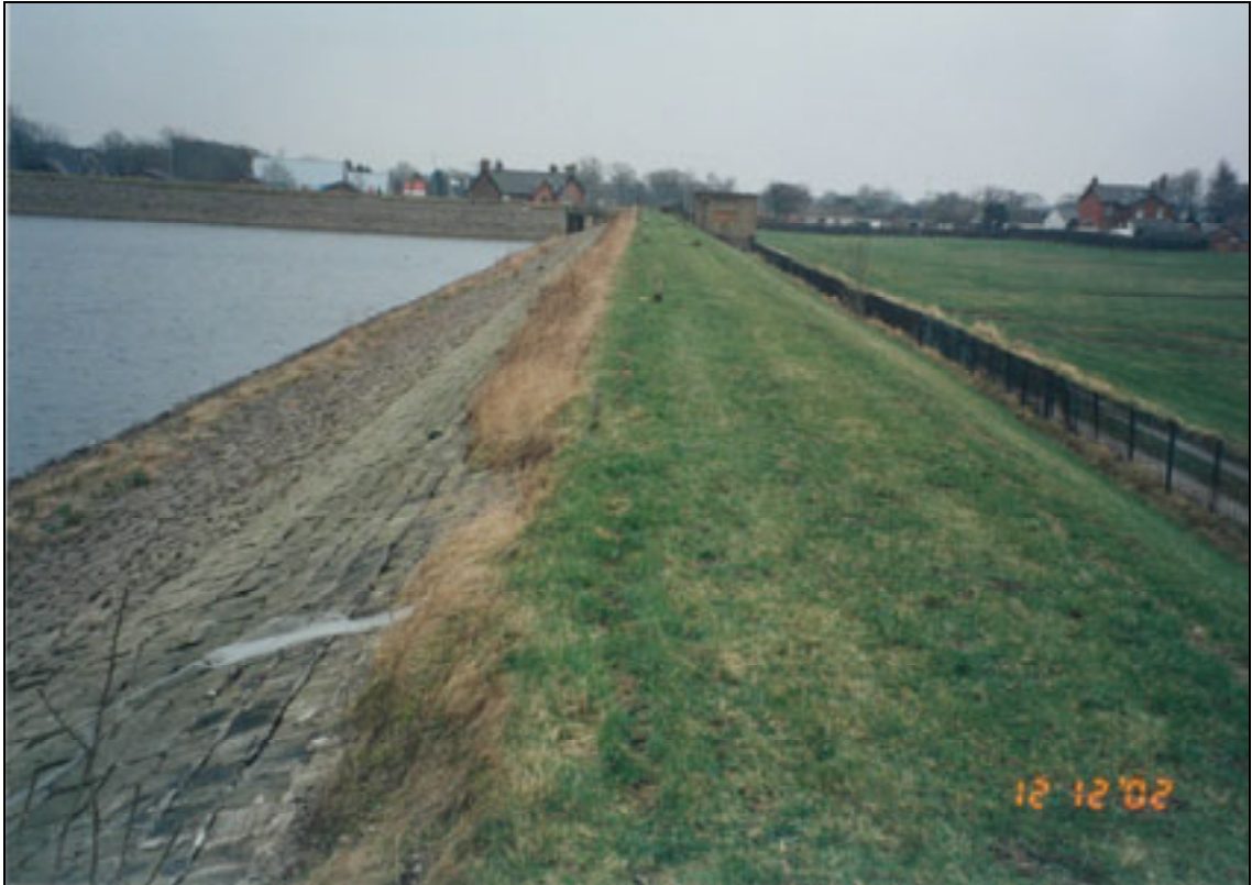
Plate A2.4 Reservoir embankment
