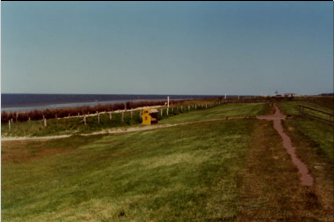
Plate A2.44 Stepped access onto embankment
