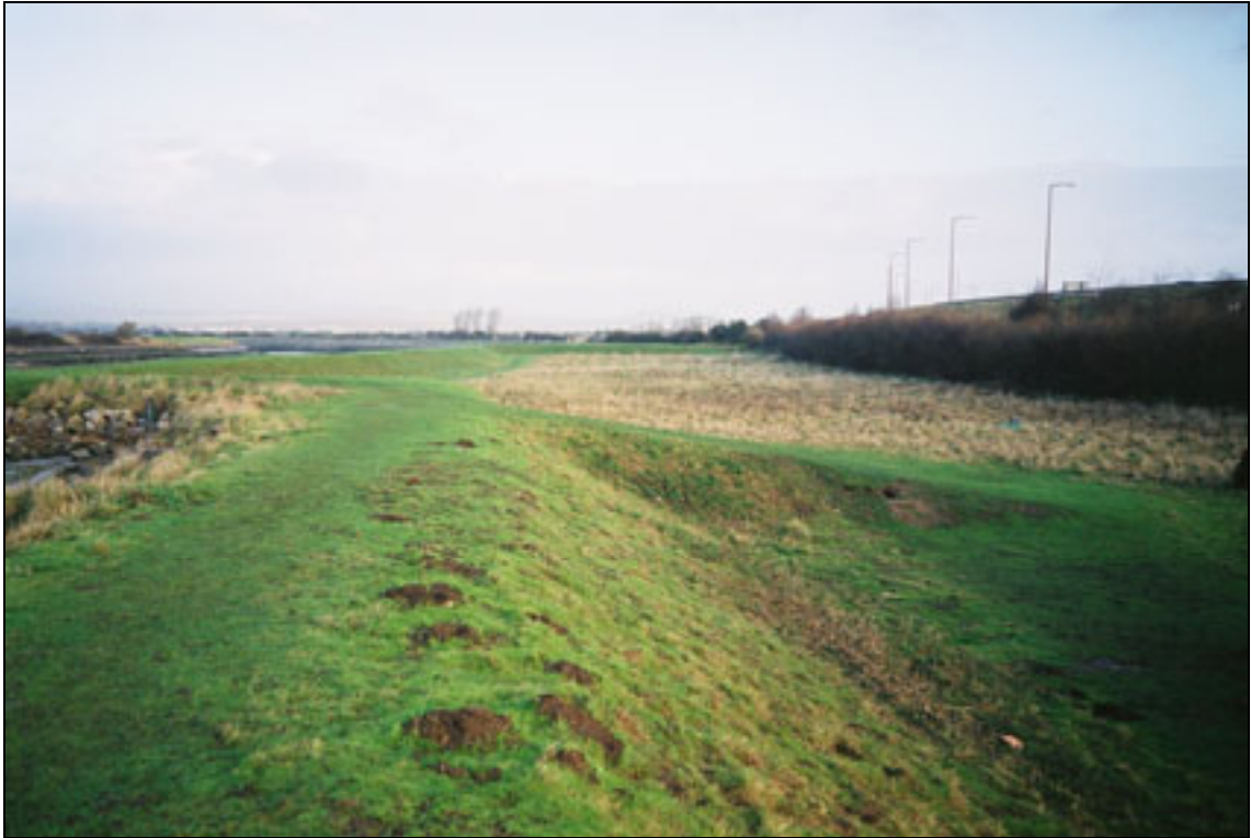
Plate A2.43 Ramped access onto an embankment
