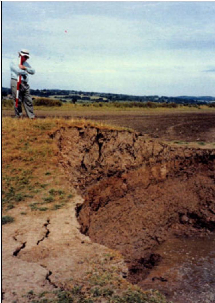
Plate A2.11 Rapid bank erosion, leading to undermining of defences
