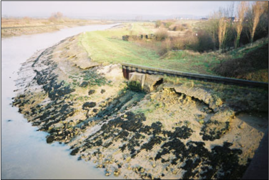
Plate A2.32 Outfall structure – tidal embankment
