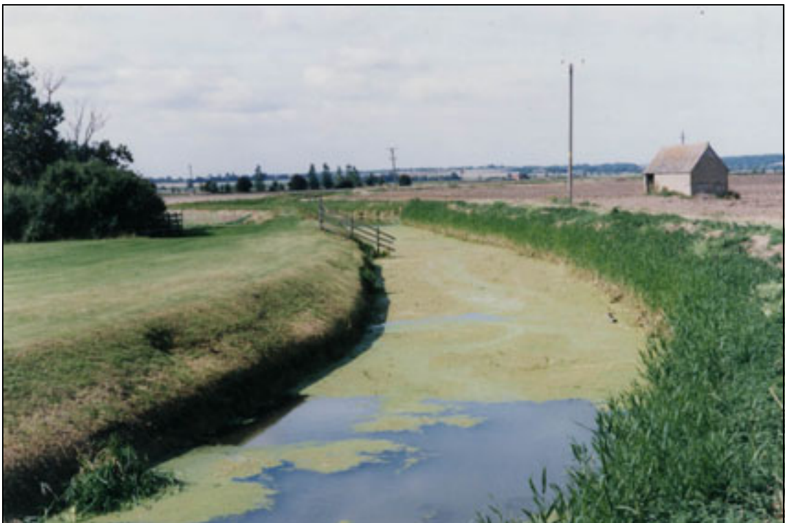
Plate B2.7 Different vegetation management on each riverbank (note fence protruding into channel)
