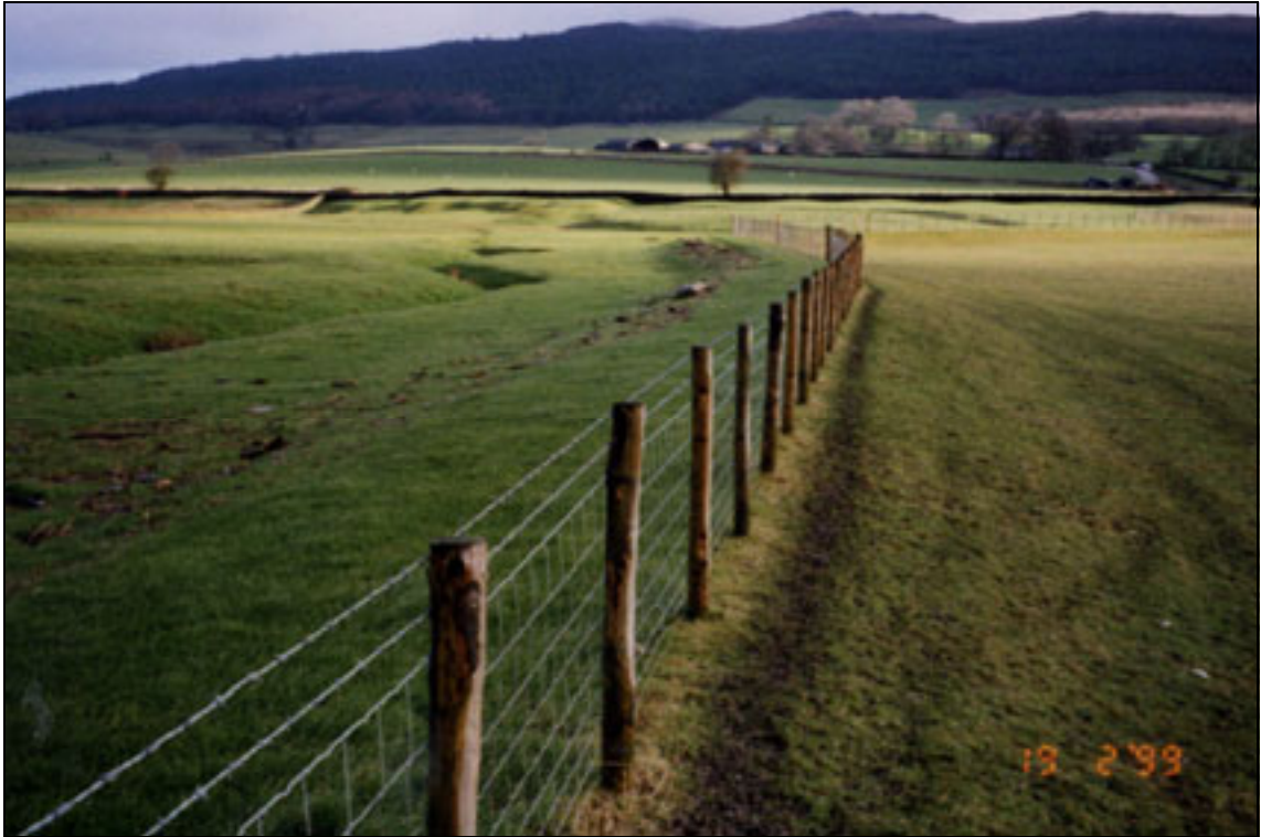
Plate A2.49 Fencing constructed along embankment
