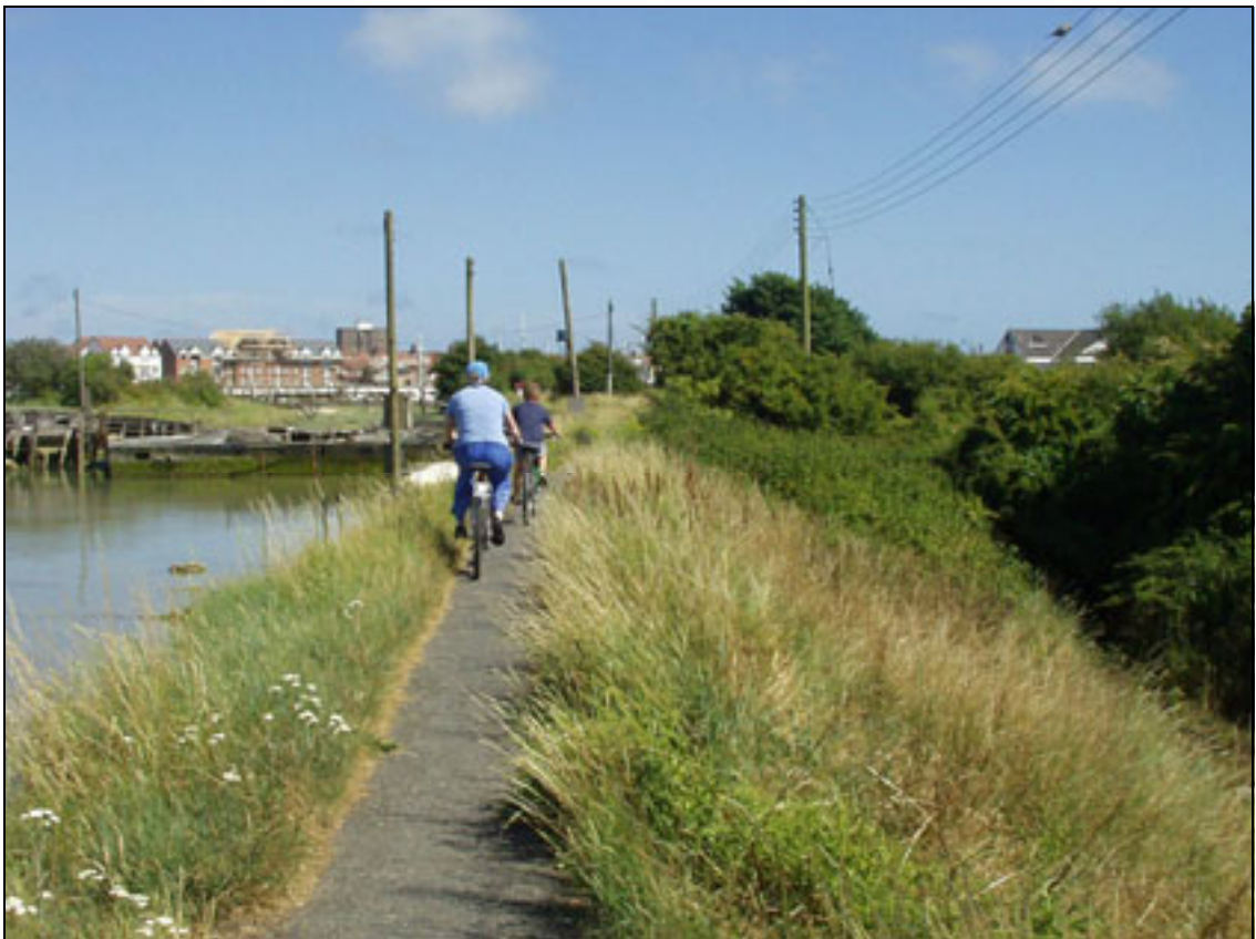
Plate A2.17 Recreational use of embankment (cycle route)
