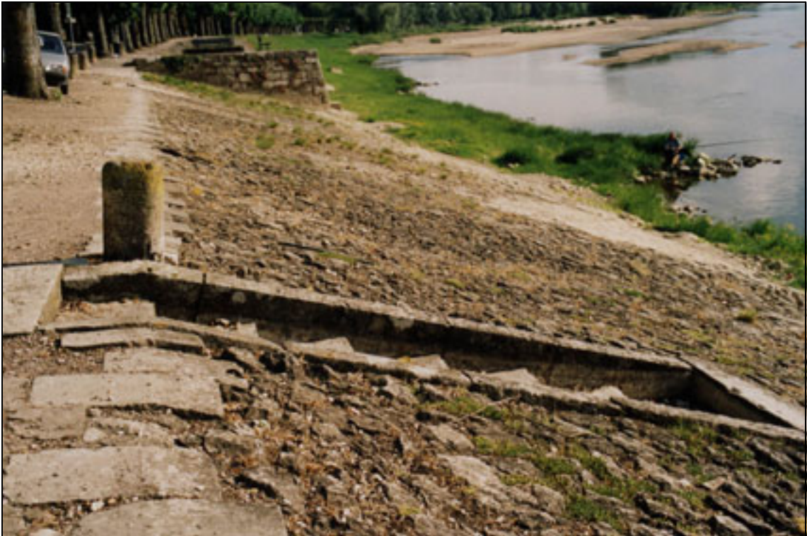
Plate A2.45 Stepped access on inward face of embankment
