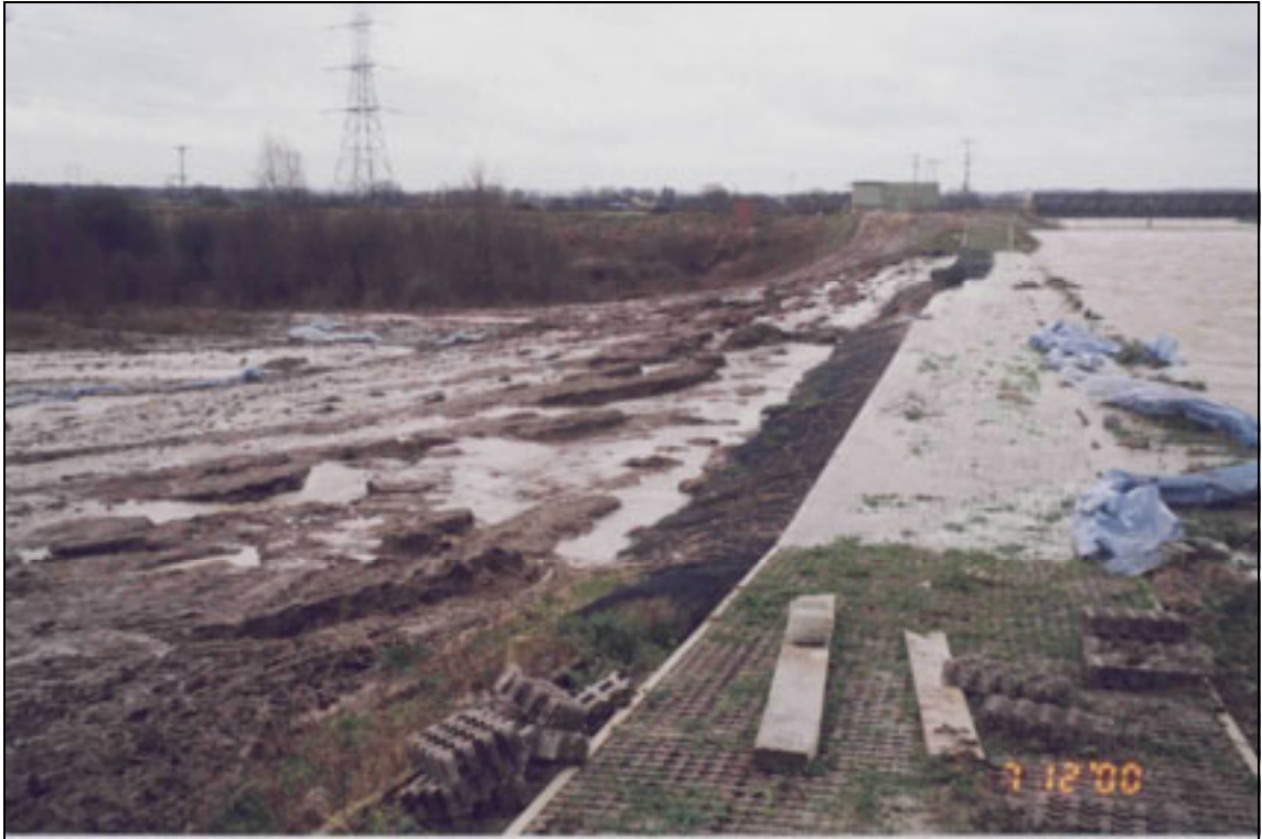
Plate A2.36 Overflow during construction
