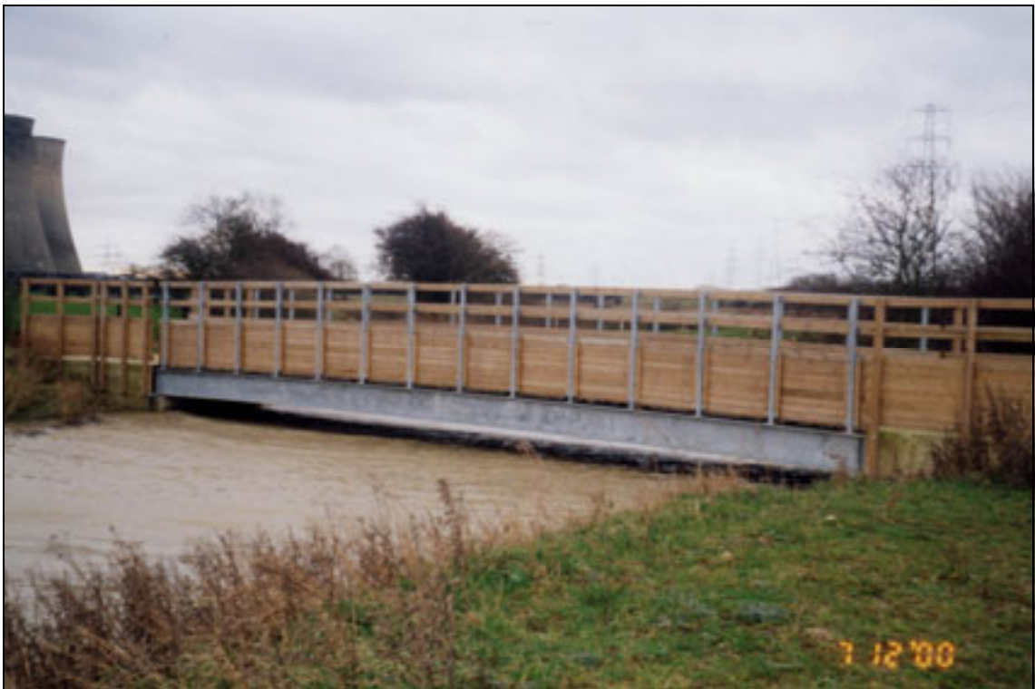
Plate A2.57 Interface between embankment and bridge abutment
