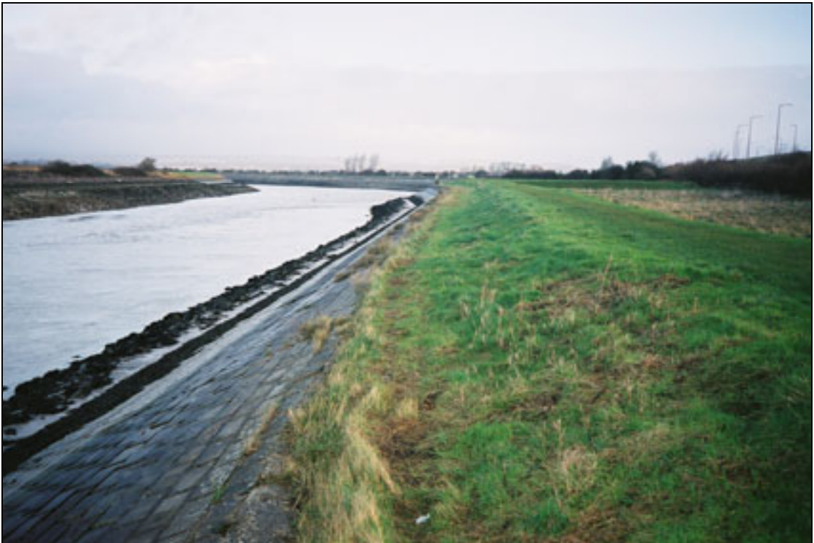
Plate B1.6 Concrete slab protection
