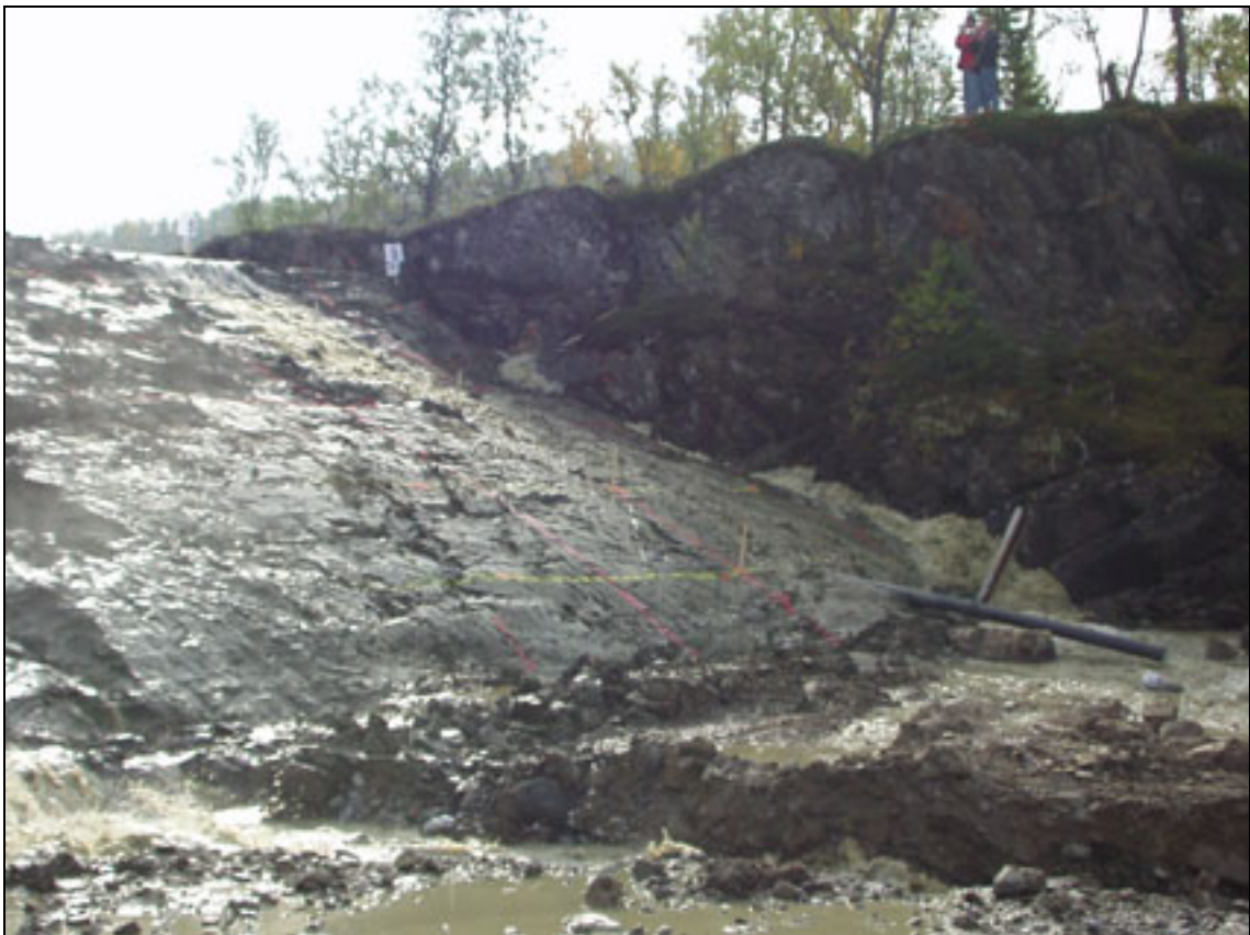
Plate D8.1 Piping through a test embankment alongside rock abutment (IMPACT Project – Field Test)
