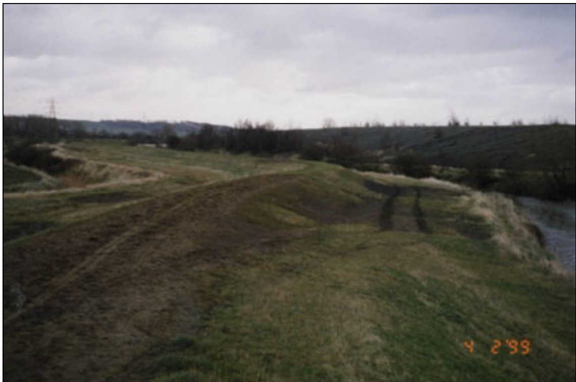
Plate A2.42 Parallel ramp access onto embankment crest
