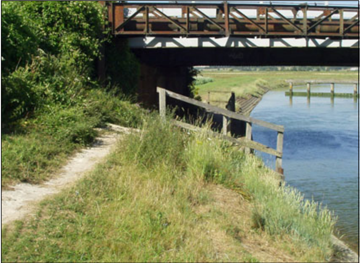
Plate A2.51 Fencing on inward face of embankment
