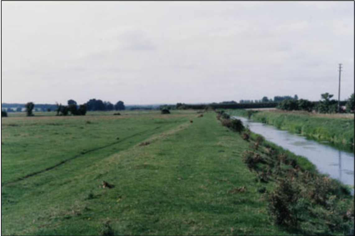
Plate B2.8 Higher vegetation growth within flow channel
