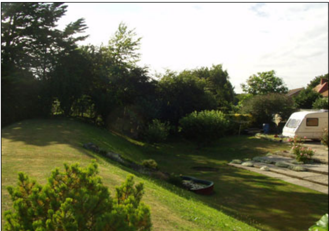
Plate A2.56 Embankment constructed within front garden of residential property
