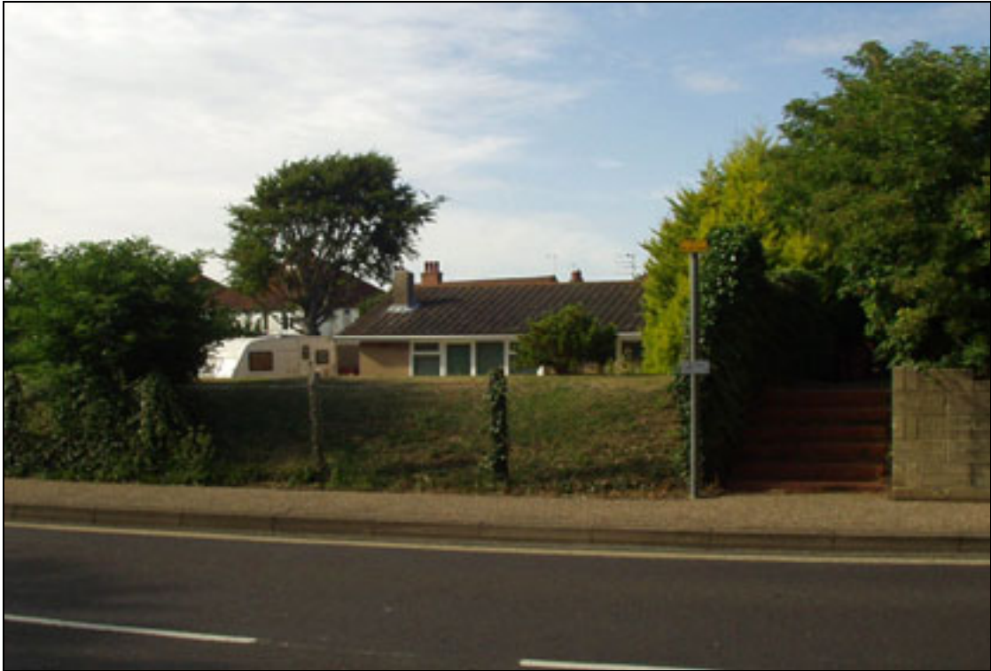
Plate A2.3 Flood embankment in front garden of house
