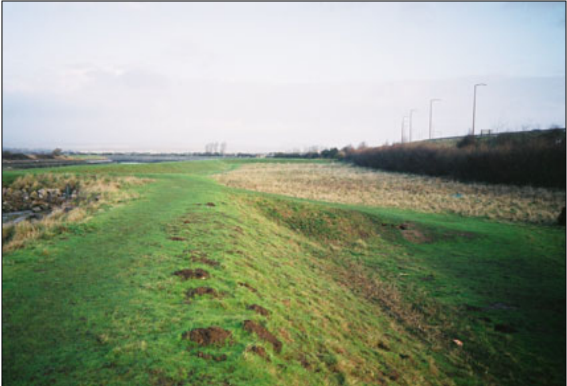
Plate A2.15 Ramped access to embankment
