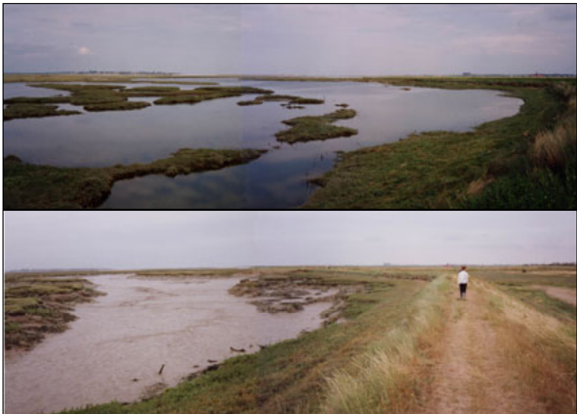
Plate A2.14 Estuary flood embankment behind saltmarsh
