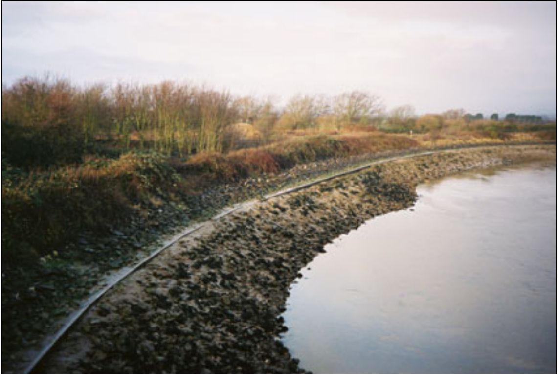
Plate B1.1 Rock protection with sheet piling to stabilise bank
