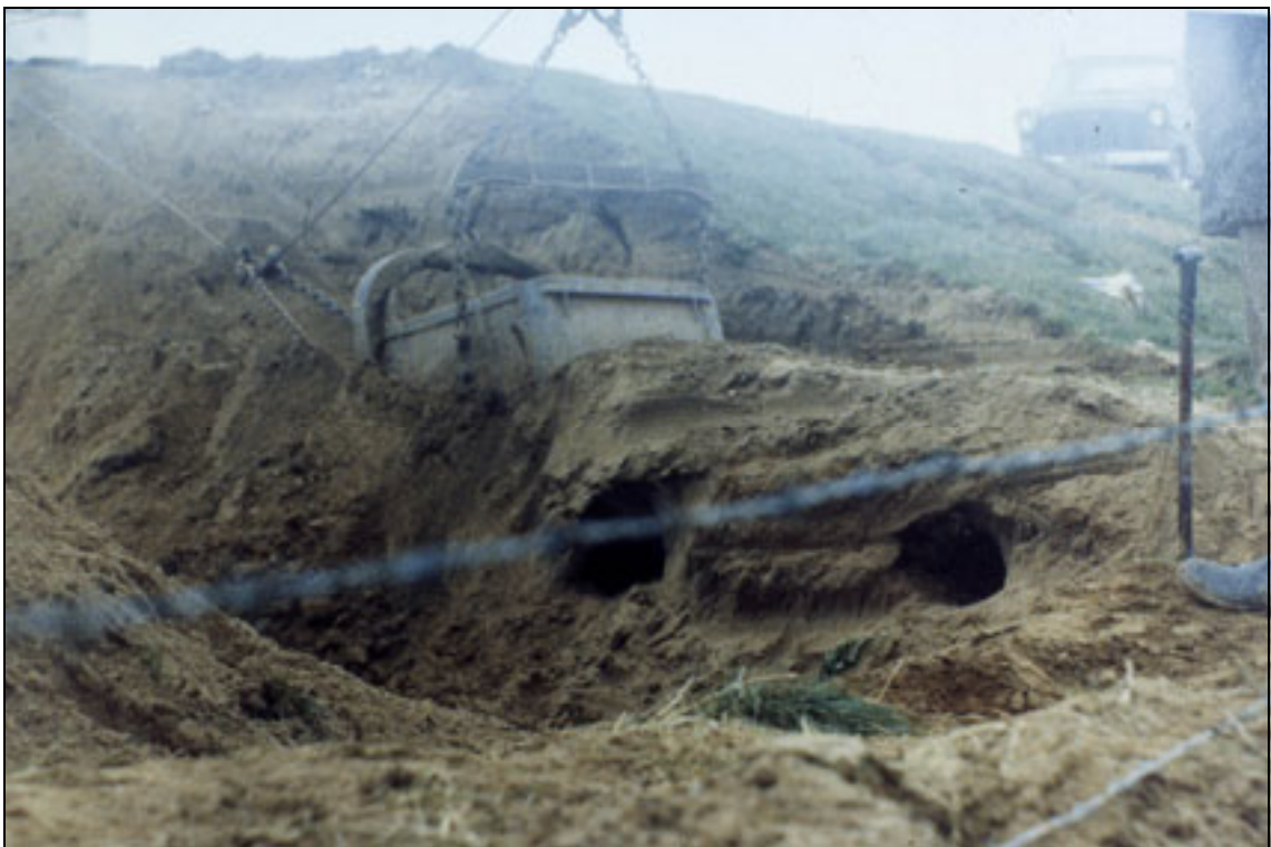
Plate A2.24 Uncovering a badger set burrowed into coastal embankment
