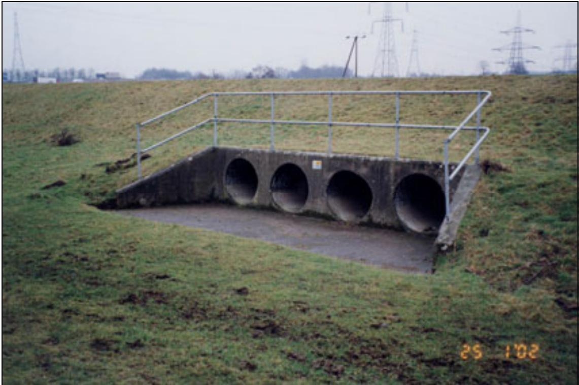
Plate A2.30 Outfall structure – outward face
