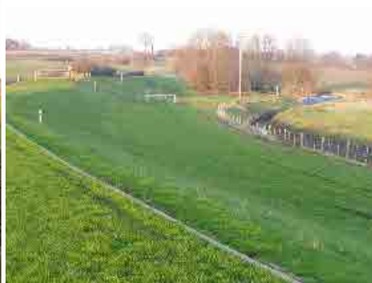
Main evacuation channel to 'throttle' – note large over-spill weir, top right, on photo on right (over-spill from main channel into flood storage area)
