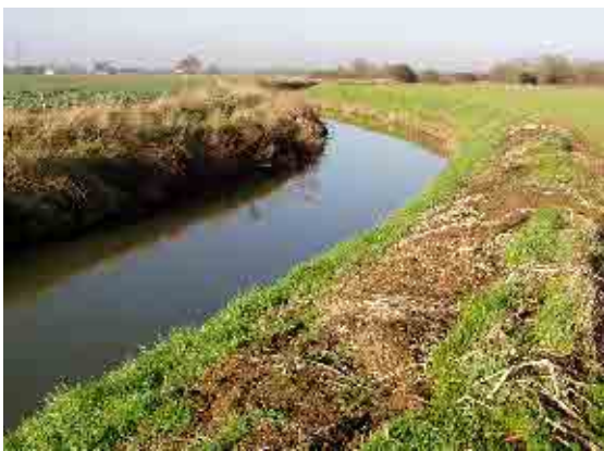
Typical dredged section – no toe left, and predominance of gravel and pebbles in dredgings
