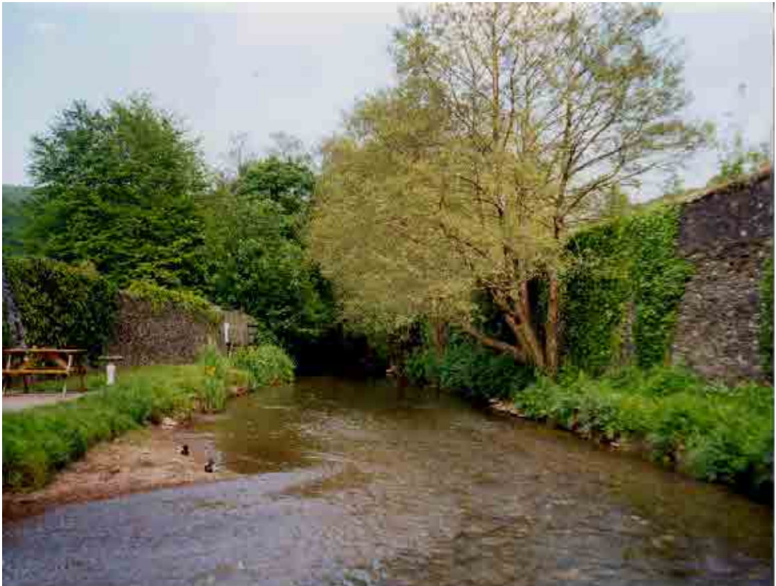
Photo 1: View of river before works
