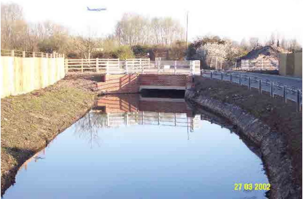
Leylands Lane culvert and new channel
