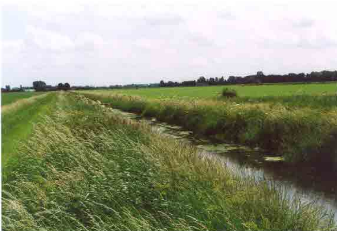
Plate 2 Gravel Drain, Welland and Deeping IDB Area, South Lincolnshire.
