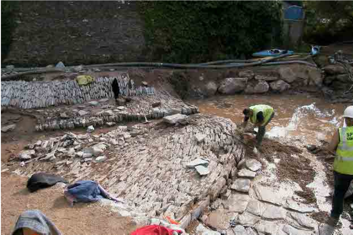
Photo 2: Village green riffle under construction
