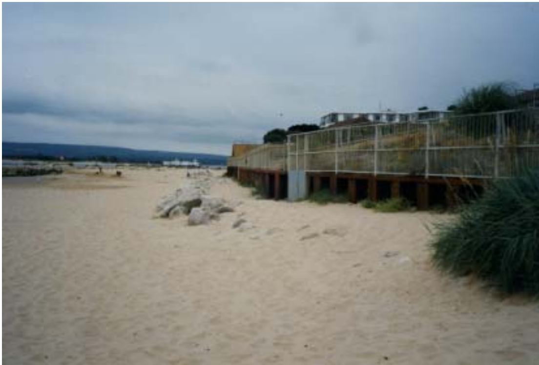
Widened beach after installation of sill and rock groynes, Sandbanks (2002)
