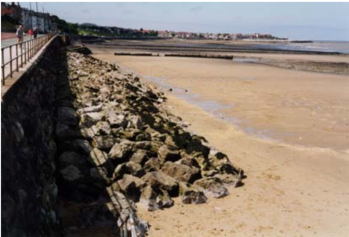
Rock berm in front of vertical seawall, Colwyn Bay
