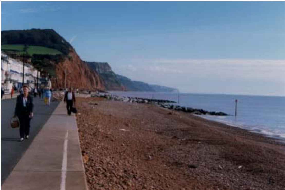
Rock groynes and beach recharge, eastern end of promenade, Sidmouth
