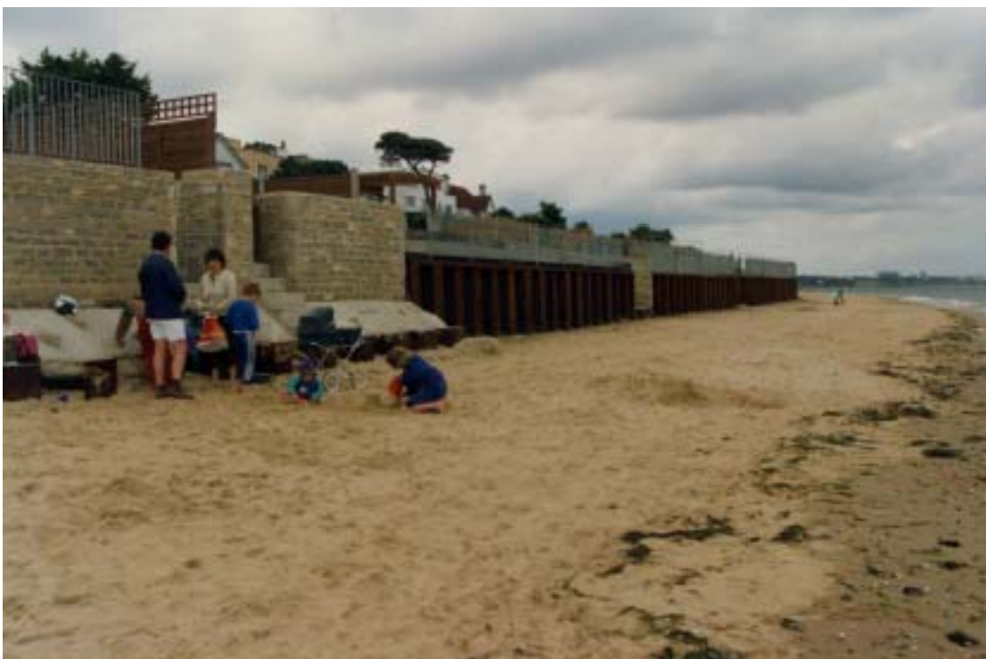
Vertical wall and low beach near Haven Hotel, Sandbanks (c1998)
