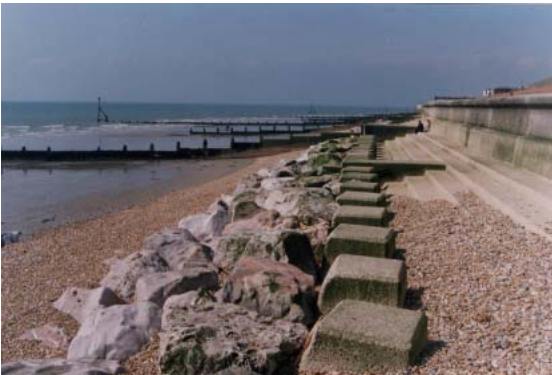
Toe berm of rock and concrete armour units, Selsey Bill (1994)
