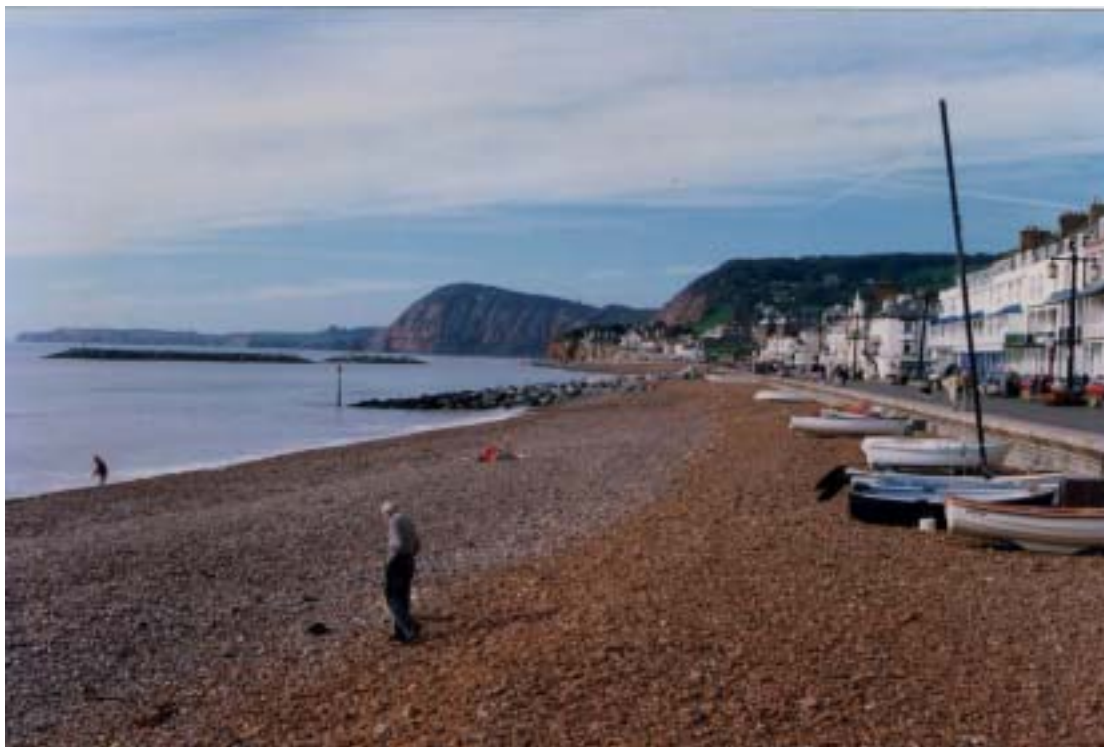
Beach recharge, groyne and offshore breakwaters, Sidmouth
