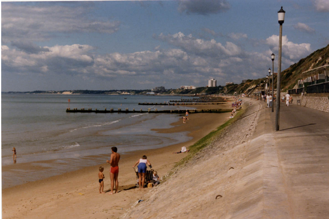
Plate 9 Seawall preventing sand supply from cliffs, Bournemouth
