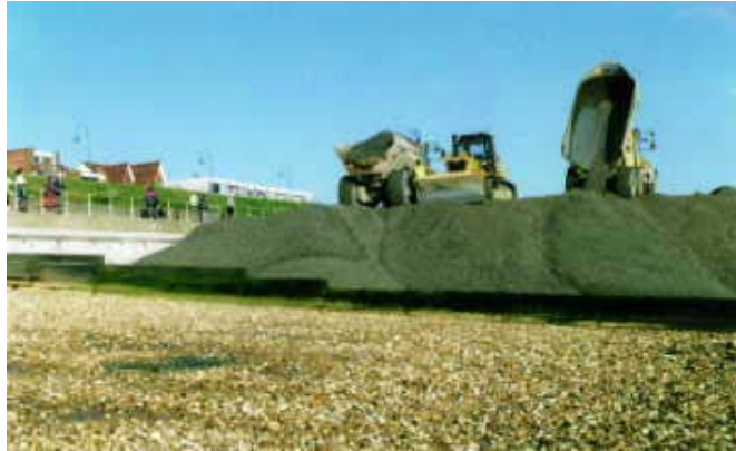
Figure 5.7 Beach recharge at Lee-on-the-Solent 1997 (from Kemp, 1999)
