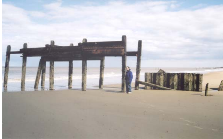
Figure 5.13 Remains of groynes at Happisburgh
