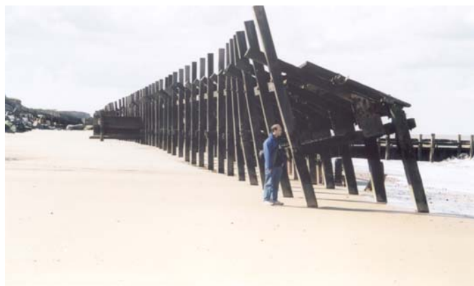
Figure 5.12 Timber revetments at Happisburgh
