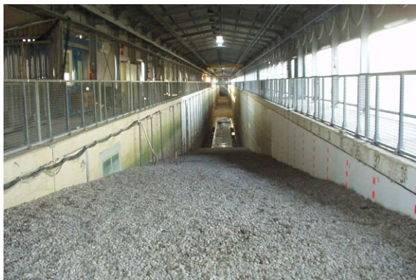
a) Installed Gravel Beach
