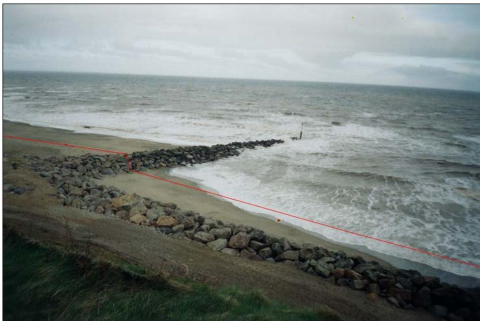
**Figure 18 Permeable Rock groyne at Mappleton**
