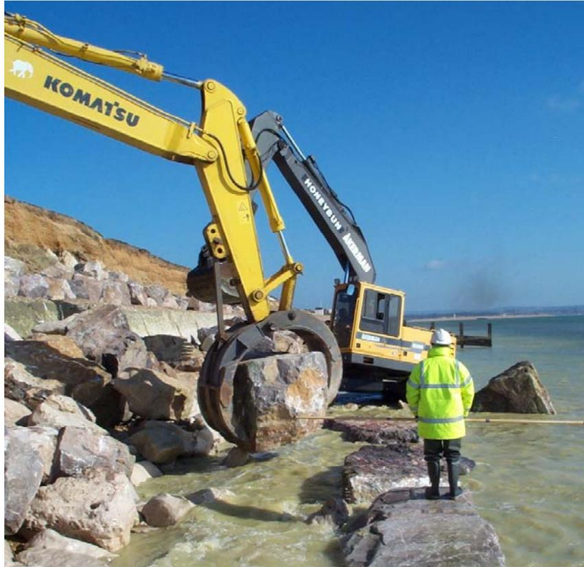
**Construction continuing on a rising tide following placement of the ‘toe stones’**
