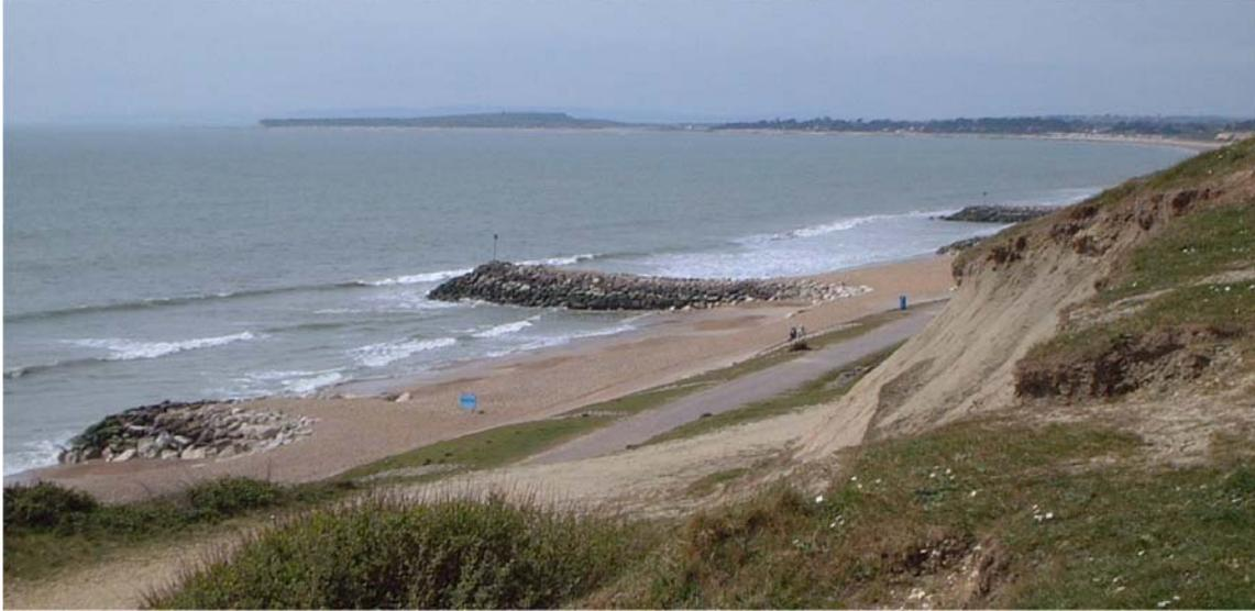
Rock groynes were constructed in 1992 to replace life-expired timber groynes at the base of an unconsolidated sandy clay cliff in Christchurch Bay, on top of which Highcliffe Castle is located. In order to minimise the cost of the works whilst maintaining the existing groyne positions and spacing, alternating long (80m) and short (60m) rock groynes were used to retain the required width of shingle beach.
