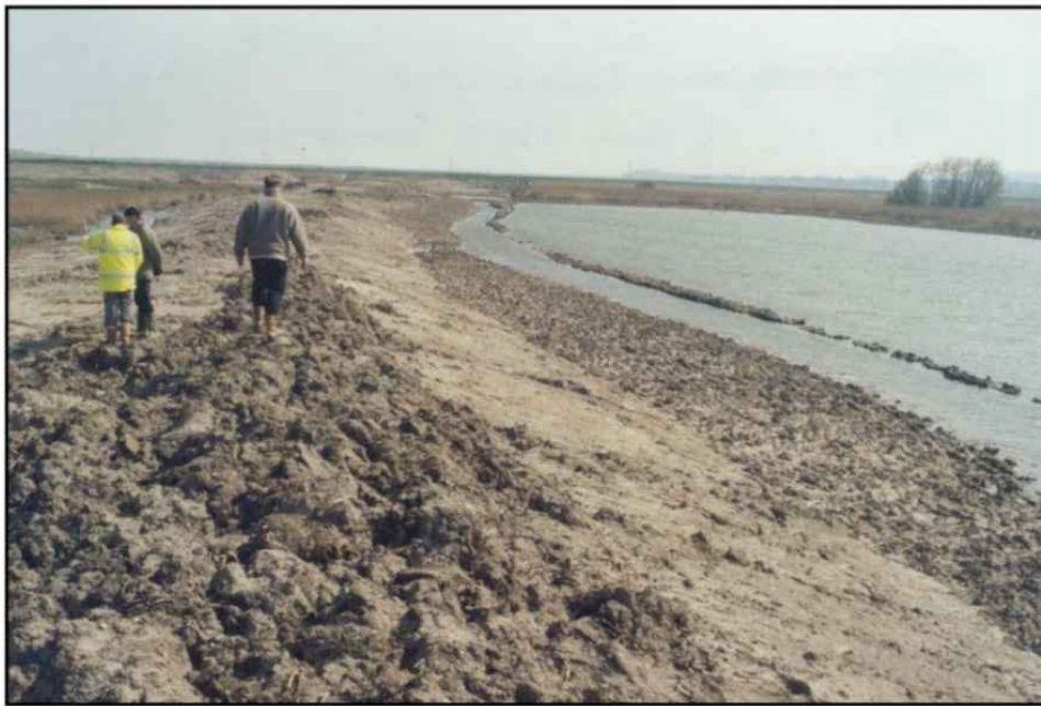
Construction of New Counter Wall (East Side of Retreat Site)
