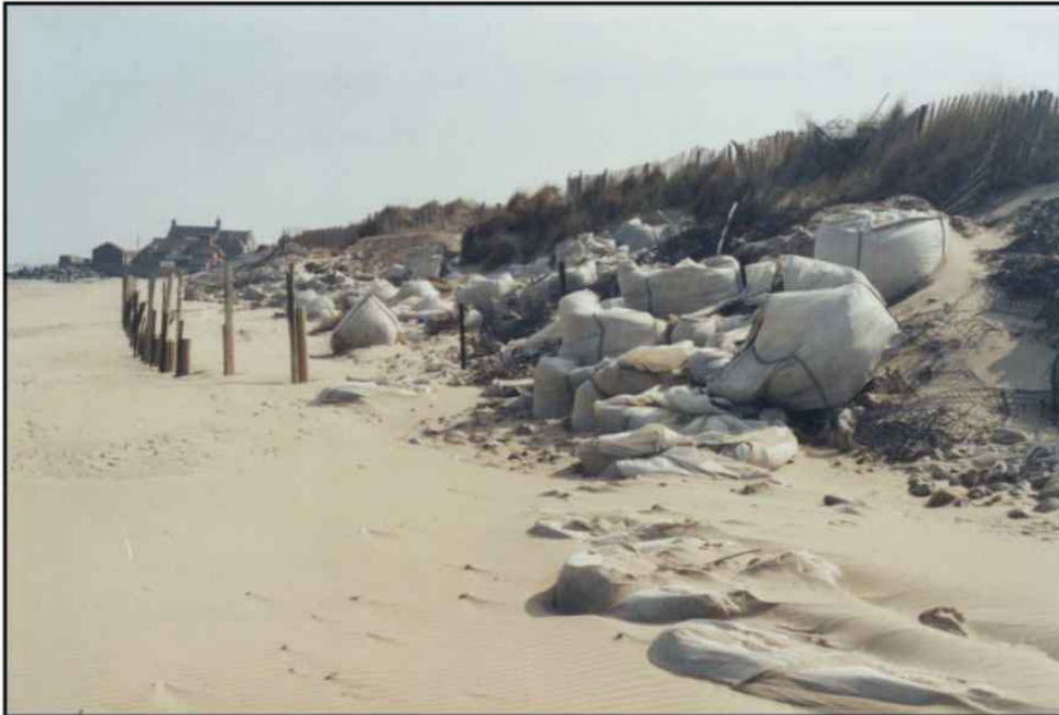
Existing Coastal Defences (North Side of Retreat Site)
