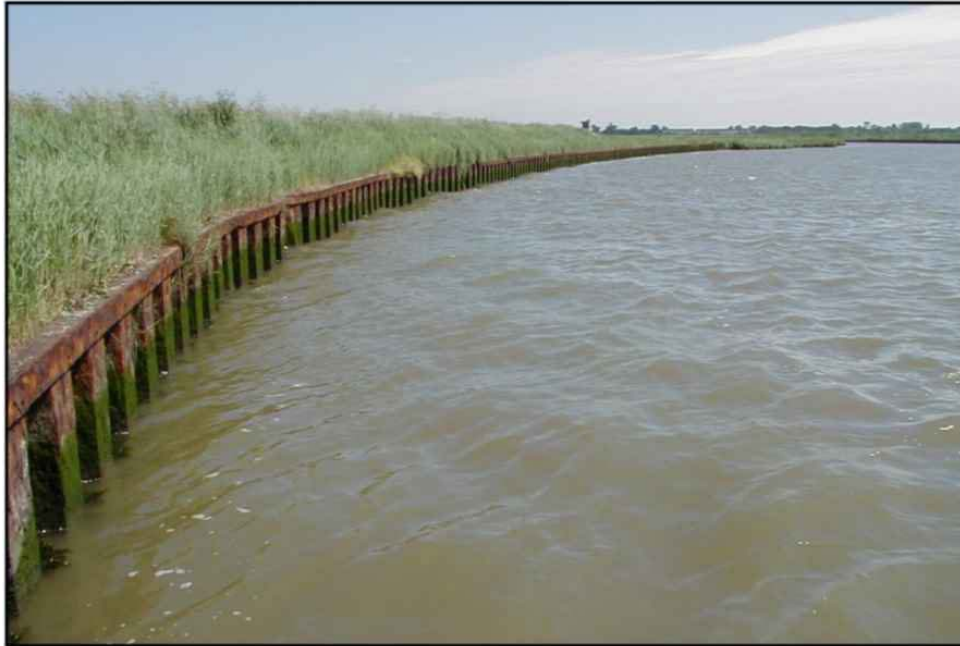
Piling, 7 mile reach
