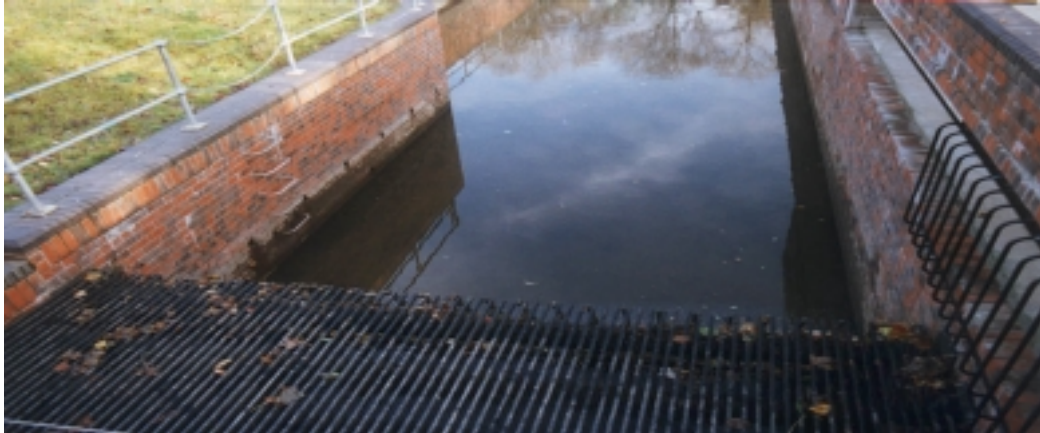
Figure 3.4 View immediately upstream of the screen showing the levels of each bank top. On the right, the position of the overflow dictates the height of the hardstanding area where debris has to be collected.
