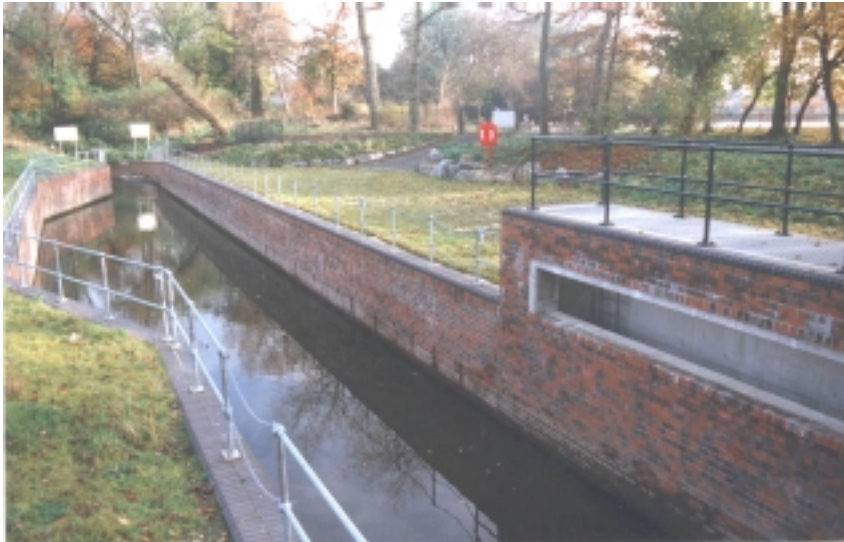
Figure 1.1 General view of Platt Fields trash screen site looking upstream showing silt trap, hard standing and emergency overflow weir. Note that the weir and hard standing are at coincident levels.
