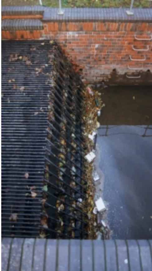
Figure 5.1 Leaf debris is clearly visible at the bottom of the screen that should be passed through the screen. Operatives have stated that during an event the majority of their time is spent clearing leaves.
