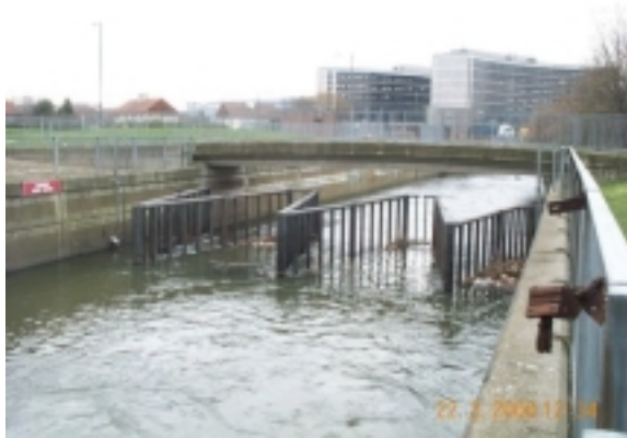
Figure 2.2 View looking downstream showing the labyrinth structure under moderate flow conditions
