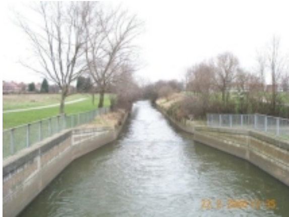
Figure 2.4.1 View looking upstream clearly showing the local channel widening at the silt trap, under moderate flow conditions.
