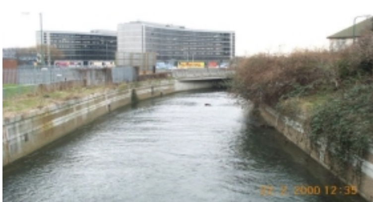
Figure 1.3 View downstream of the screen showing the culvert entry under the North Circular
