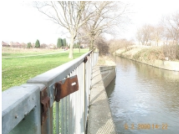
Figure 2.6 The park area to the left of the fence is designed to be used as a flood storage area.
