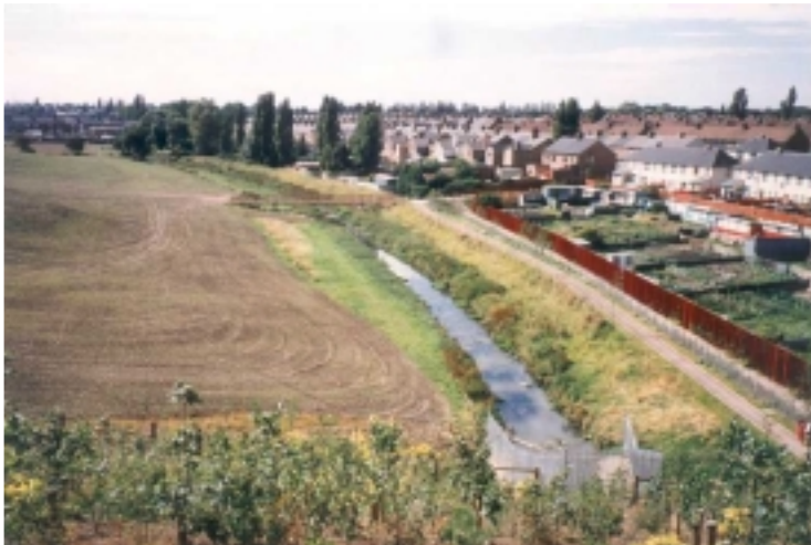
Figure 1.1 View of the area prior to construction of the screen but after the installation of the culvert.
