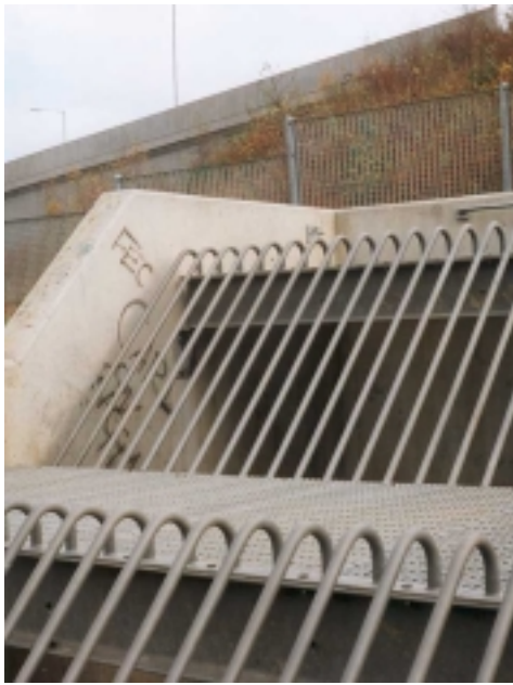
Figure 3.3 View on top screen, the angle of rake and construction details are clearly visible.
