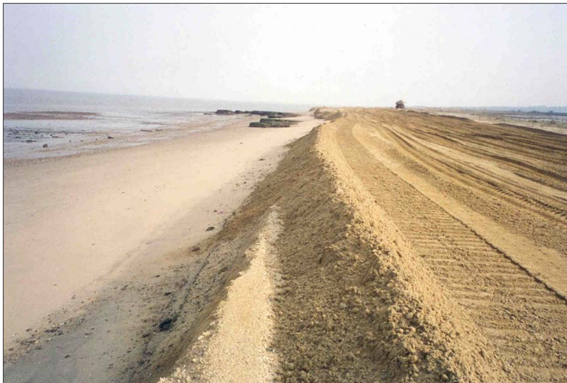
Plate 4.31 Creation of an artificial 'washover dune' using sand dredged from Harwich Harbour, entrance to Walton Backwaters.
