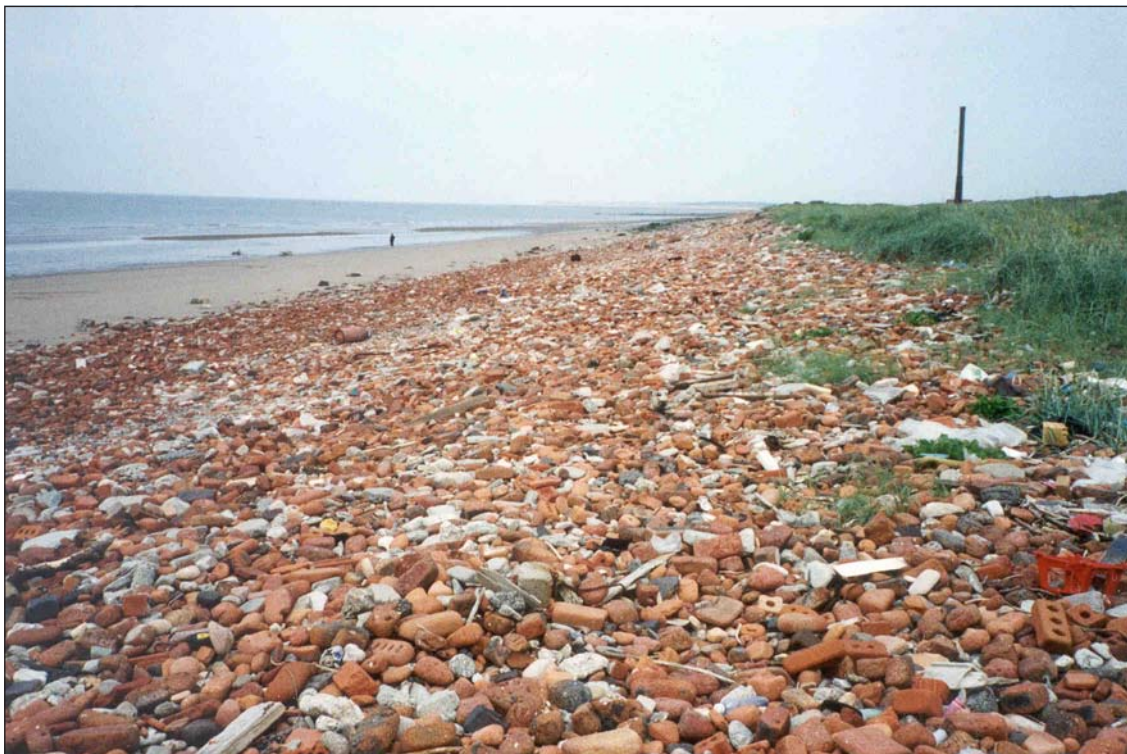
Plate 4.8 Dune frontage protected by an artificial beach composed of bricks and lumps of concrete from the demolition of Fort Crosby, between Hightown and Blundellsands, Sefton Coast.
