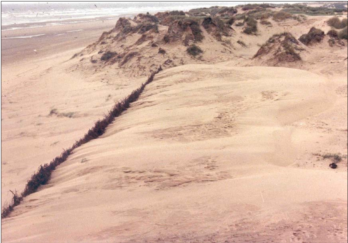
Plate 4.22 Brushwood fence erected across the mouth of a large blowout to trap sand on the leeward side, Formby Point, Sefton Coast.
