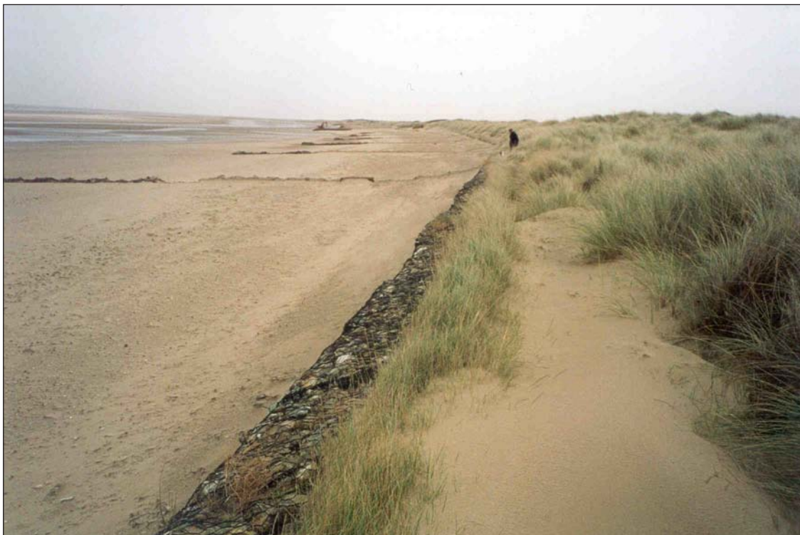
Plate 4.6 Dune frontage protected by rock-filled gabions and low groynes, Old Hunstanton, North Norfolk.
