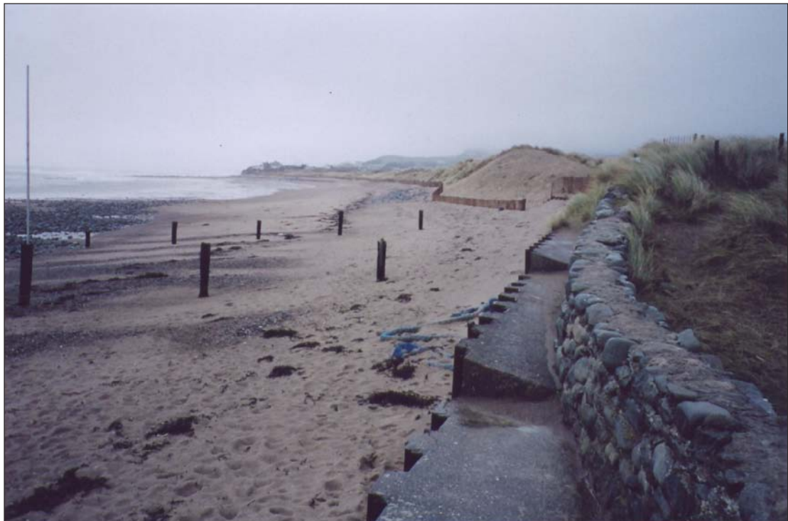
Plate 4.2 Dune toe protected by steel pilings, concrete, and masonry wall, south end of Llandanwg frontage, Wales.
