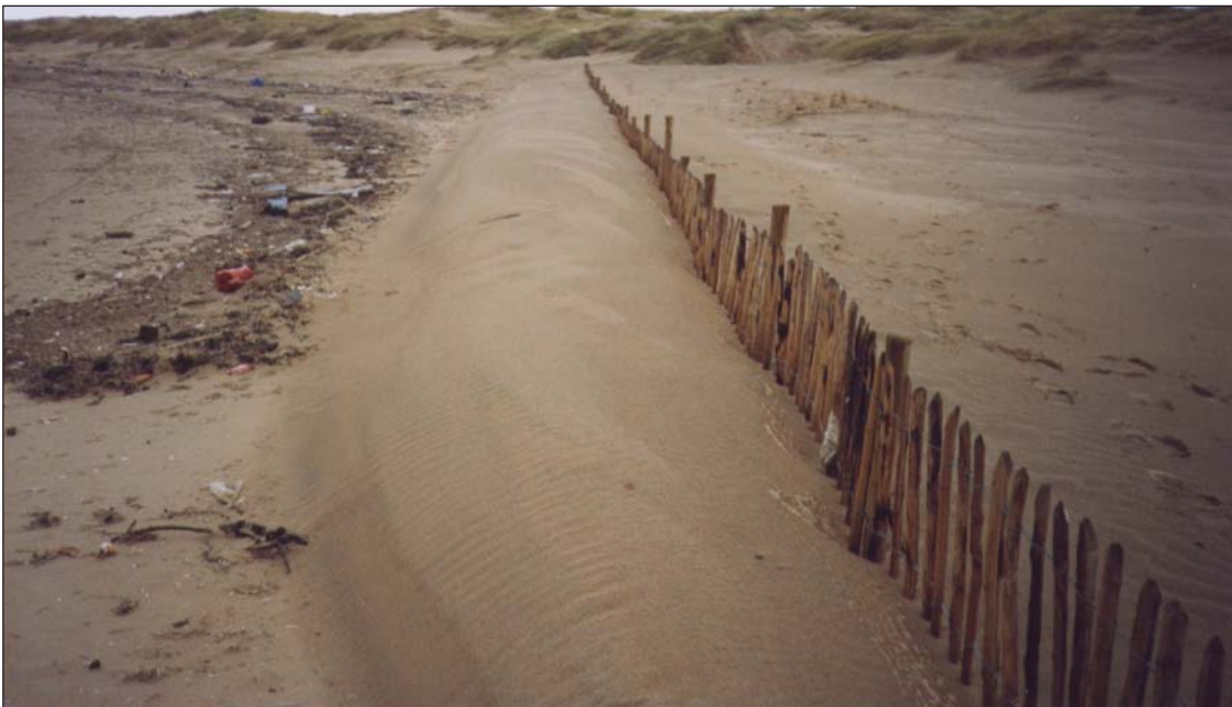
Plate 4.14 Single line of chestnut plating fencing placed obliquely on the upper beach to trap sand and with the intention of creating a wet slack behind, Cabin Hill National Nature Reserve frontage, Sefton Coast.
