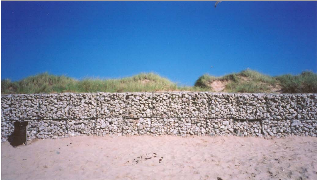
Plate 4.5 Dune frontage protected by cobble-filled gabions, Fistral Bay Cornwall.
