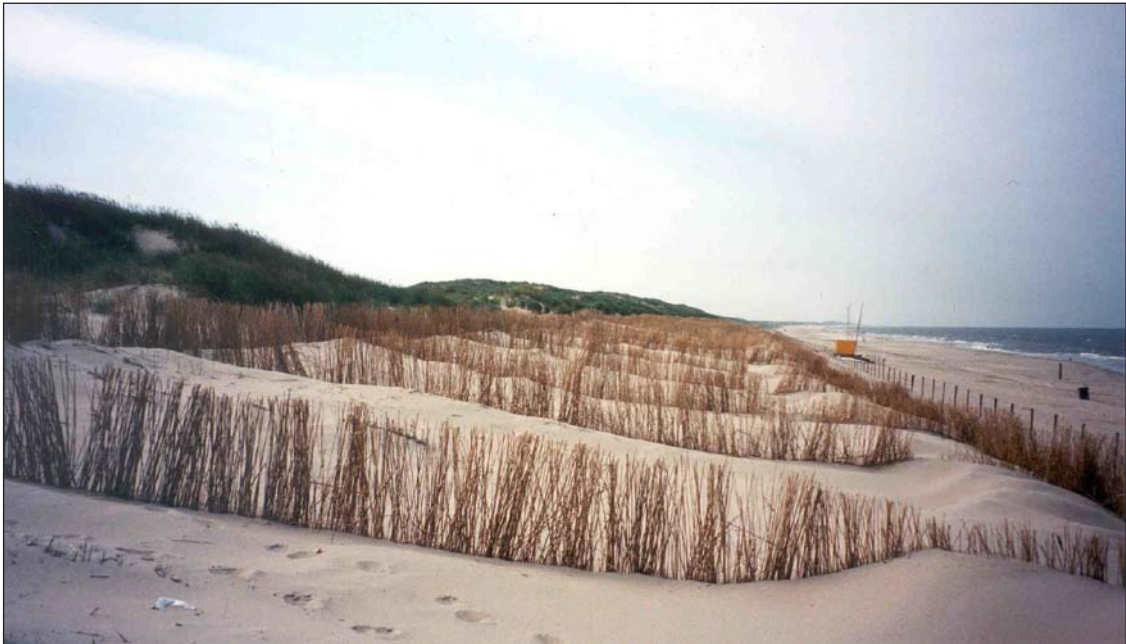
Plate 4.13 Wattle fencing placed both parallel and perpendicular to the beach and frontal dune toe in order to increase the width of the frontal dune, Texel, The Netherlands.
