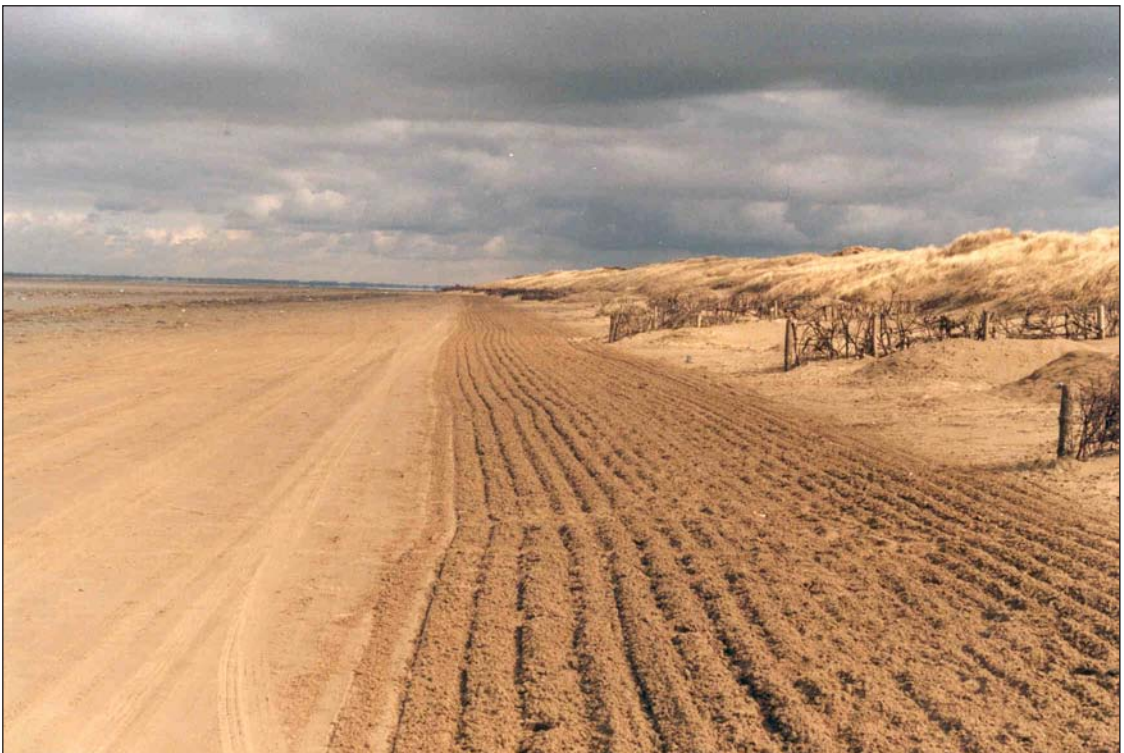
Plate 4.16 Timber posts and brushwood fencing constructed transverse to the dune front in order to trap sand blown along the beach. Ploughing of the upper beach in this instance was undertaken primarily for racecourse training but also has the effect of enhancing aeolian transport to the dunes, Ainsdale, Sefton Coast.
