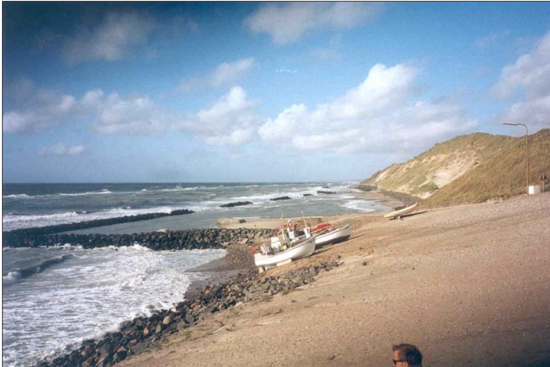
Plate 4.9 Eroding dunes protected by an artificial rocky beach and offshore rock reefs, near Løkken, Denmark.
