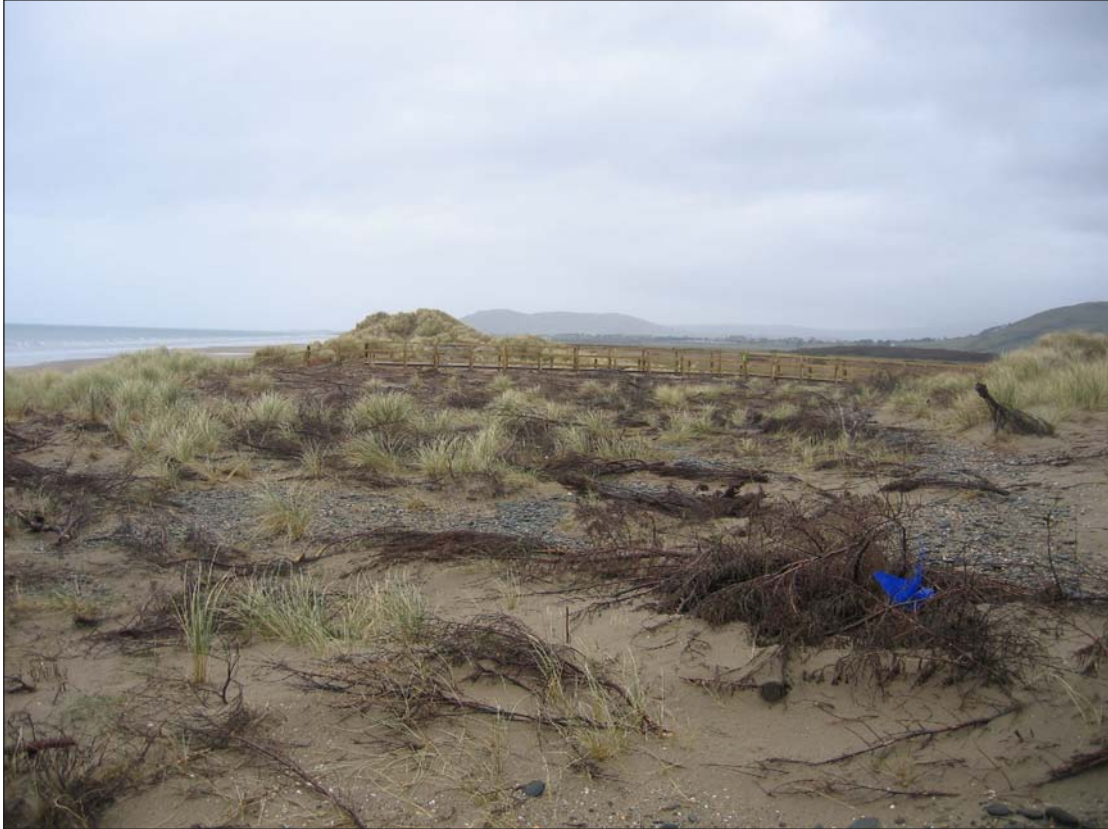
Plate 4.28 A recharged area of the frontal dunes north of Aberdovey, west Wales. Wind-deflation of the deposited sand is limited by emplacement of brushwood and gravel which is naturally present in the harbour dredgings.
