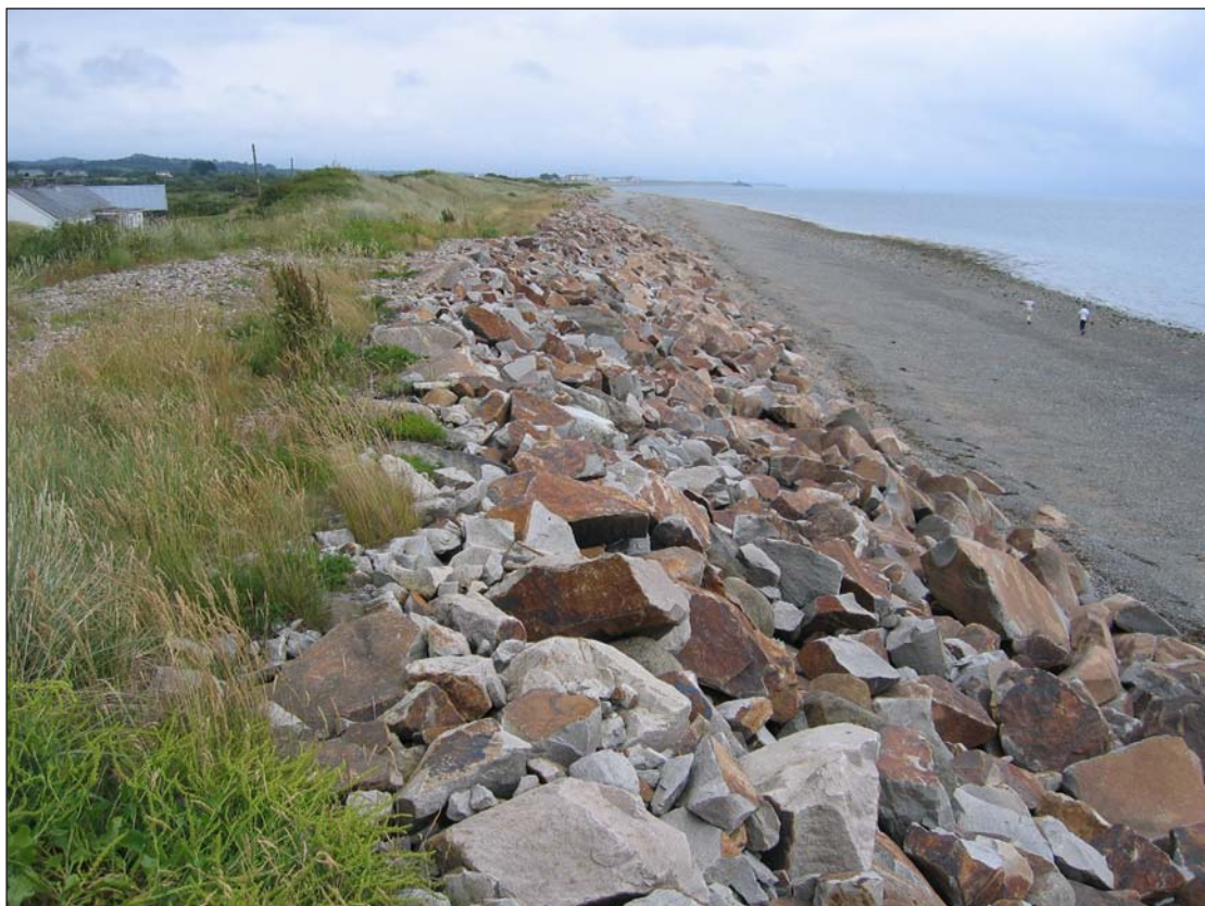
Plate 4.4 Narrow frontal dune ridge protected by rock armour, Traeth Crugan, Wales. Pwllheli golf club to the left of the picture.
