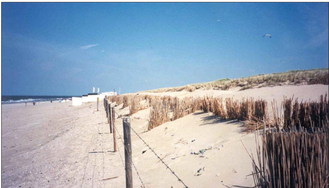
Plate 4.12 Barbed wire fencing and planted rows of wattle fencing designed to trap sand on the seaward side of the foredune ridge, Texel, The Netherlands.
