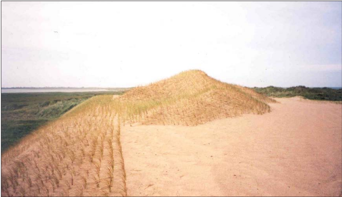
Plate 4.24 Artificially re-profiled dune recently planted with marram, Thy, Denmark.
