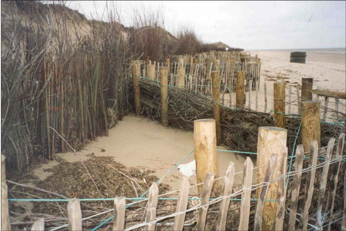
Plate 4.15 Zig-zag arrangement of timber posts, chestnut palings and placed brushwood designed to trap sand transported to the upper beach both by wave action and aeolian processes, Brancaster Bay, north Norfolk.
