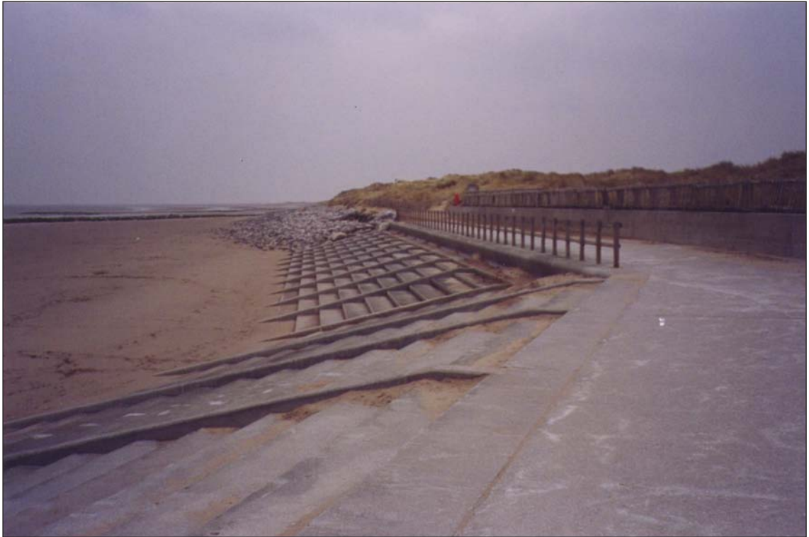
Plate 4.1 Example of a dune frontage protected by a concrete sea wall and (in the distance) rock armour: east of Prestatyn, North Wales.
