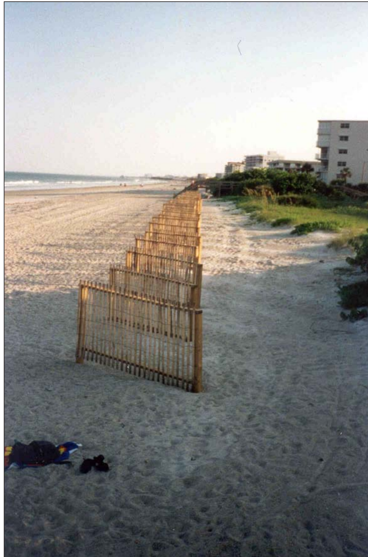
Plate 4.17 Short lengths of wooden fencing placed in a line on the upper beach oblique to the dune toe but transverse to the dominant sand transport. Cocoa Beach, Florida.
