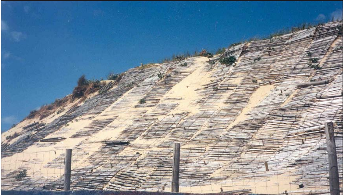
Plate 4.19 Wooden slats placed on the seaward face of an eroding dune to reduce sand loss by wind deflation, Cap Feret, southwest France.
