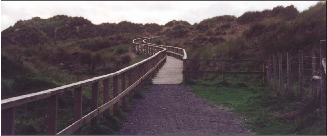
Plate 4.26 Boardwalk constructed to control access through the dunes to the beach, Morfa Dyffryn, west Wales.
