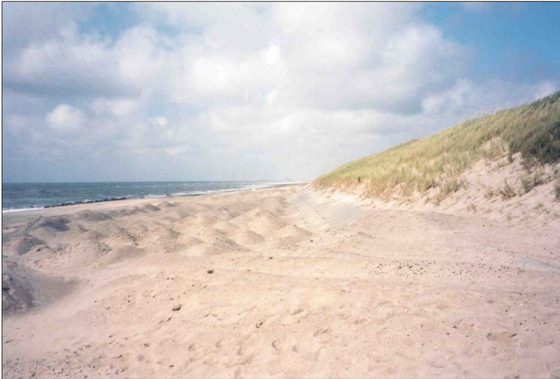
Plate 4.30 Artificial piles of sand placed on the backshore to nourish the dunes behind, Bjerghuse, western Denmark.
