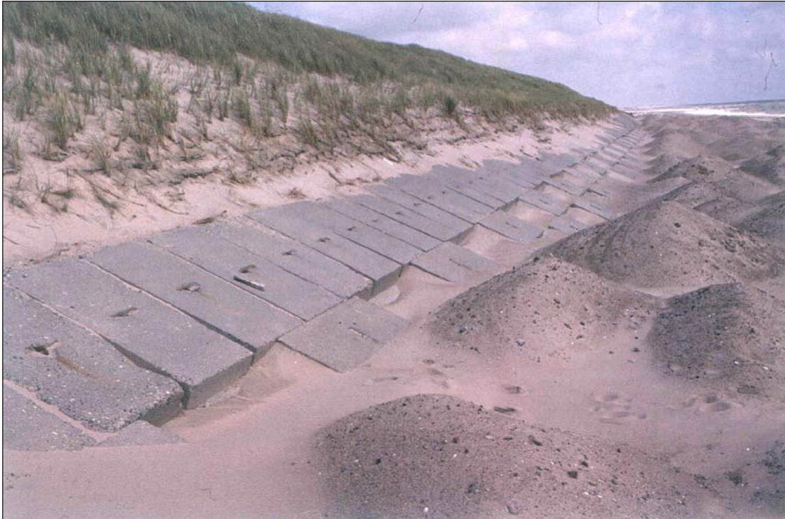
Plate 4.3 Dune toe protected by placed concrete blocks. Note piles of 'placed' beach nourishment material designed to trickle-feed the frontal dunes with wind blown sand. The seaward face of the foredune ramp has been covered with a coarse-mesh geotextile and planted with marram. West coast of Jutland, Denmark.
