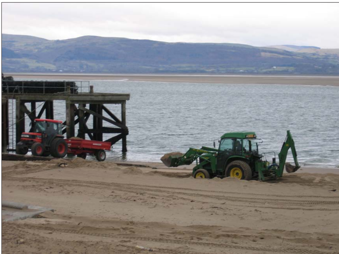
Plate 4.27 Removal of sand from the Aberdovey harbour area for recharge of the frontal dunes along the Aberdovey to Tywyn frontage, west Wales.
