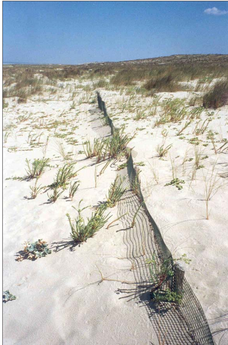
Plate 4.21 Single row of plastic mesh fencing placed to control the rate of movement of bare sand, Cap Feret, southwest France.
