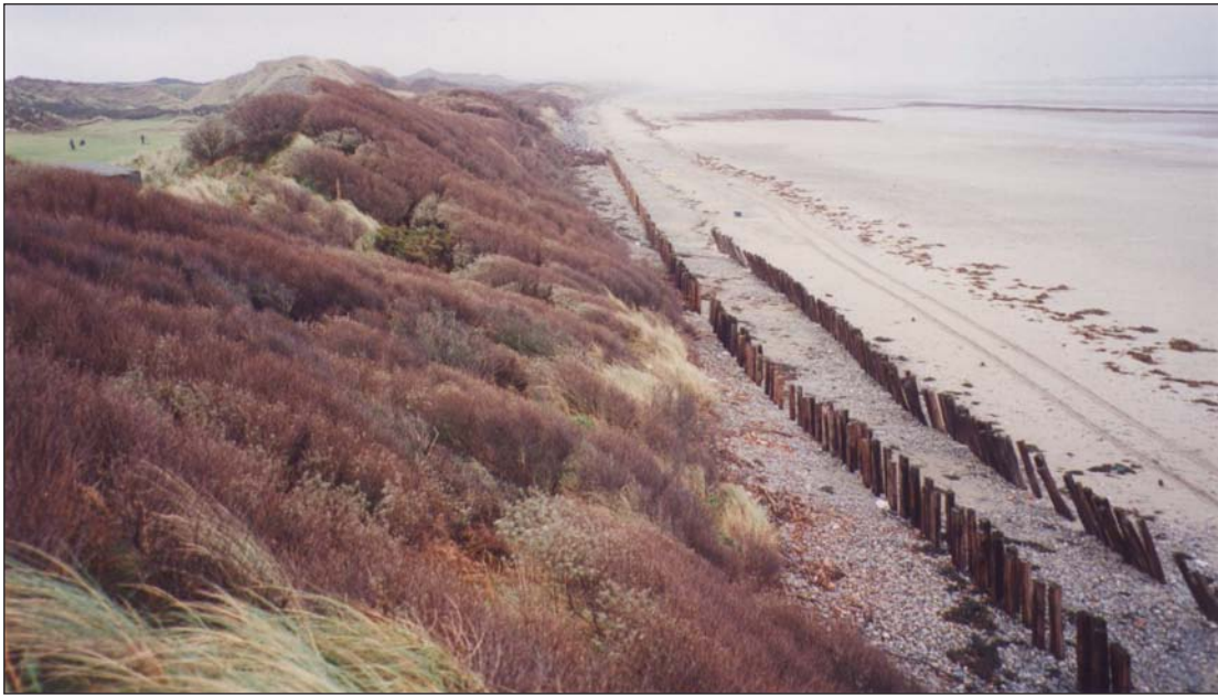
Plate 4.7 Dune frontage protected by a wooden revetment constructed of old railway sleepers, Dundrum Bay, Northern Ireland. Royal County Down Golf Club to the left of the picture.
