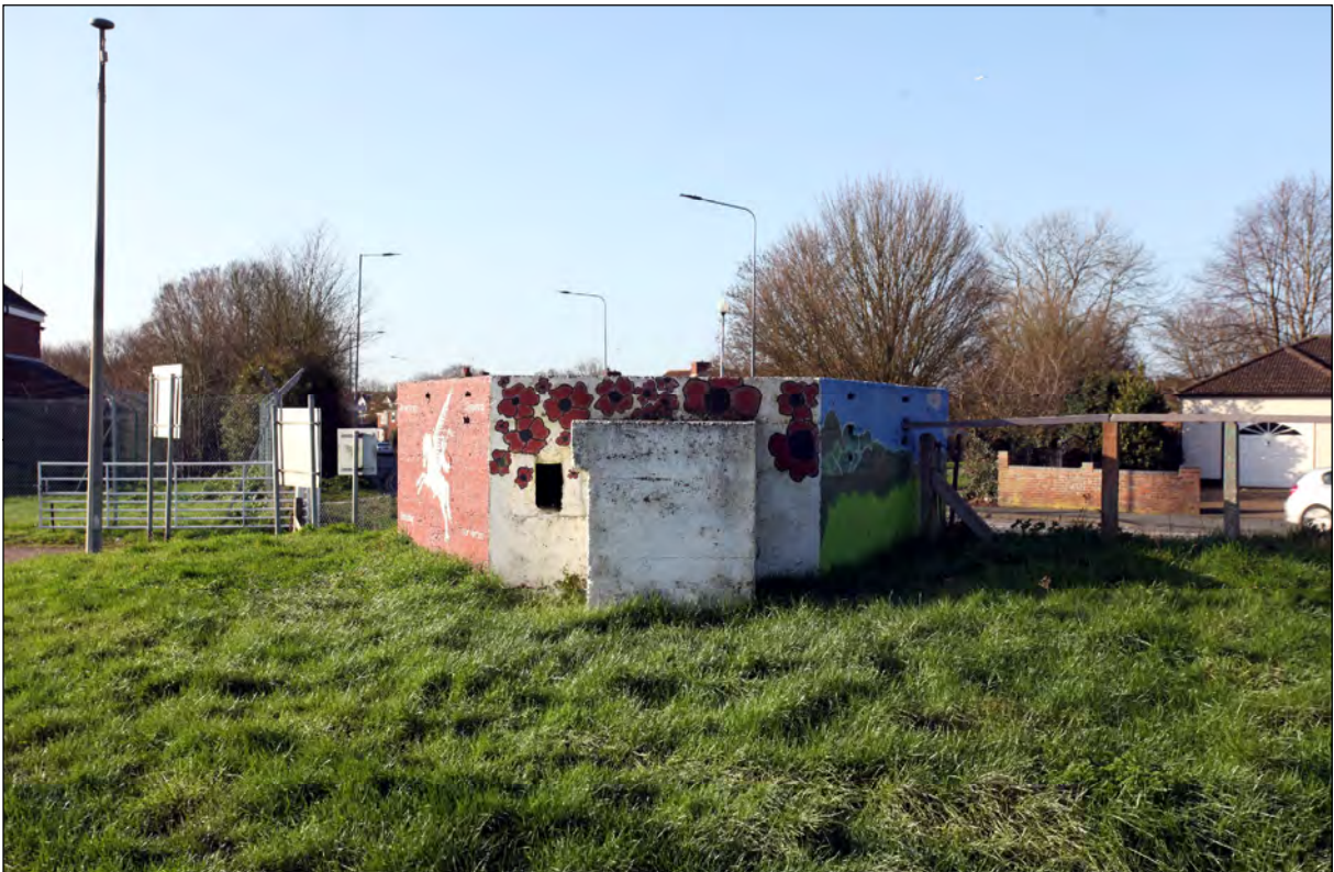
Plate 23) Pillbox (MCC5357) at western boundary of the Site
