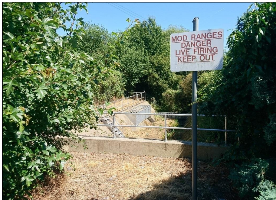
Figure 5.1 Anglian Water outfall compound adjacent to Mersea Road (image taken June 2018)
