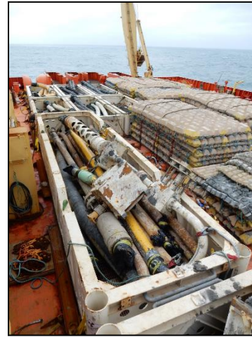
Infield Jumpers and Flowlines Recovered
