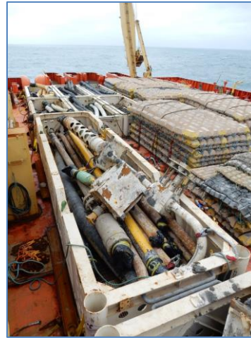
Infield Jumpers and Flowlines Recovered
