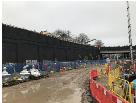
Park Village East retaining wall
