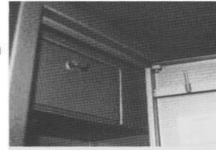
Any internal compartments for the storing of ammunition rifle bolts, etc. should be as strong as the main body of the cabinet
