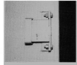
Fastenings must be appropriate to the size and structure. 'Rawl' and expanding bolts should be utilised in stone, brick and concrete. Coach screws and bolts for timber joists. The cabinet manufacturers will usually include recommendations for fixing devices
