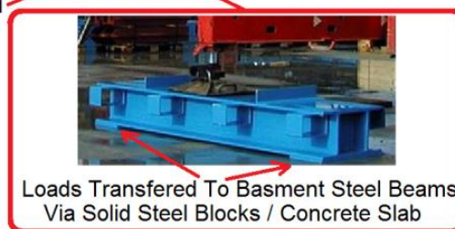
Temporary Outrigger Steel For Mobile Crane
