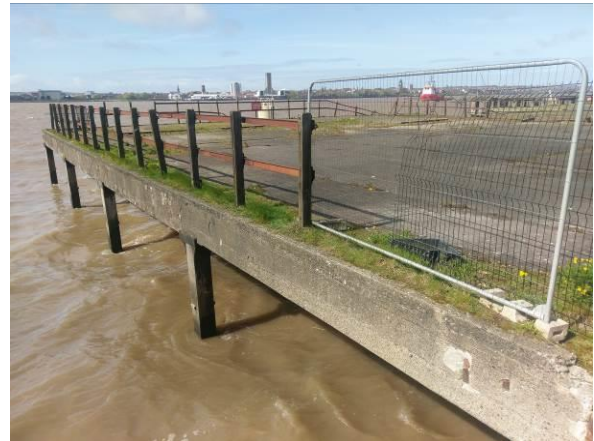
Plate 4: Large concrete topped jetty
