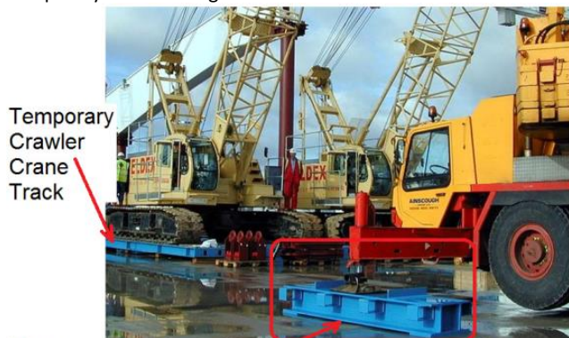
Temporary Outrigger Steel For Mobile Crane
