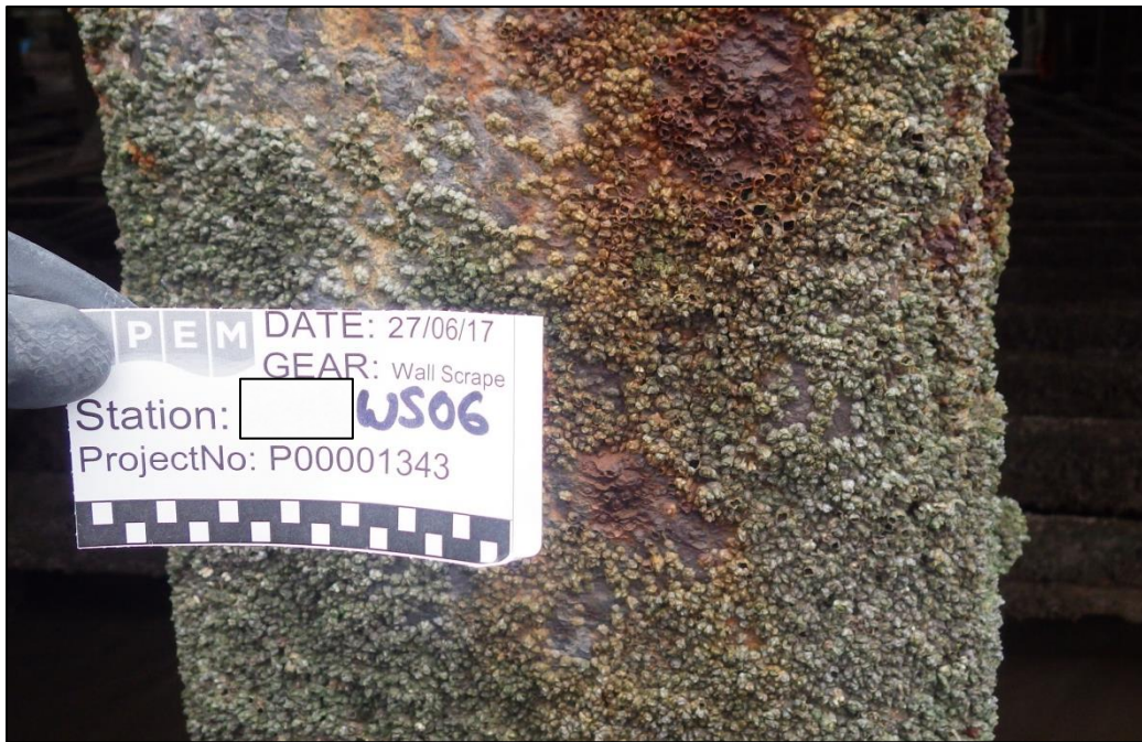
Figure 10: Metal pontoon leg at Station WS06 with encrusting A. modestus .
