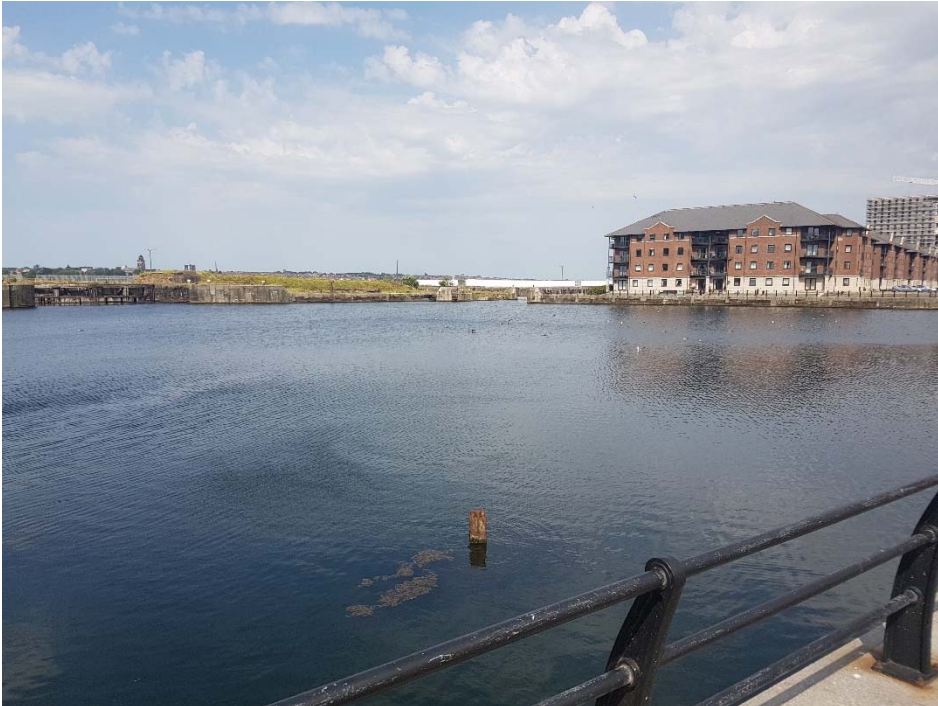
Photo 1 – Princes Half-Tide Dock site
