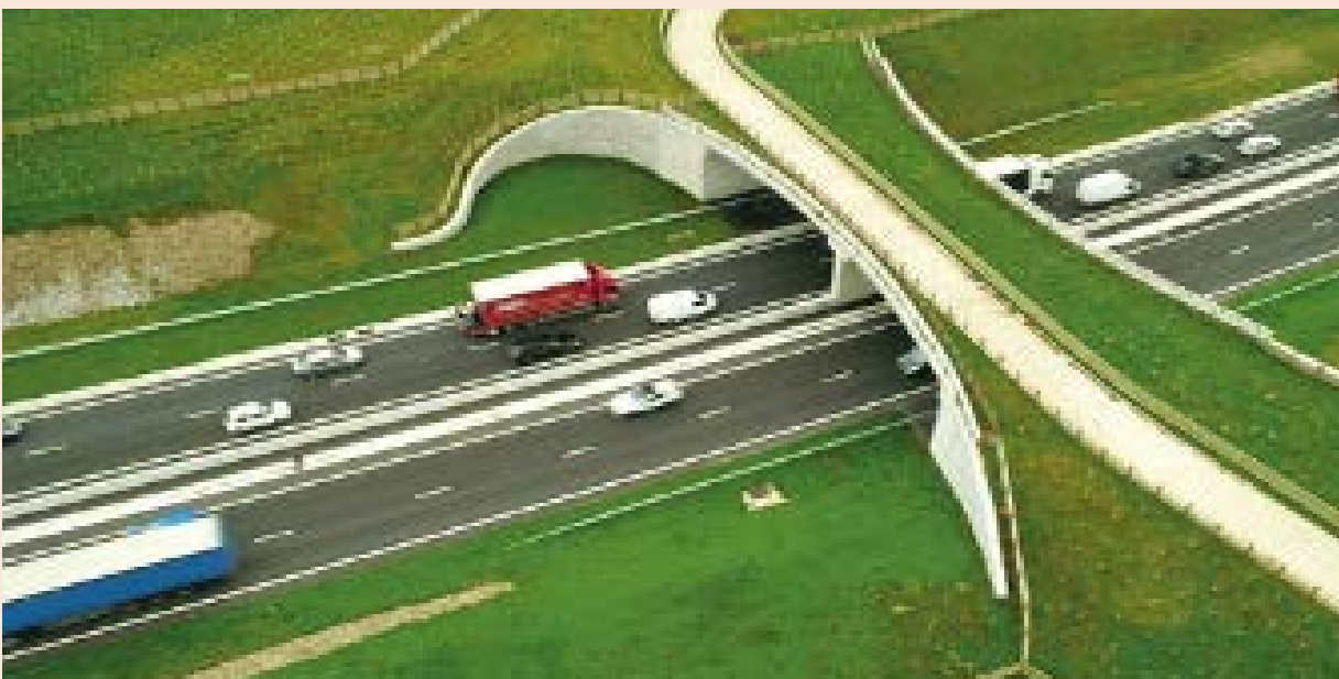
A green bridge over the A556 constructed during RP1
