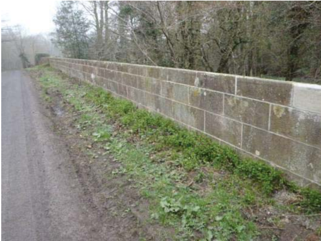
Photo No.4: East roadside parapet: Pointing repairs.
