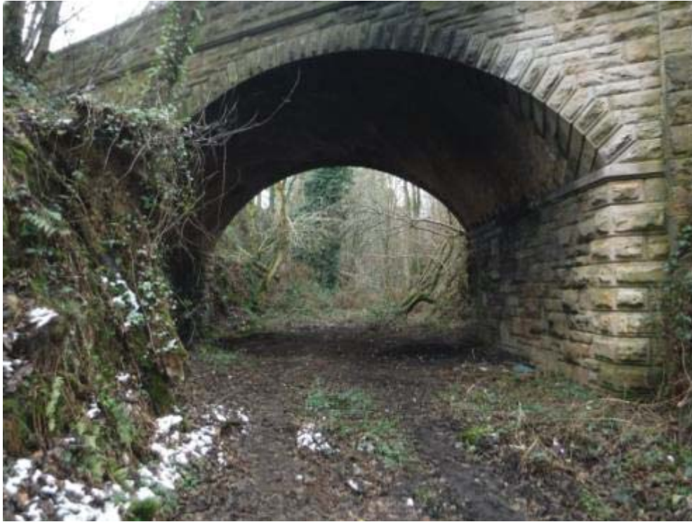
Photo No: 9 – Area under the structure: Typical example.
