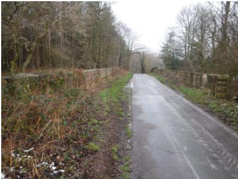
Photo No: 10 – View: Across the structure looking north.
