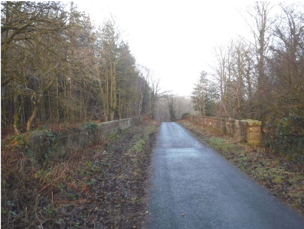
Photo No.7: View: Across Structure.
