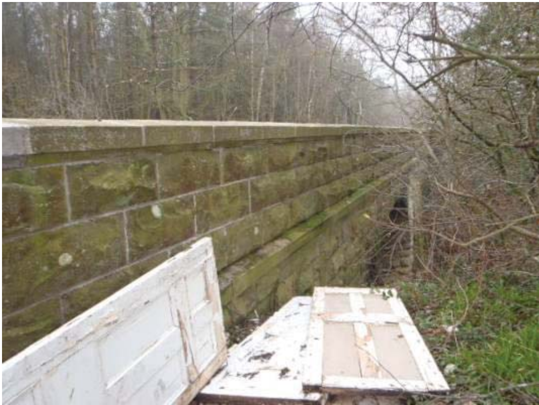
Photo No.6: East outer parapet: Pointing repairs.
