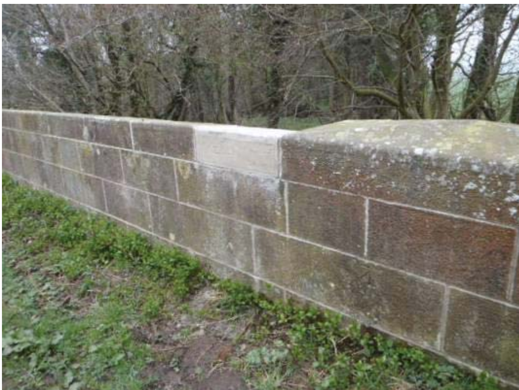
Photo No.6: East outer parapet: Pointing repairs.
