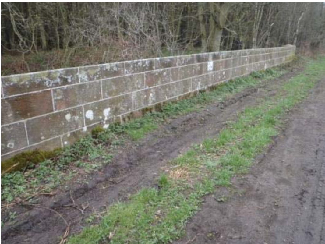
Photo No.5: West roadside parapet: Pointing repairs.
