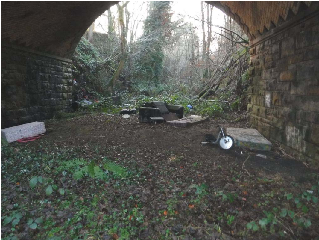
Photo No.3: Area under the structure: Typical example.
