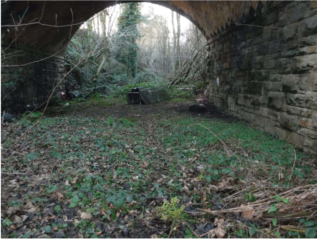
Photo No.6: Area under the structure: Typical example.
