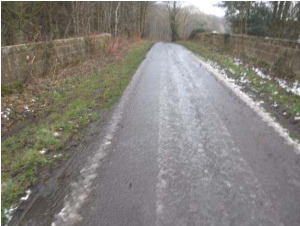
Photo No: 4 - Road surface: Typical example of the condition.
