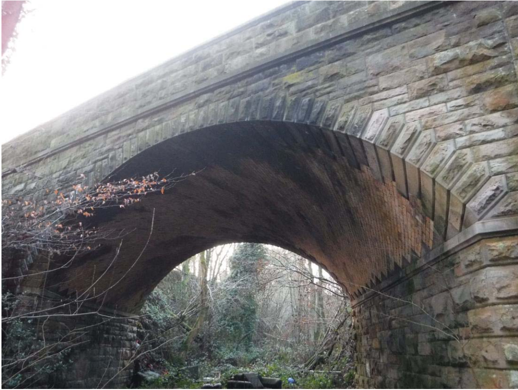
Photo No.6: Arch ring soffit: View.
