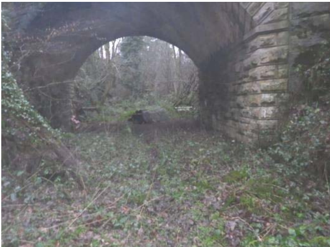
Photo No.5: Area under the structure: Typical example.
