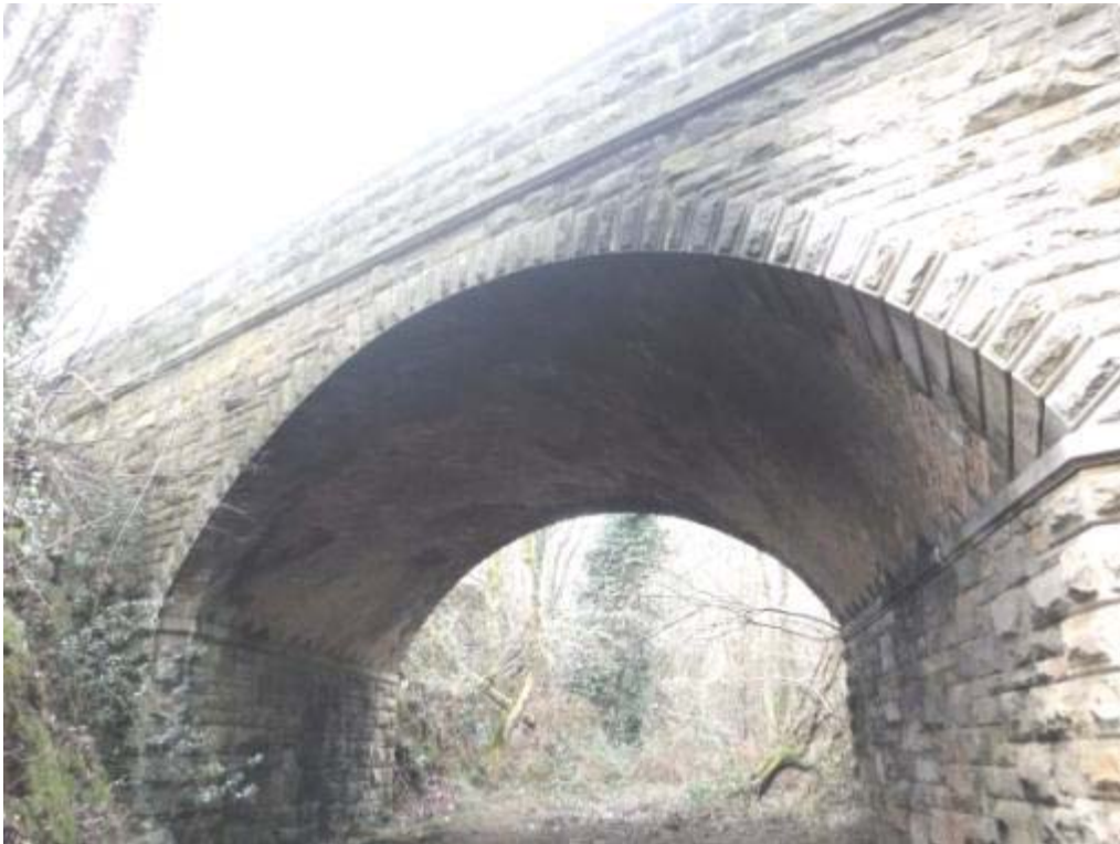
Photo No: 8 – Arch ring soffit: View.
