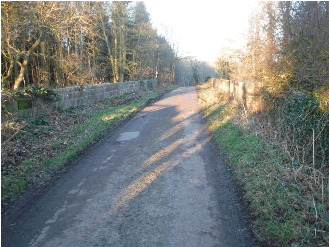
Photo No.7: View: Across Structure.
