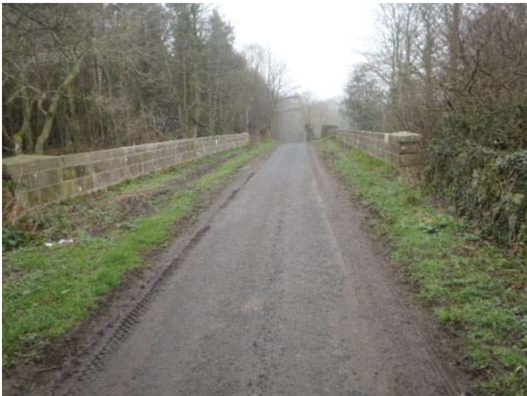
Photo No.11: View: Across Structure.
