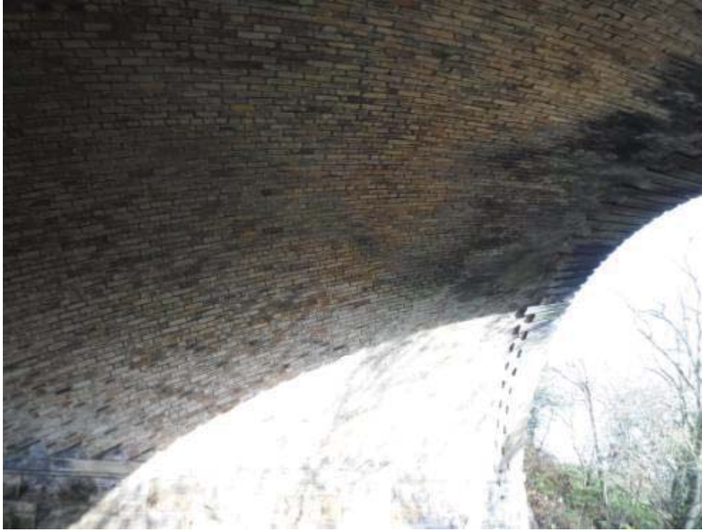
Photo No.9 - Arch ring soffit: Typical example of the condition.
