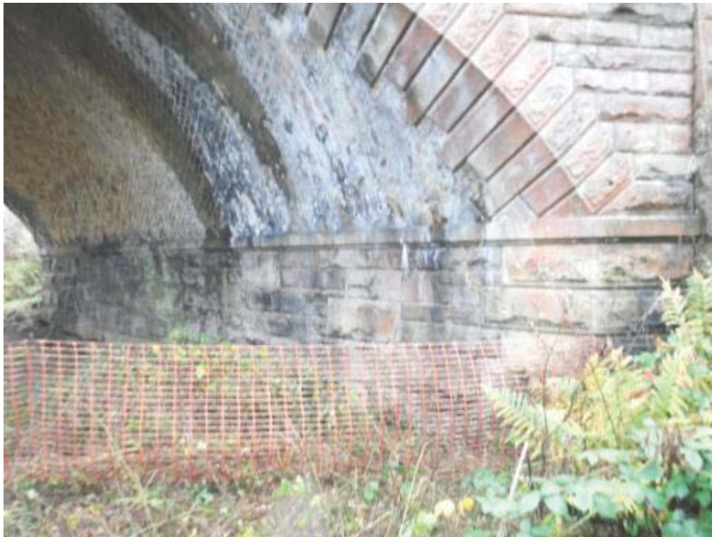
Photo No.66 - West abutment: View.
