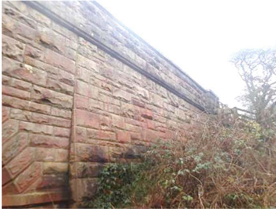
Photograph 3: general view of the northwest wingwall
