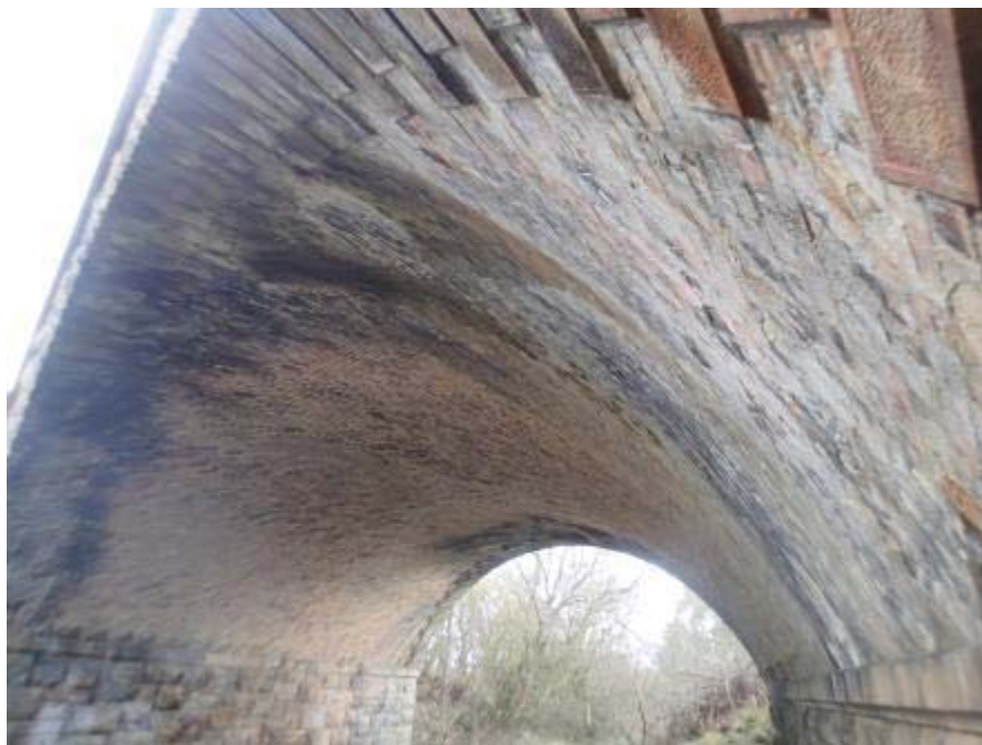
Photograph 2: general view of the soffit
