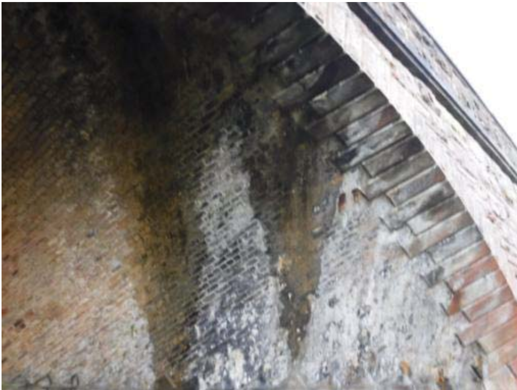
Photo No.14 - Arch ring soffit: Typical example of the condition.
