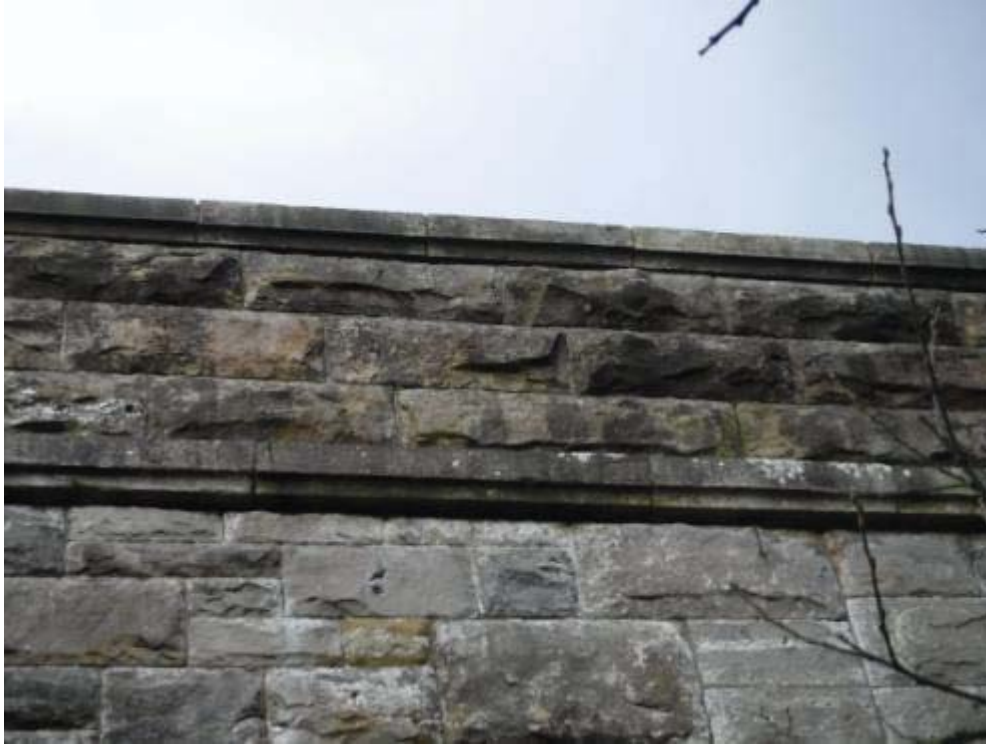
Photo No.141 - South outer parapet: Typical example of the condition.
