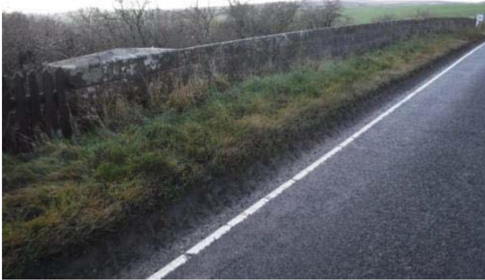
Photo No.127 - South roadside parapet: View.
