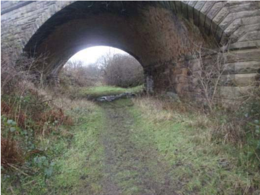
Photo No.4: Area under the structure: Typical example.
