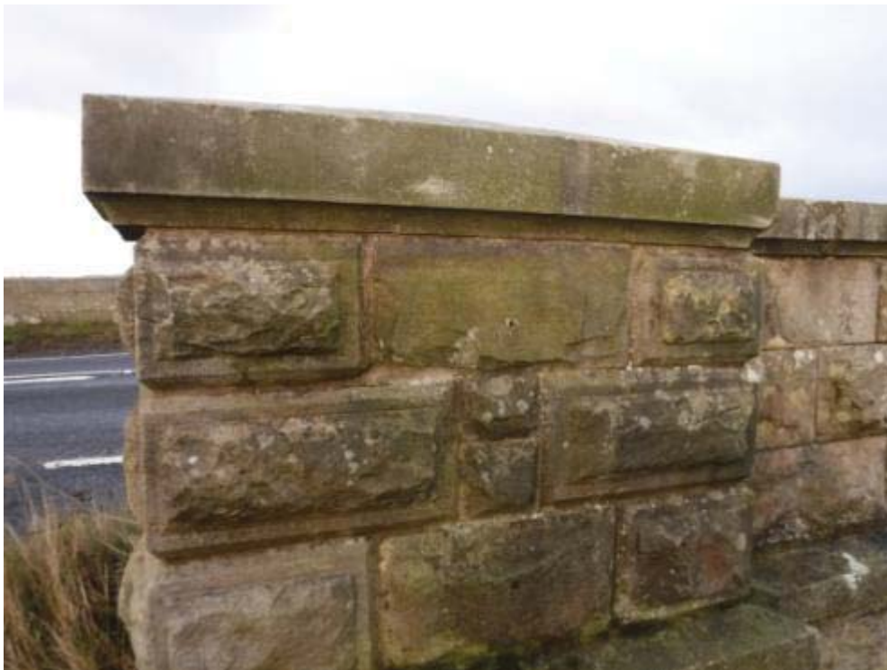
Photo No.138 - South outer parapet: S/W pilaster region rebuilt.
