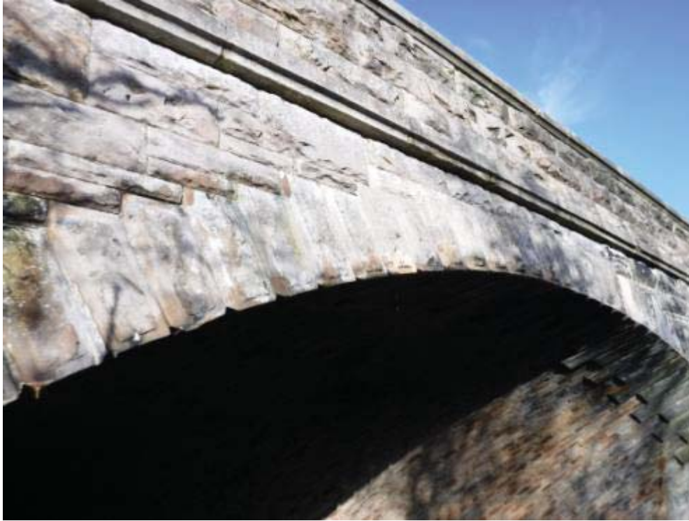
Photo No.21 - South arch ring face: Typical example of the condition.
