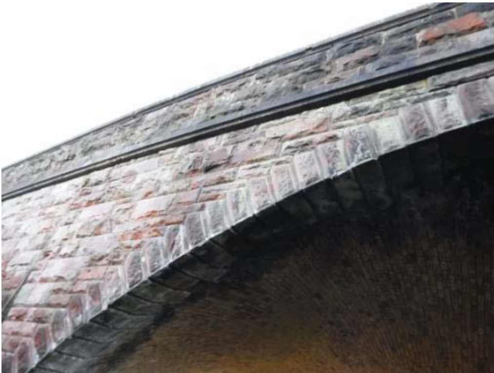
Photo No.32 - North arch ring face: Typical example of the condition.
