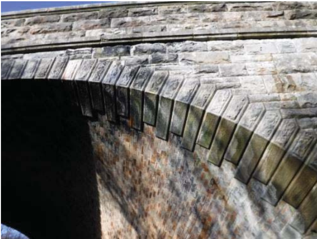
Photo No.22 - South arch ring face: Typical example of the condition.
