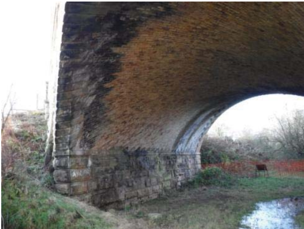
Photo No.8 - Arch ring soffit: Typical example of the condition.
