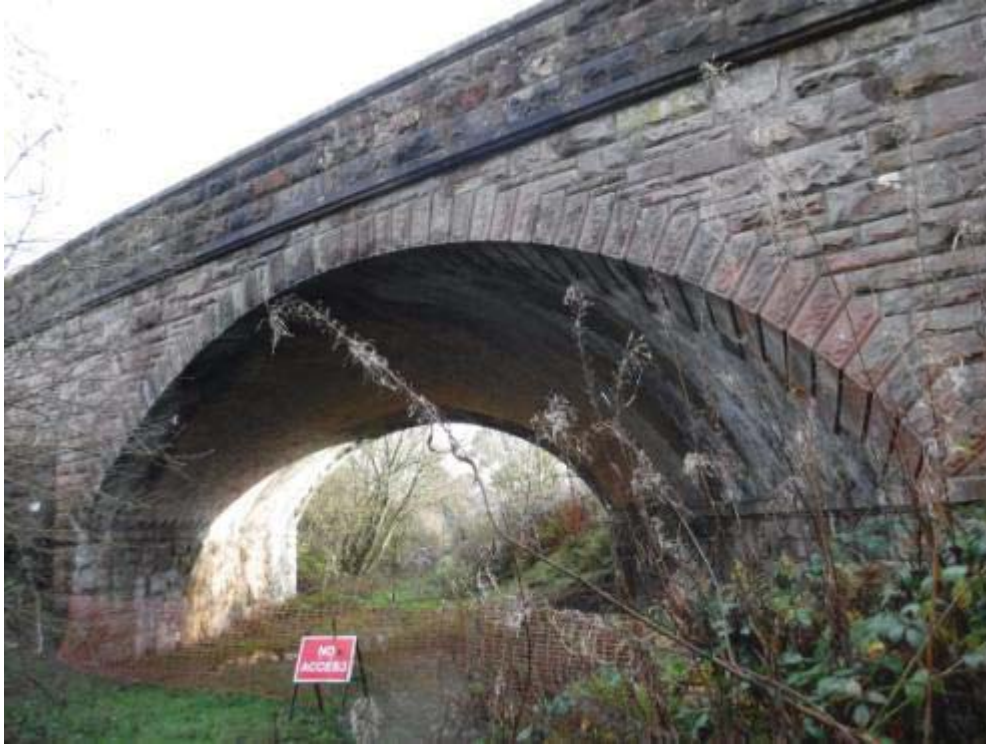
Photo No.5 - Arch ring soffit: View.
