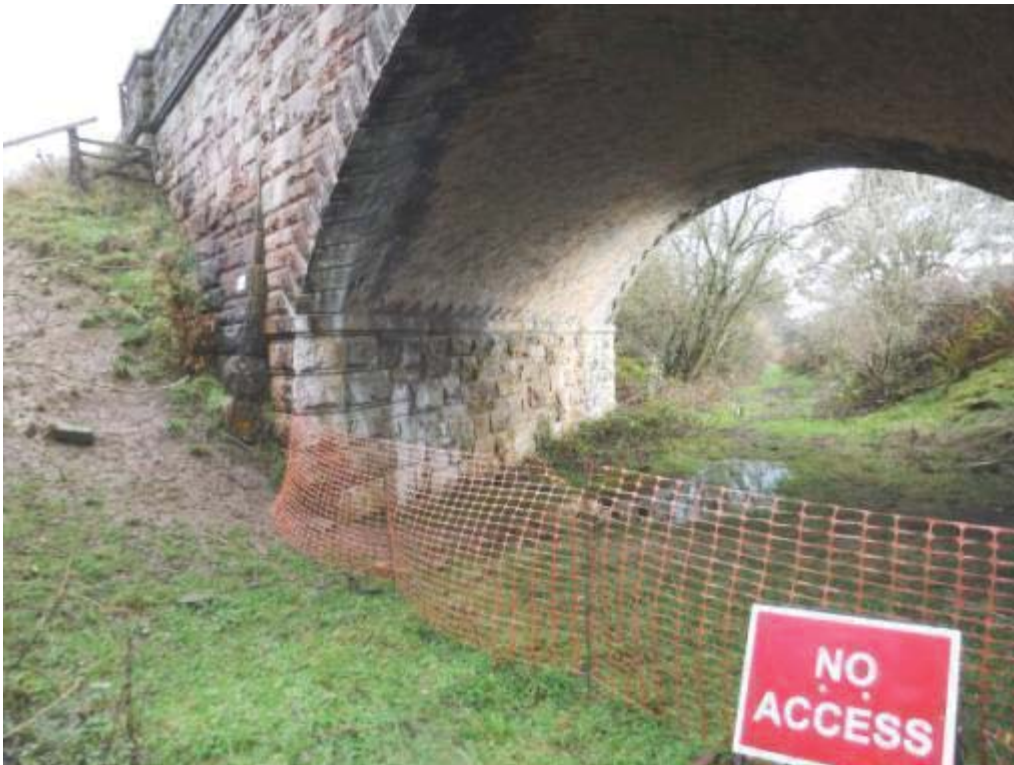
Photo No.54 - East abutment: View.
