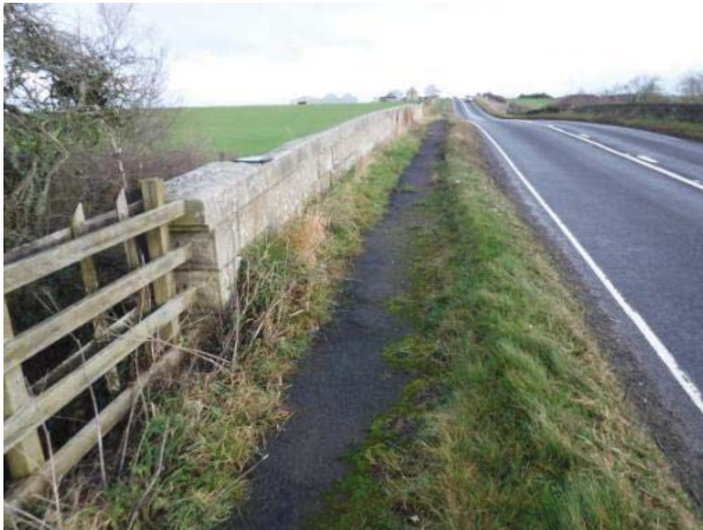
Photo No.100 - North roadside parapet: View.
