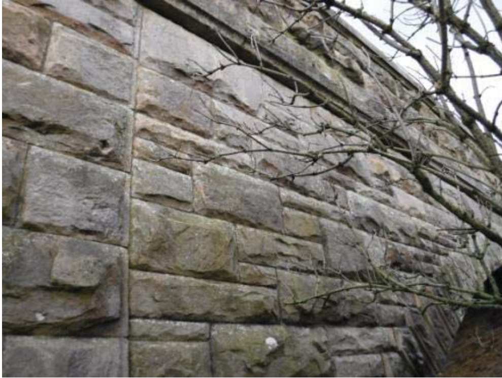
Photo No.51 - South spandrel: Typical example of the condition.
