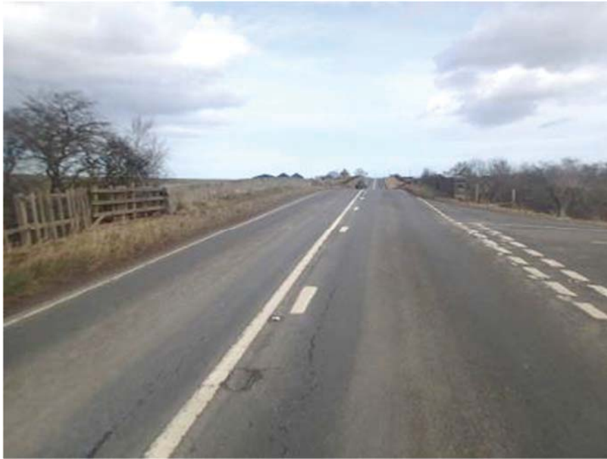
Photograph 7: general view over the structure from the west looking east
