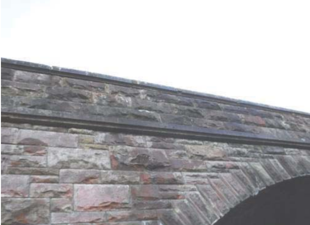
Photo No.121 - North outer parapet: Typical example of the condition.
