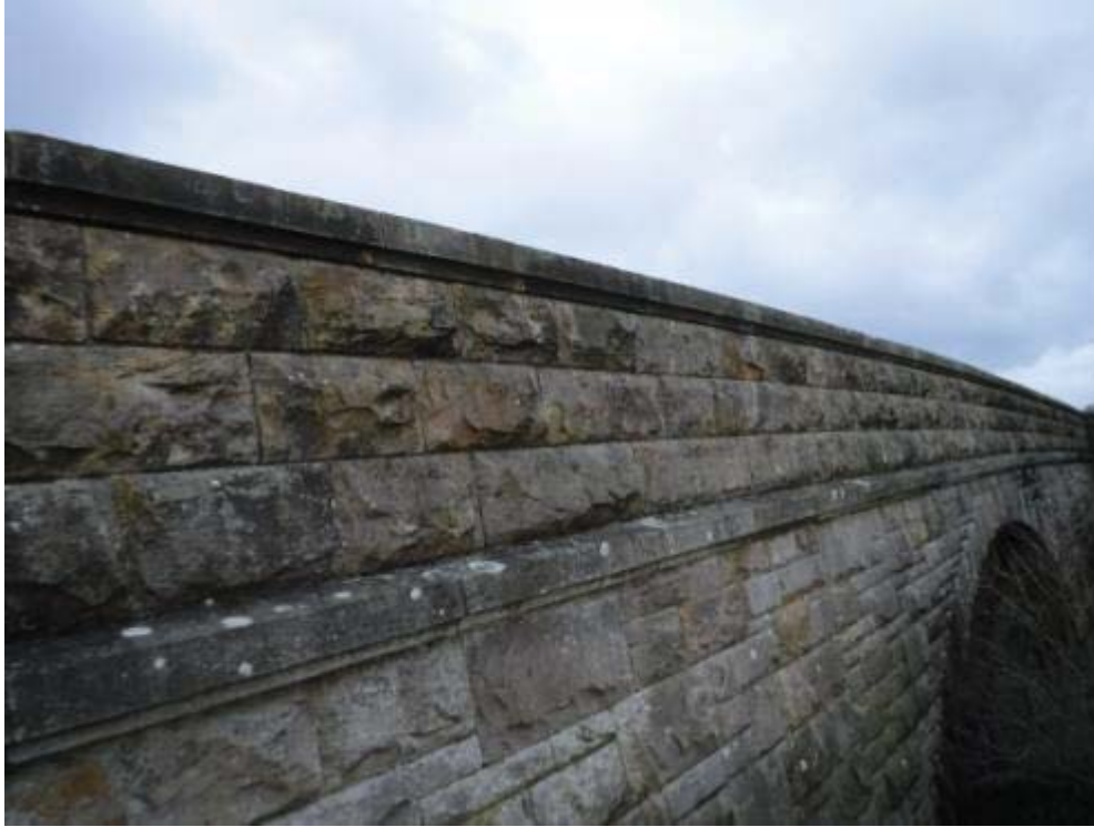
Photo No.139 - South outer parapet: Typical example of the condition.
