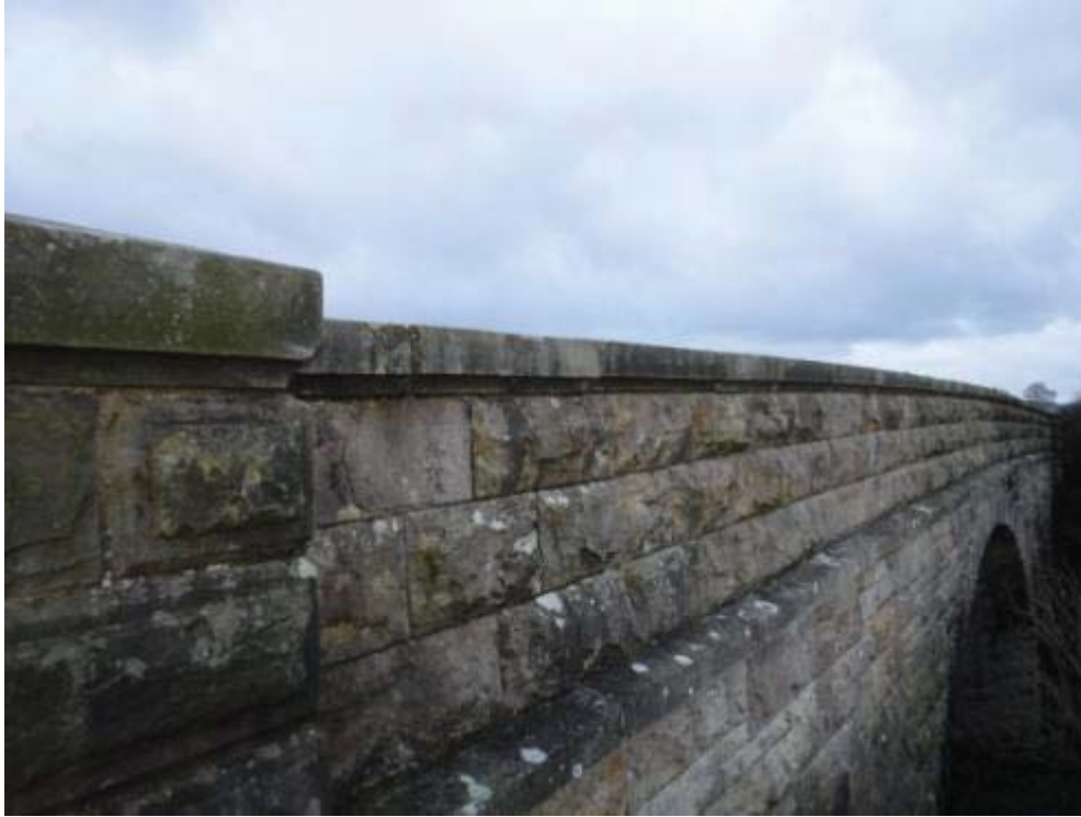
Photo No.137 - South outer parapet: View.
