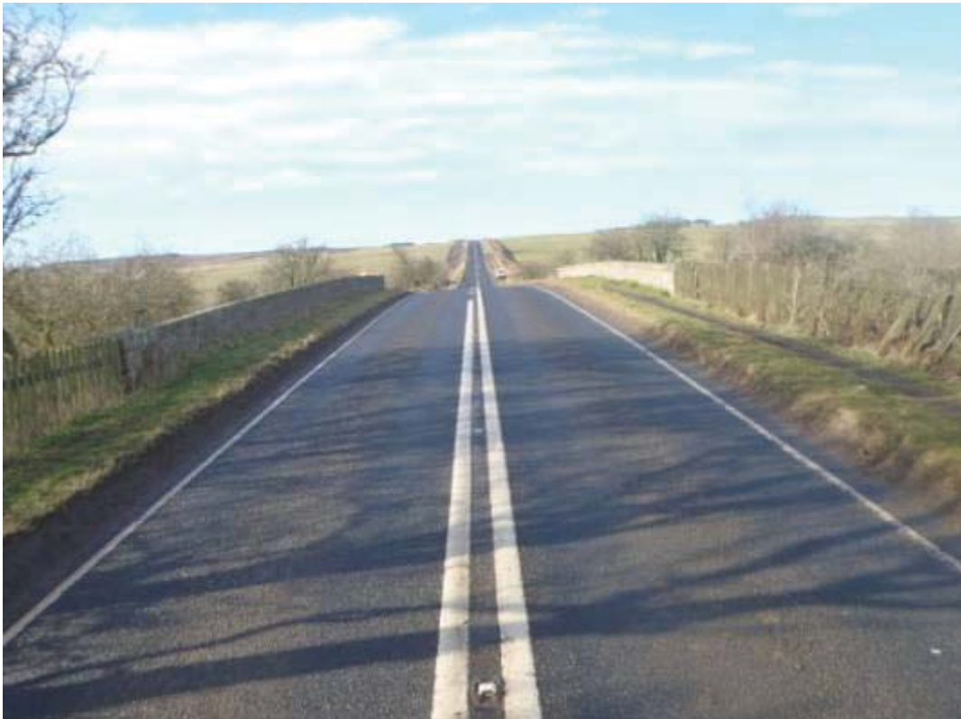
Photo No.3: View: Across Structure.
