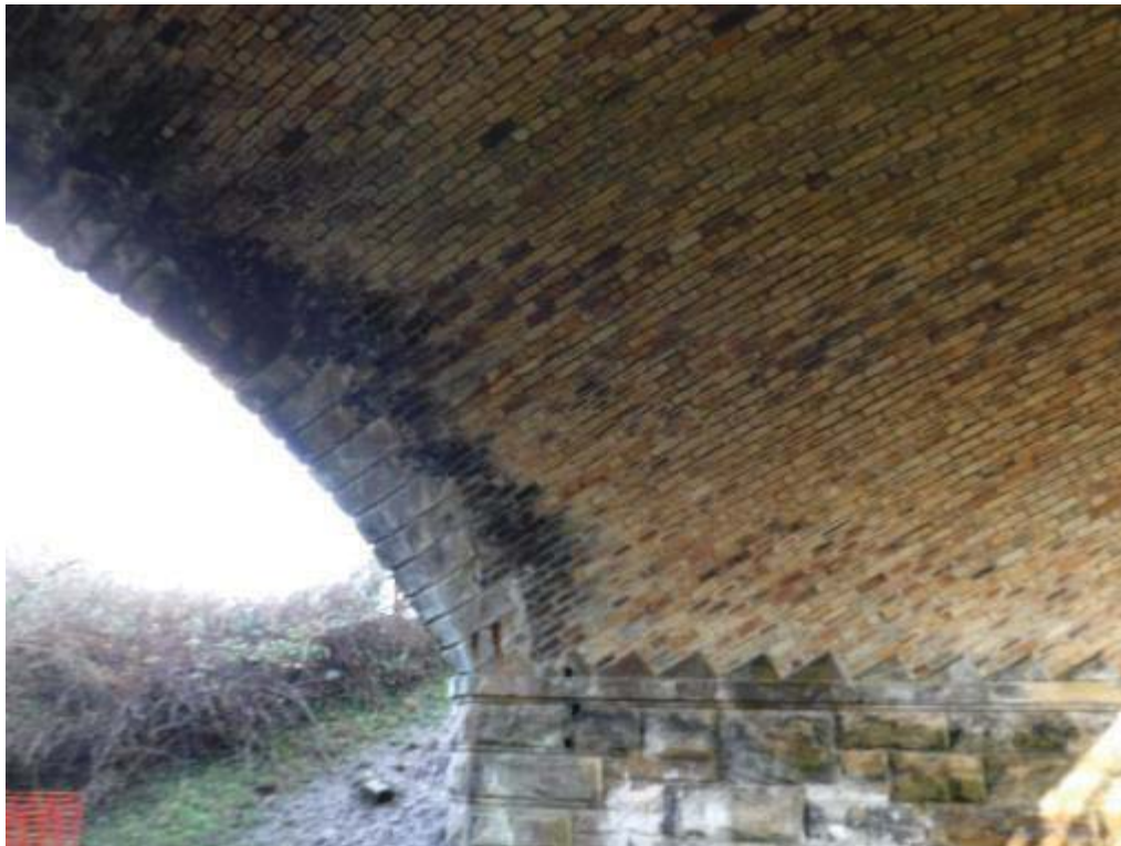
Photo No.10 - Arch ring soffit: Typical example of the condition.
