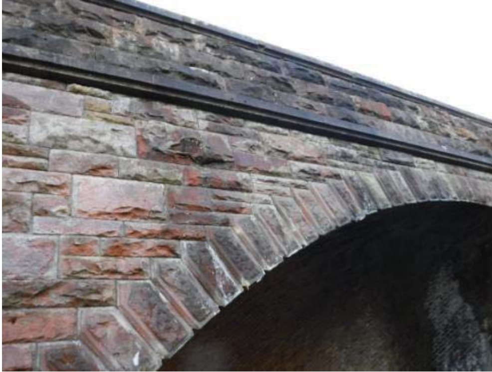
Photo No.41 - North spandrel: Typical example of the condition.
