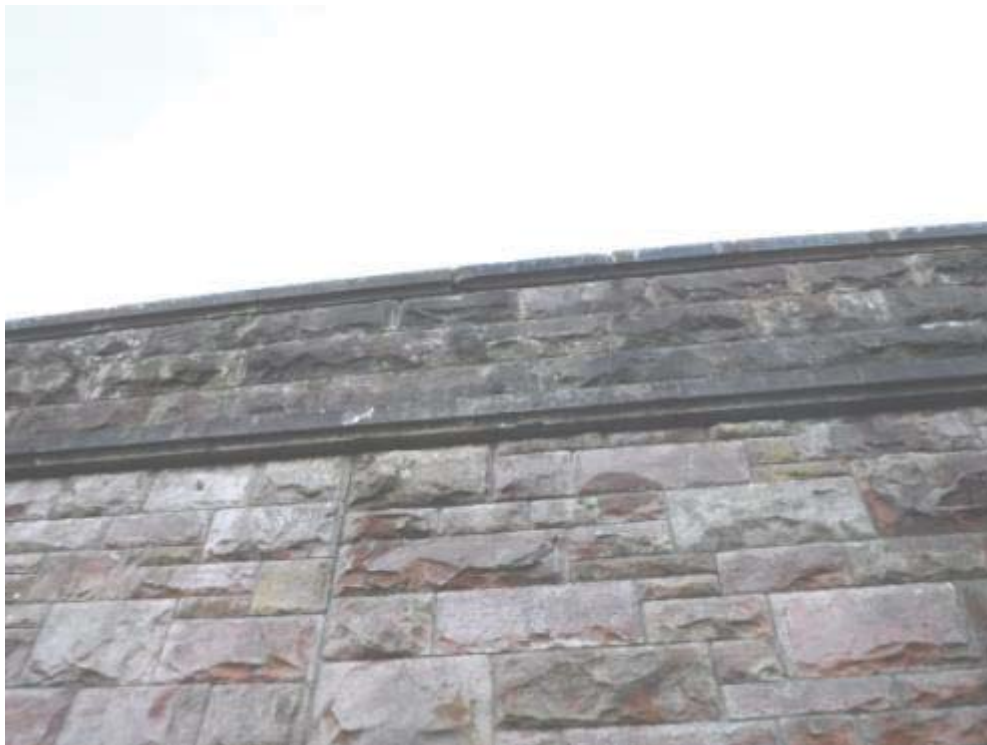
Photo No.122 - North outer parapet: Typical example of the condition.
