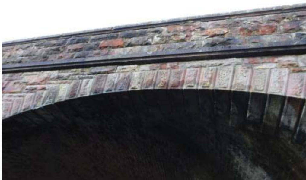
Photo No.30 - North arch ring face: Typical example of the condition.
