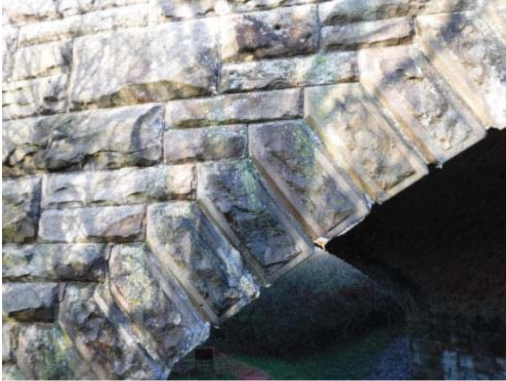
Photo No.19 - South arch ring face: Typical example of the condition.
