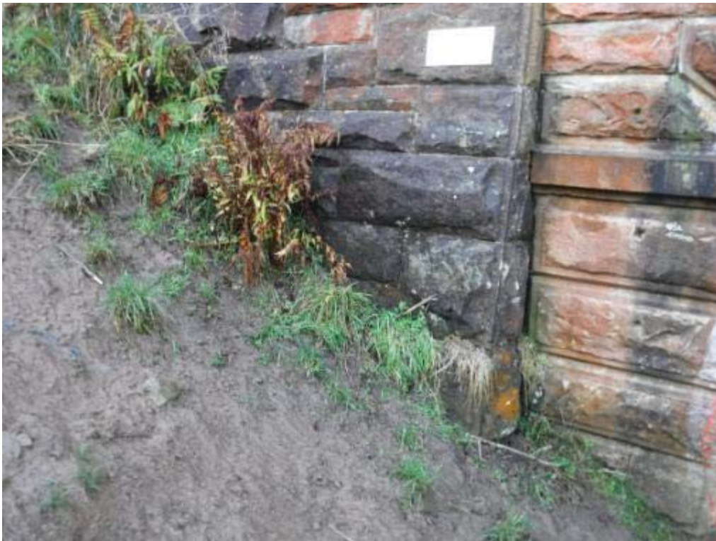
Photo No.78 - N/E wing wall: Typical example of the condition.
