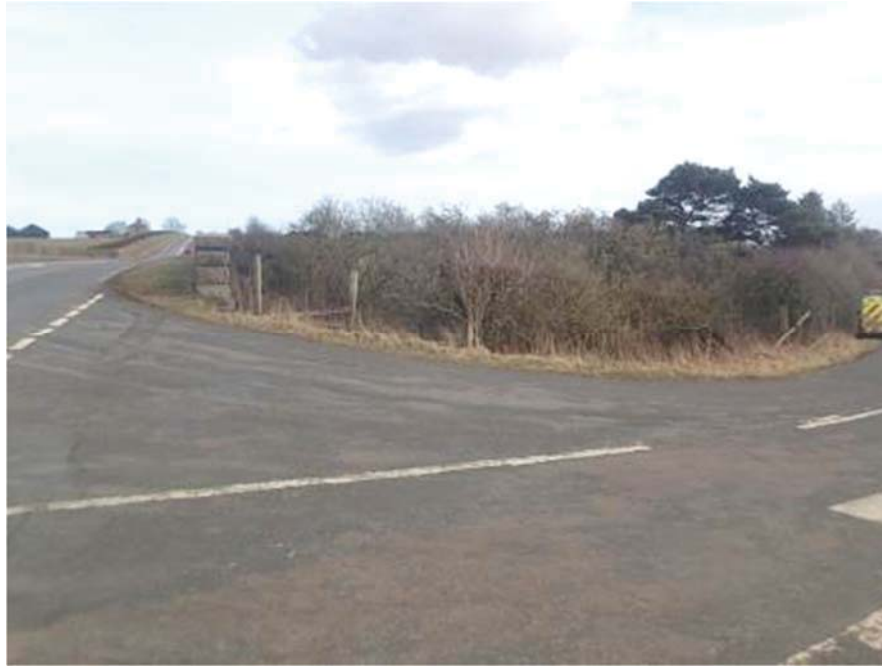
Photograph 18: long-standing failure of the southwest fence line
