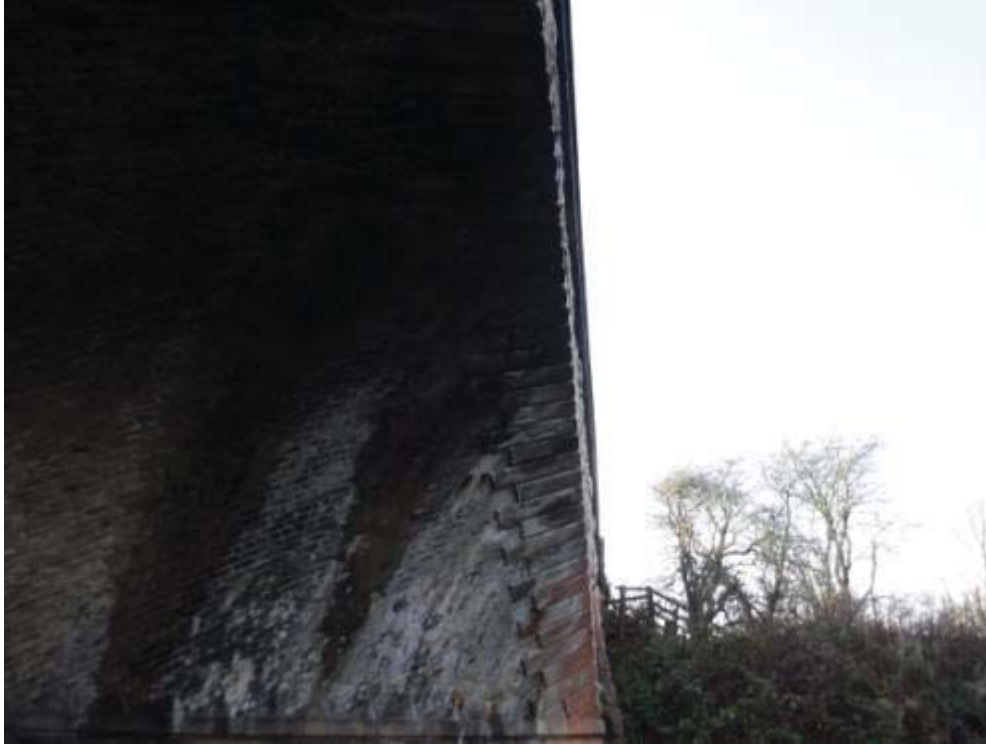
Photo No.13 - Arch ring soffit: Typical example of the condition.
