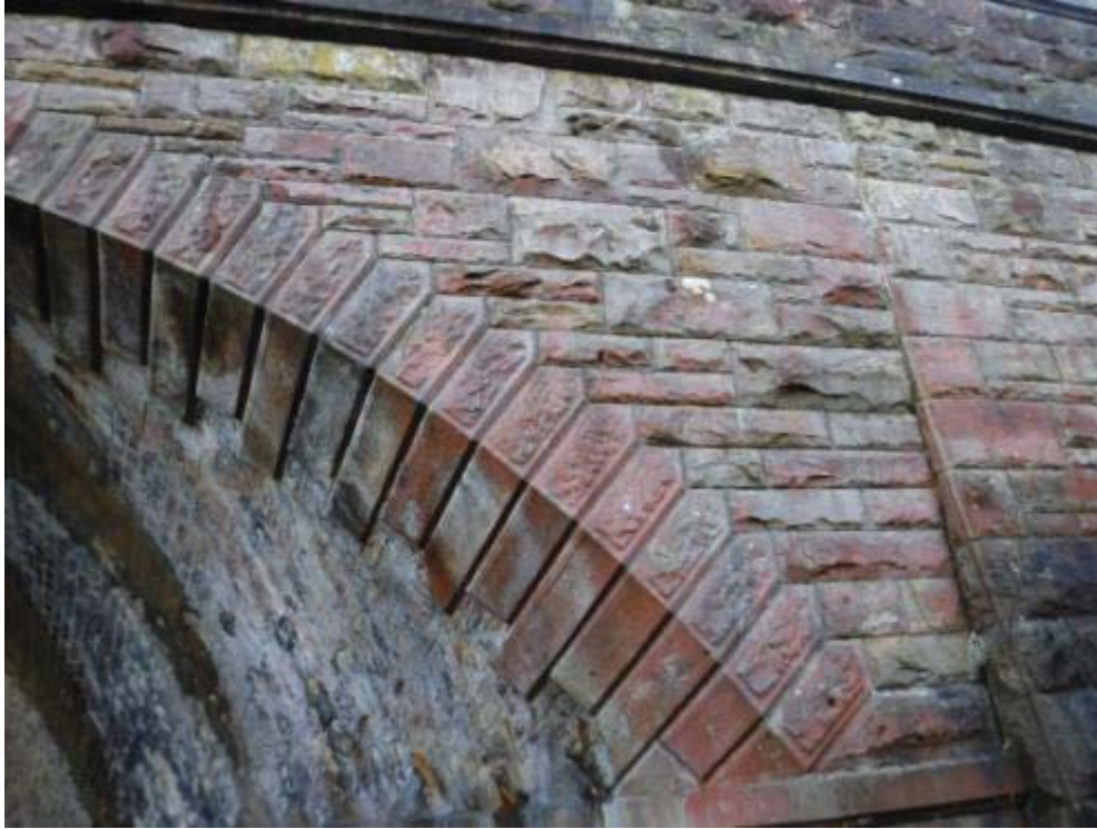
Photo No.27 - North arch ring face: Typical example of the condition.
