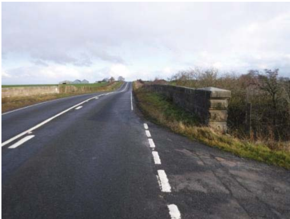
Photo No.126 - South roadside parapet: View.
