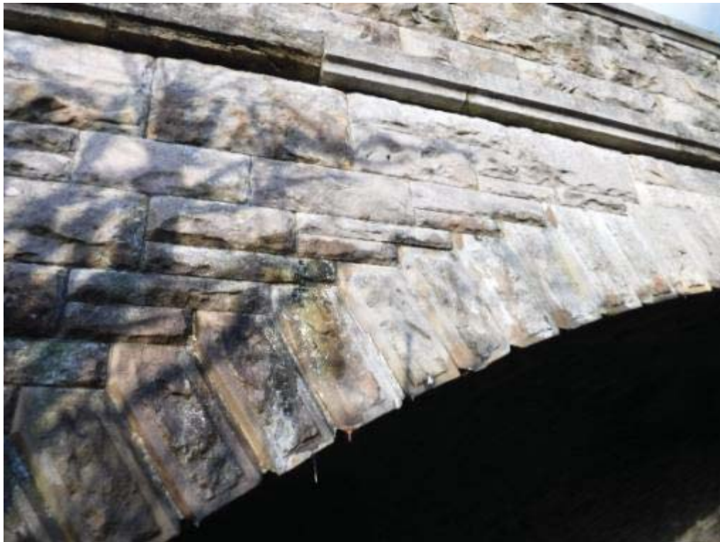
Photo No.20 - South arch ring face: Typical example of the condition.
