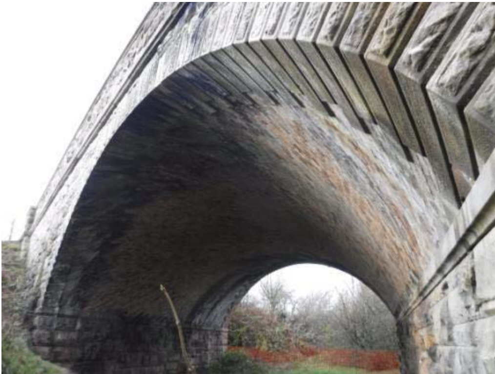
Photo No.6 - Arch ring soffit: View.
