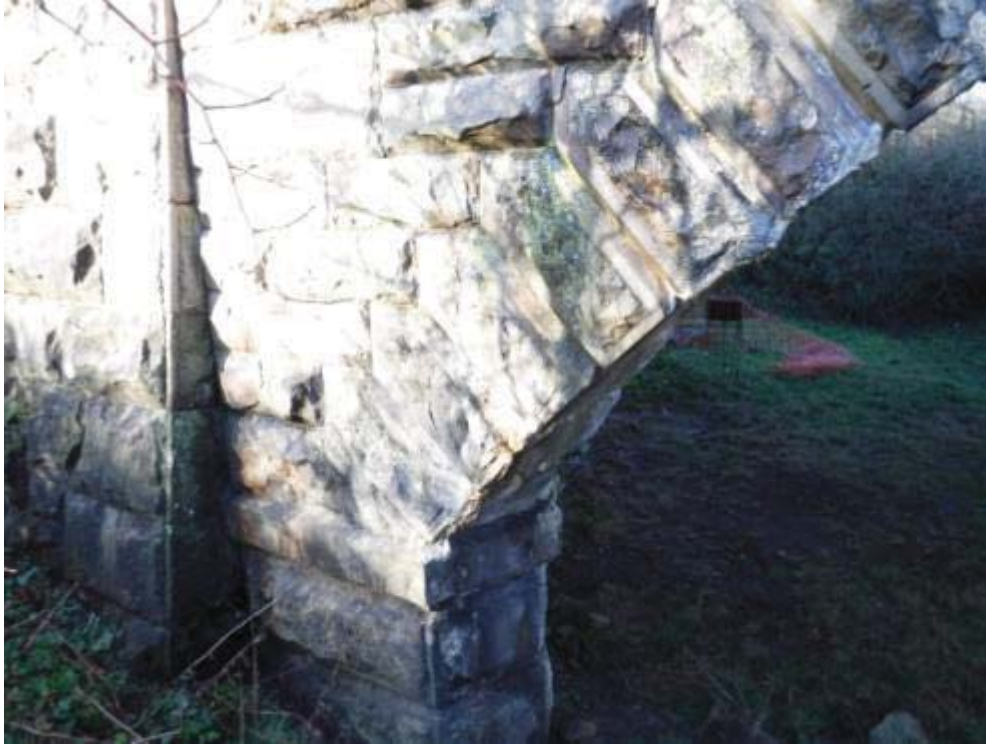
Photo No.17 - South arch ring face: Typical example of the condition.
