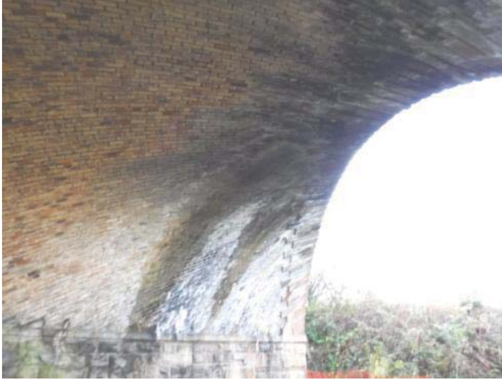
Photo No.11 - Arch ring soffit: Typical example of the condition.
