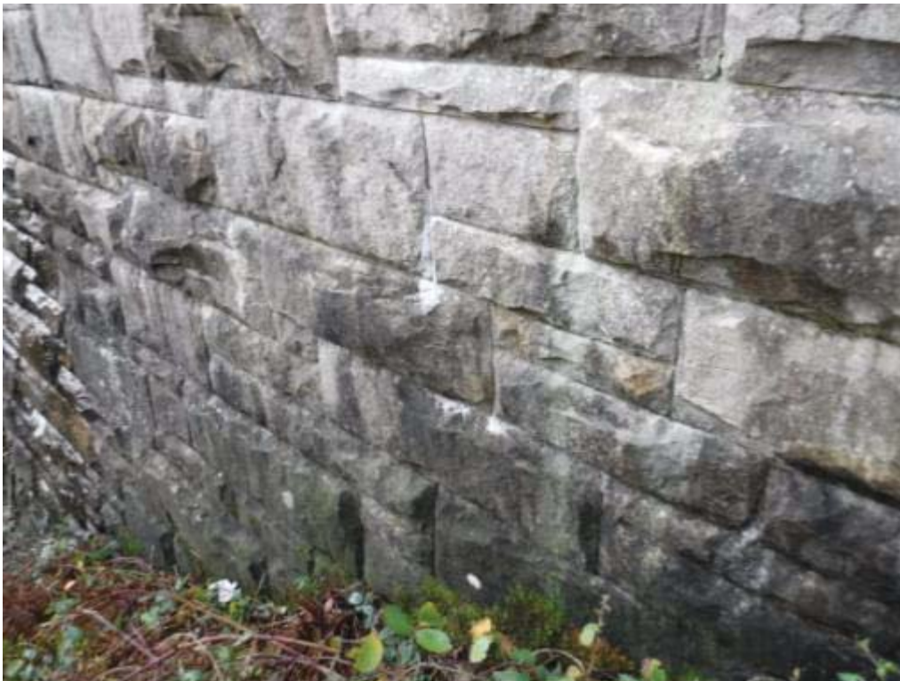
Photo No.90 - S/E wing wall: Typical example of the condition.
