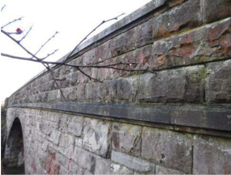
Photo No.119 - North outer parapet: Typical example of the condition.
