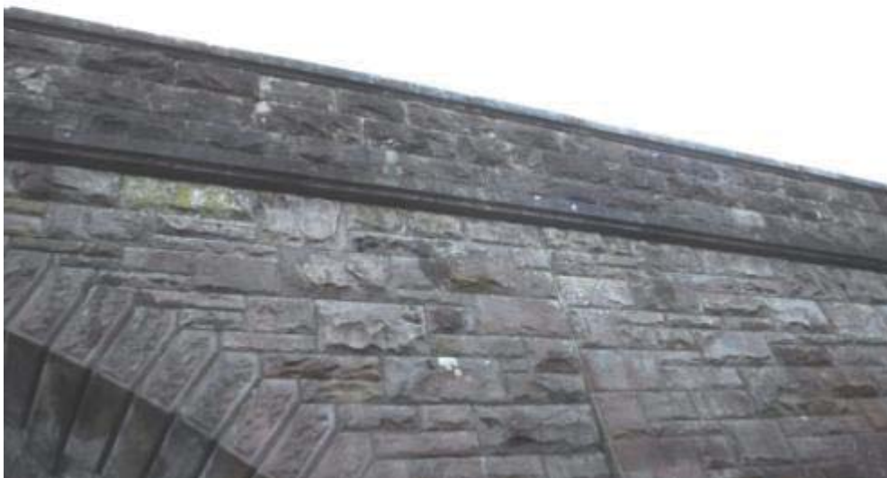
Photo No.120 - North outer parapet: Typical example of the condition.
