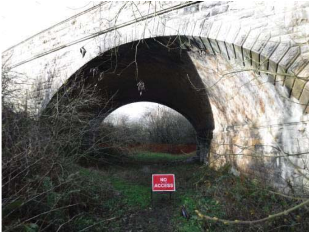
Photo No.16 - South arch ring face: View.
