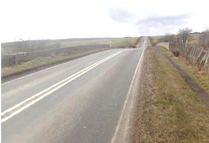
Photograph 8: general view over the structure from the east looking west
