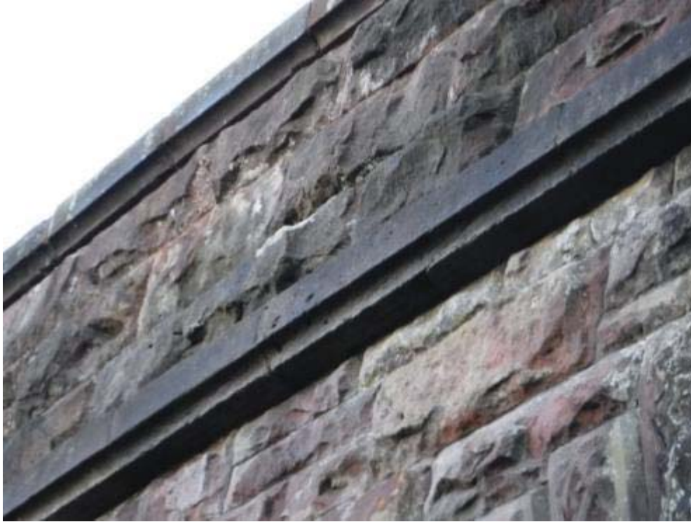
Photo No.157 - String course: Typical example of the condition.
