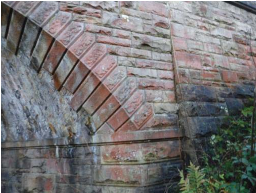
Photo No.26 - North arch ring face: Typical example of the condition.
