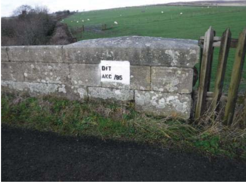
Photo No.167 - Structure I.D.
