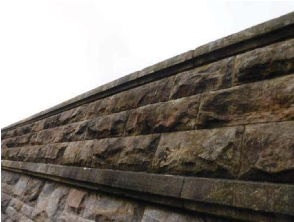
Photo No.140 - South outer parapet: Typical example of the condition.
