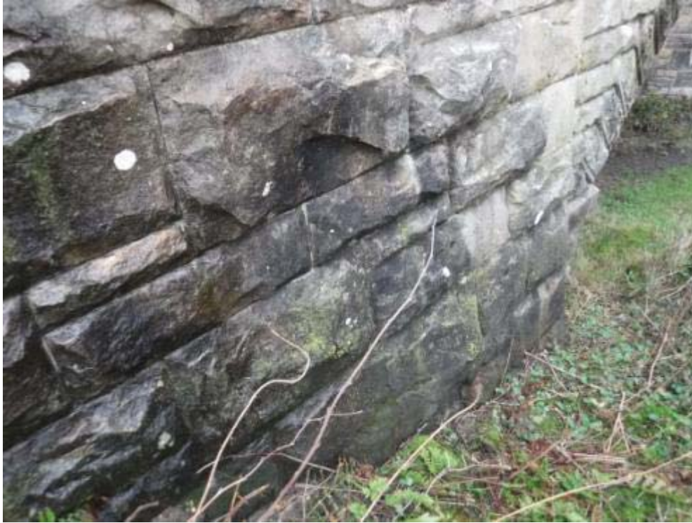
Photo No.97 - S/W wing wall: Typical example of the condition.
