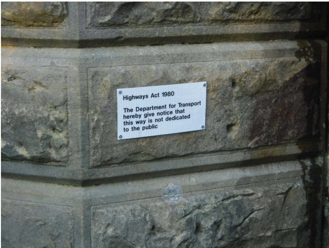
Photo No.5: Non - Dedication plate: Installed to the substructure.
