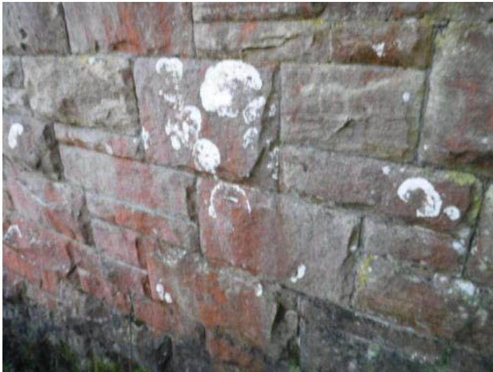
Photo No.82 - N/W wing wall: Typical example of the condition.
