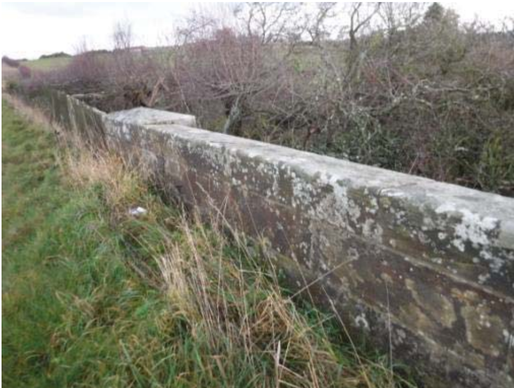
Photo No.134 - South roadside parapet: Typical example of the condition.
