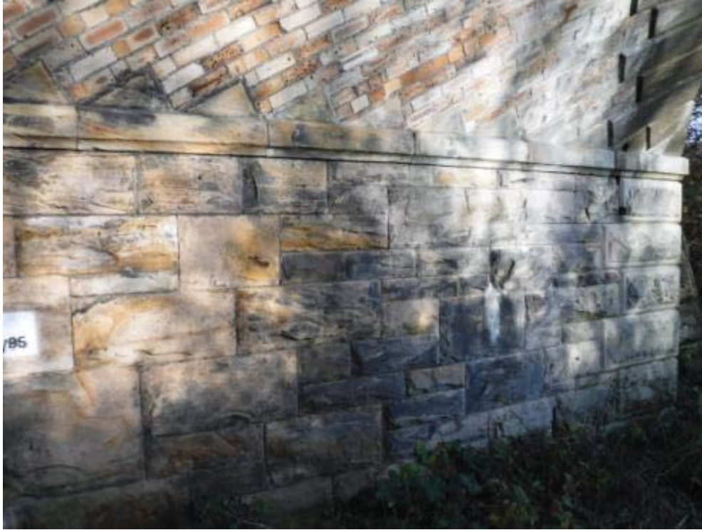
Photo No.61 - East abutment: Typical example of the condition.
