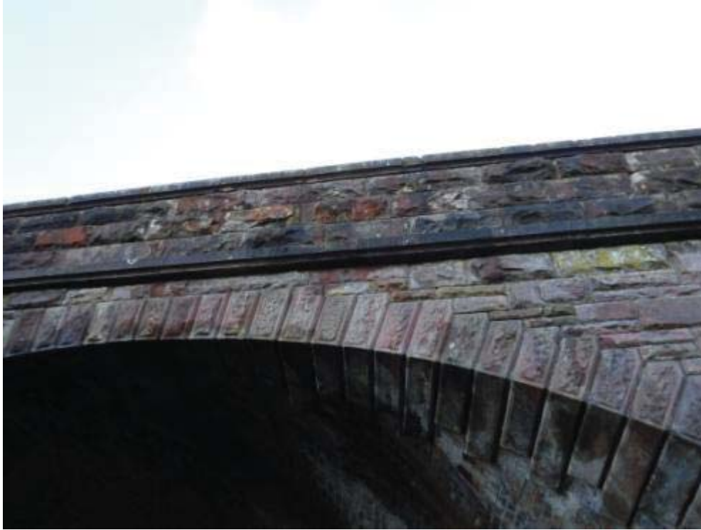
Photo No.29 - North arch ring face: Typical example of the condition.
