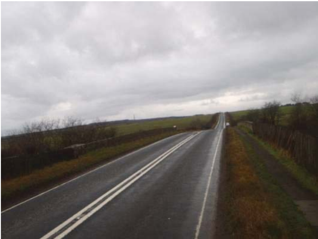
Photo No.9: View: Across Structure.
