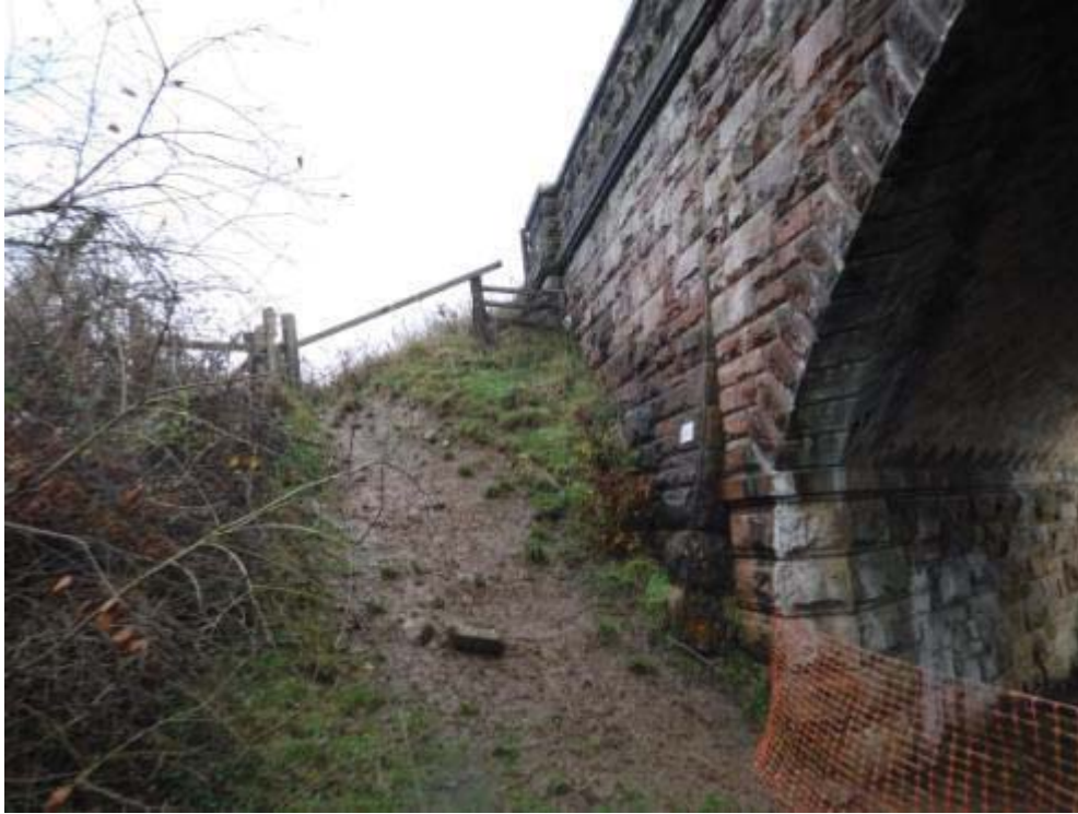
Photo No.75 - N/E wing wall: View.
