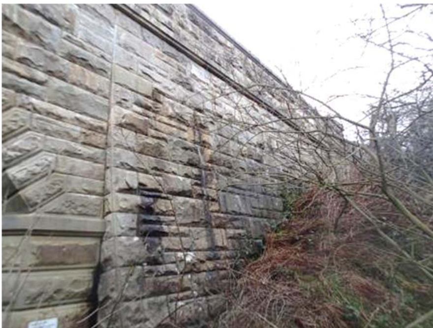
Photograph 6: general view of the southeast wingwall
