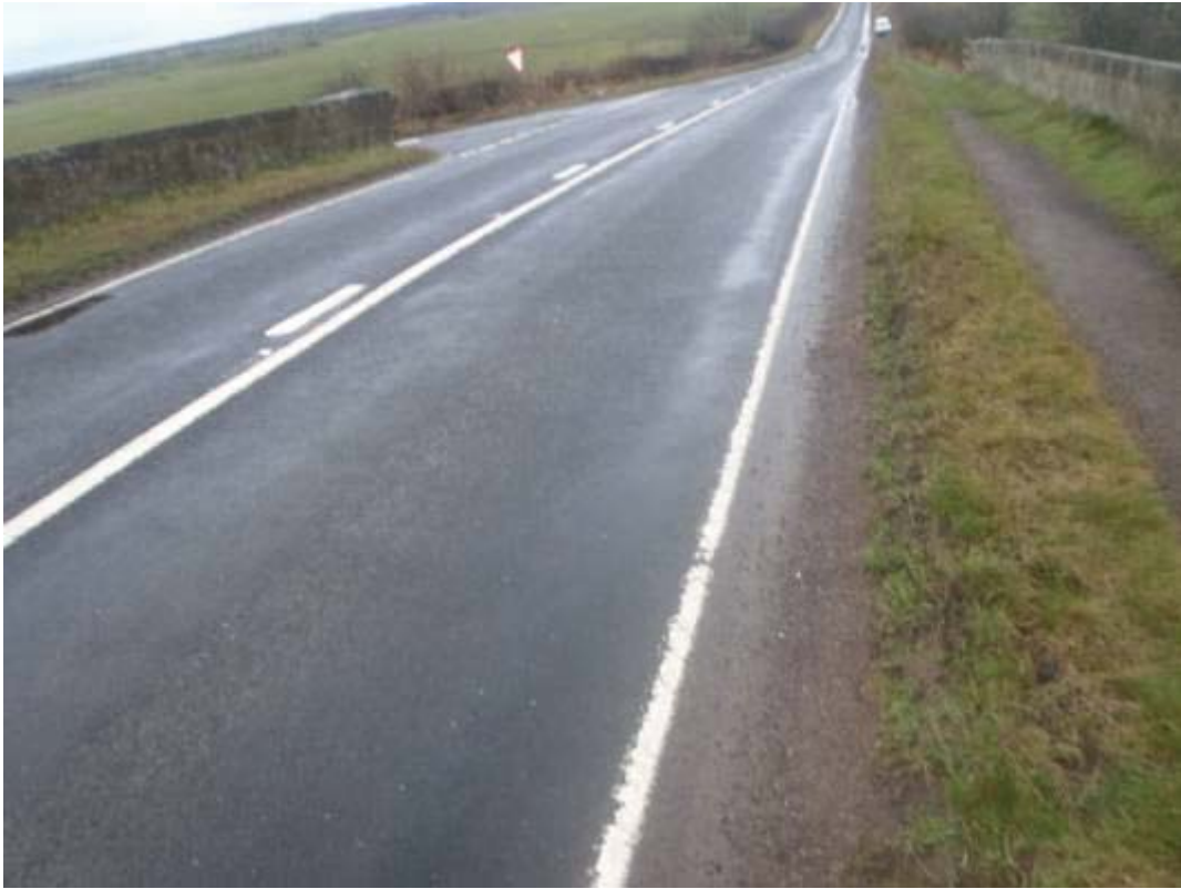
Photo No.2: Road surface: Typical example of the condition.
