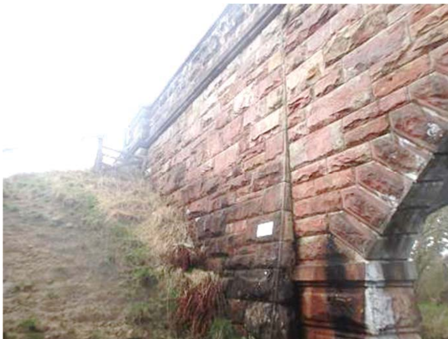
Photograph 4: general view of the northeast wingwall
