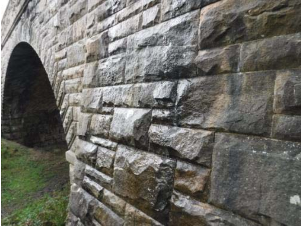
Photo No.91 - S/E wing wall: Typical example of the condition.
