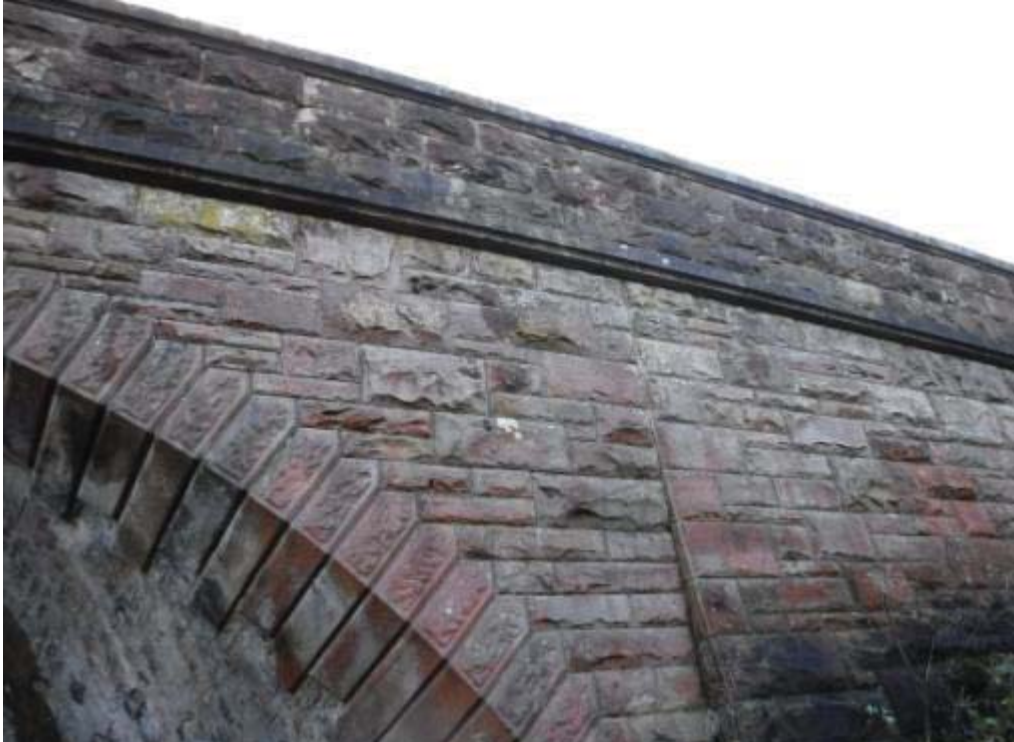
Photo No.43 - North spandrel: Typical example of the condition.
