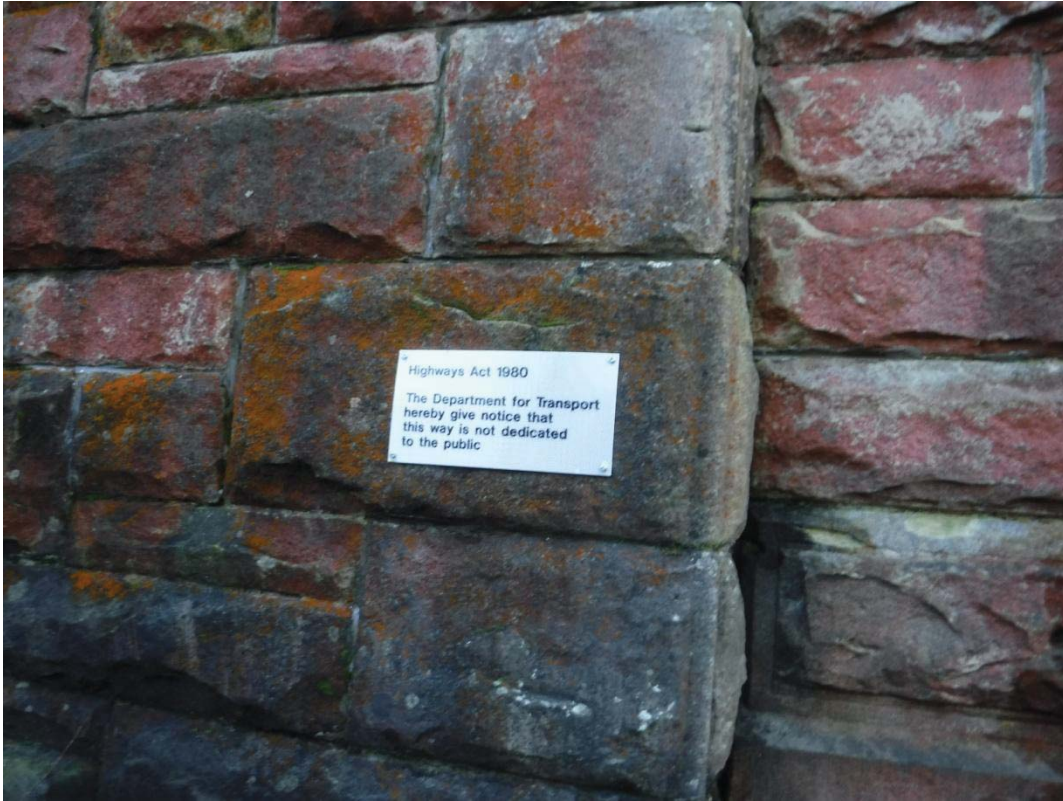
Photo No.4: Non - Dedication plate: Installed to the substructure.
