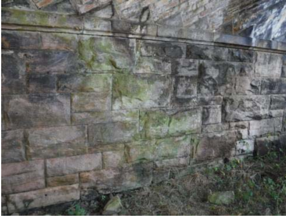
Photo No.69 - West abutment: Typical example of the condition.
