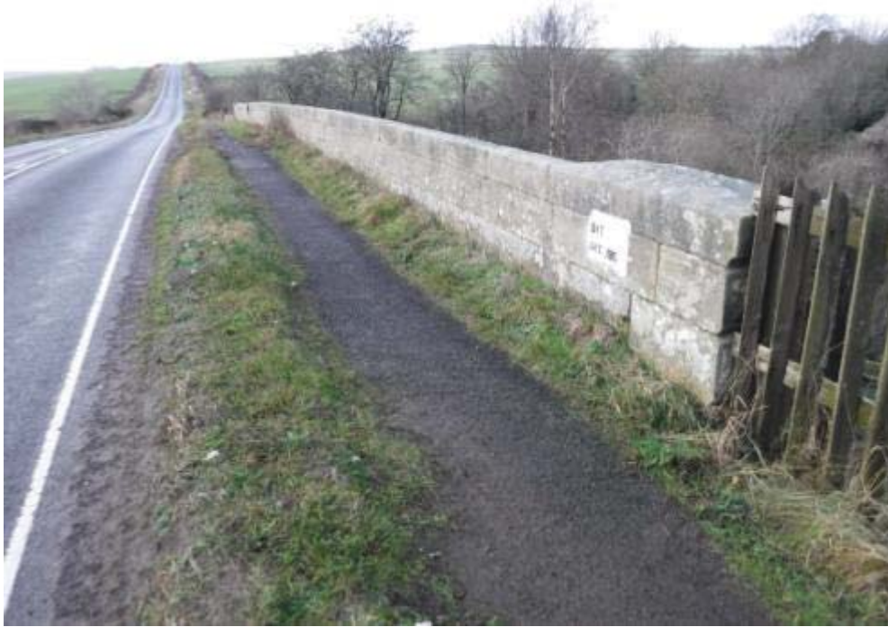
Photo No.113 - North roadside parapet: Typical example of the condition.
