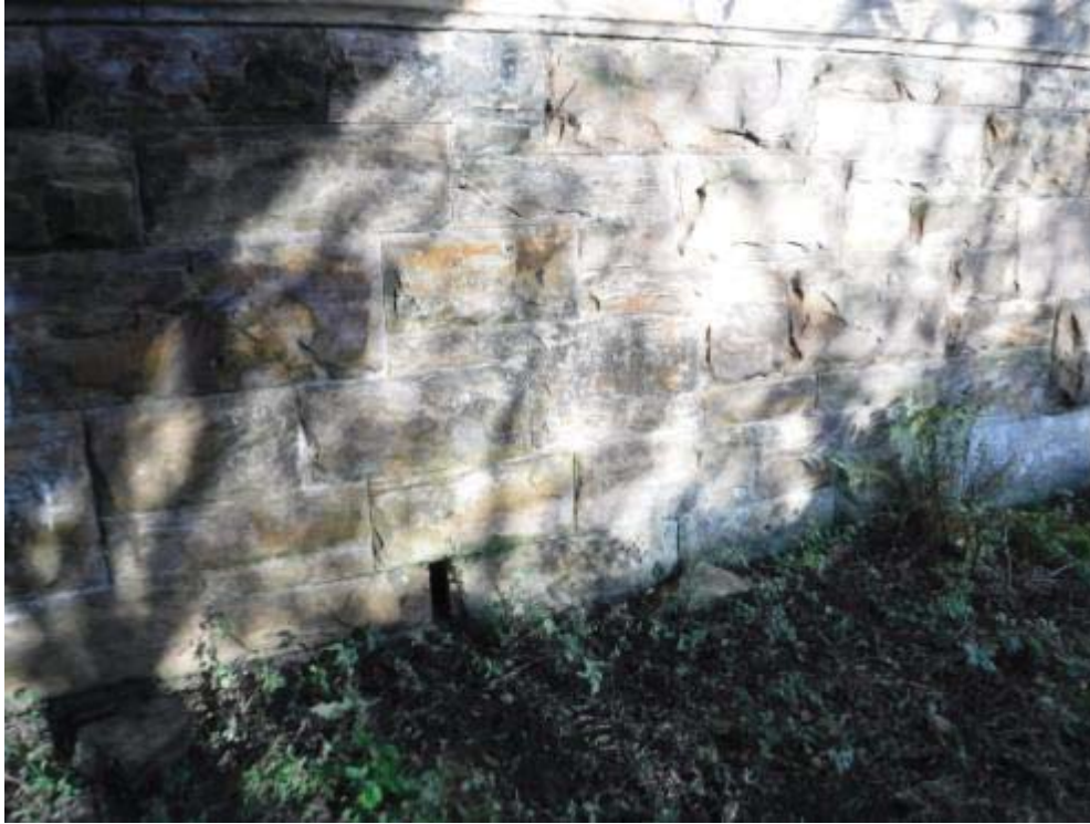
Photo No.59 - East abutment: Typical example of the condition.
