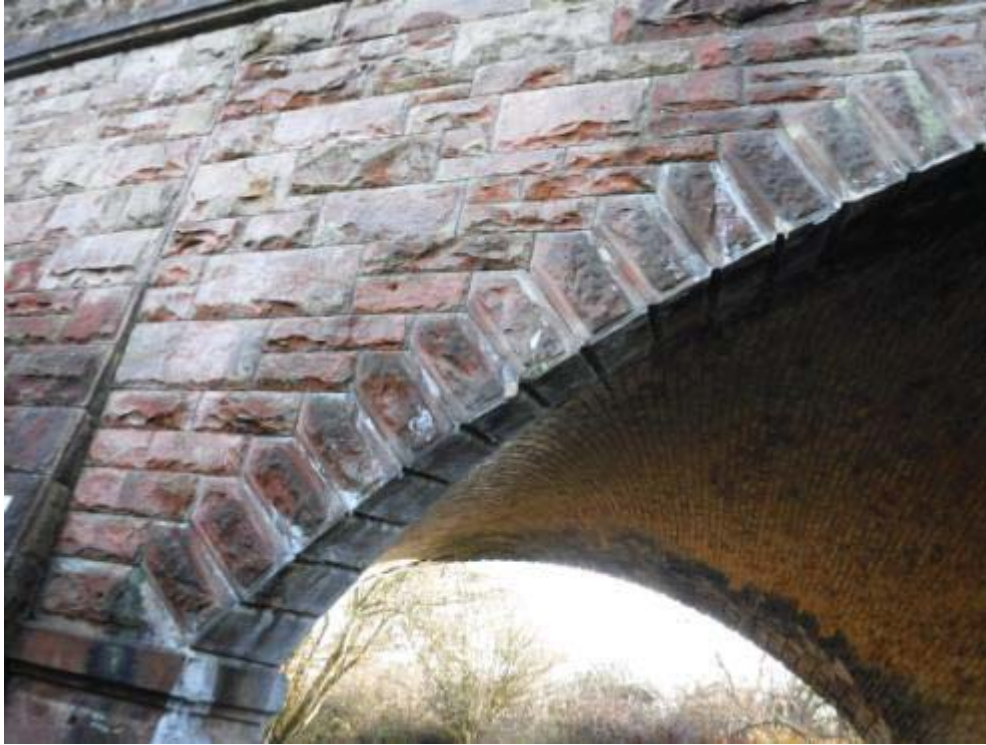
Photo No.33 - North arch ring face: Typical example of the condition.
