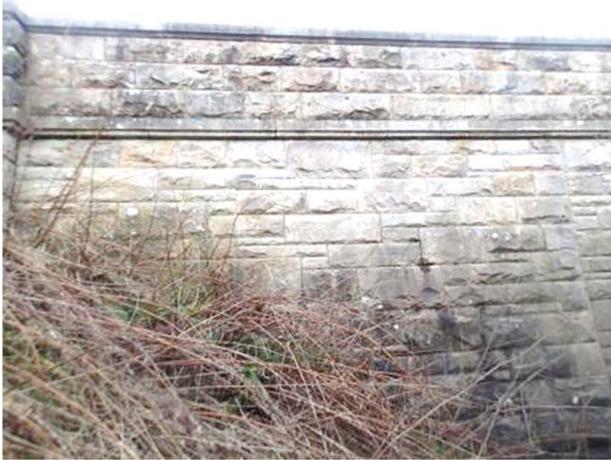
Photograph 5: general view of the southwest wingwall
