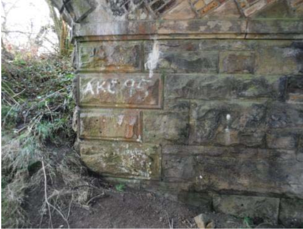
Photo No.67 - West abutment: Typical example of the condition.
