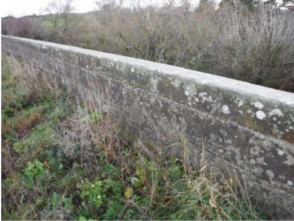
Photo No.131 - South roadside parapet: Typical example of the condition.
