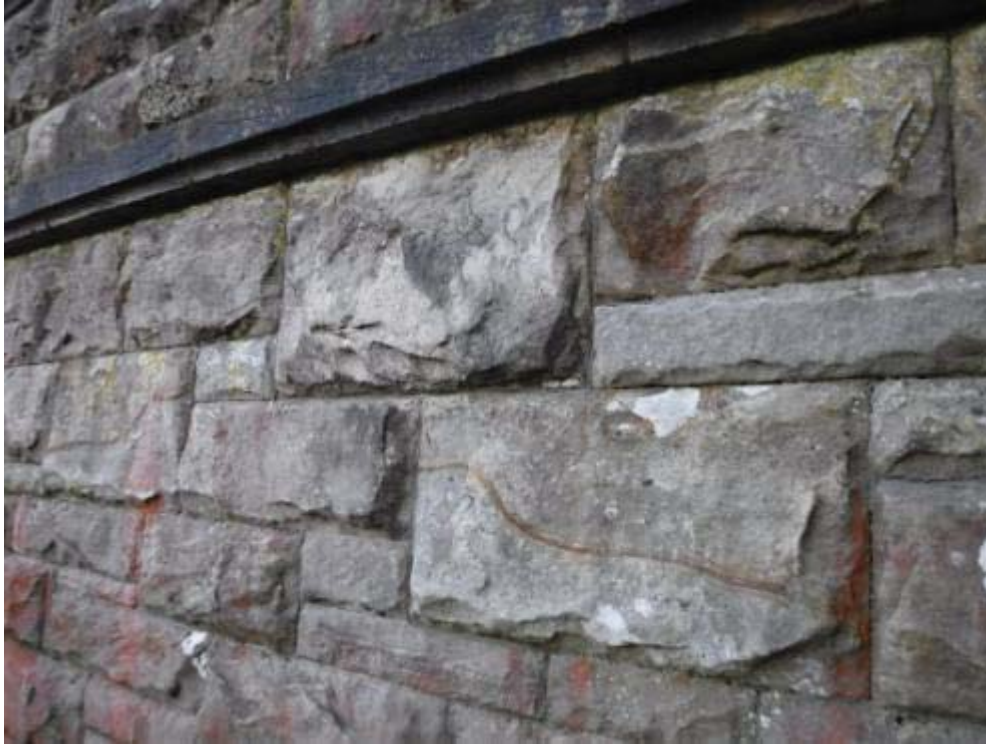
Photo No.83 - N/W wing wall: Typical example of the condition.
