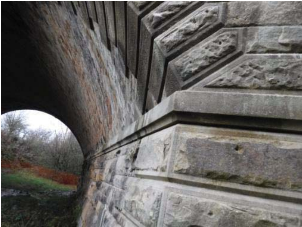
Photo No.146 - East springer course: View.
