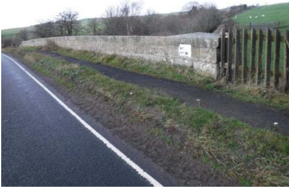
Photo No.101 - North roadside parapet: View.
