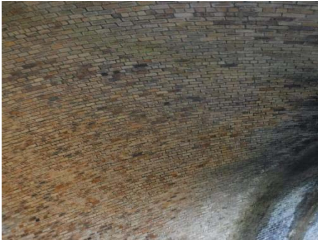
Photo No.12 - Arch ring soffit: Typical example of the condition.
