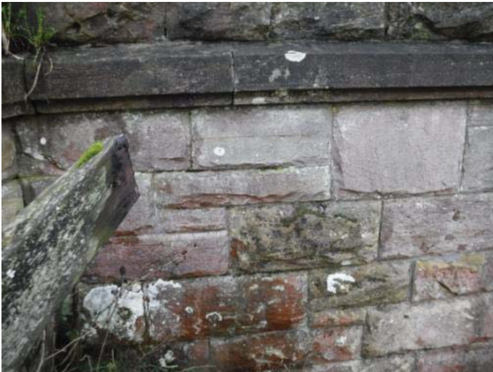
Photo No.76 - N/E wing wall: Typical example of the condition.
