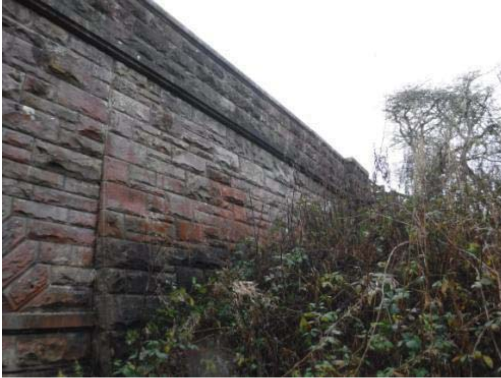
Photo No.81 - N/W wing wall: View.
