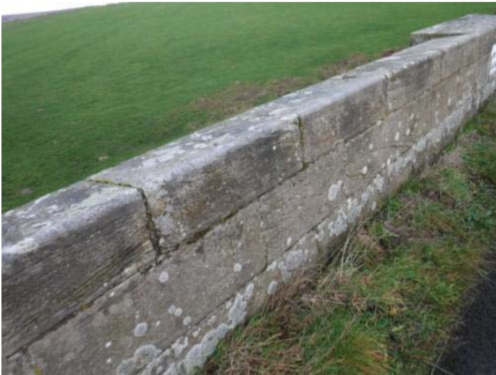
Photo No.112 - North roadside parapet: Typical example of the condition.
