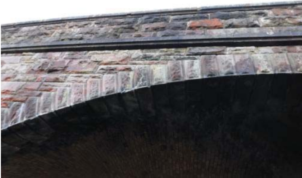
Photo No.31 - North arch ring face: Typical example of the condition.
