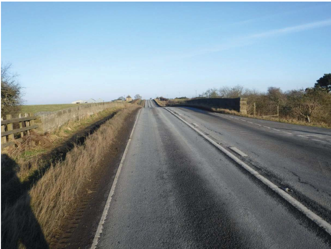
Photo No.9: View: Across Structure.
