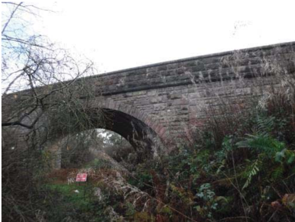
Photo No.2 – General view: {North}
