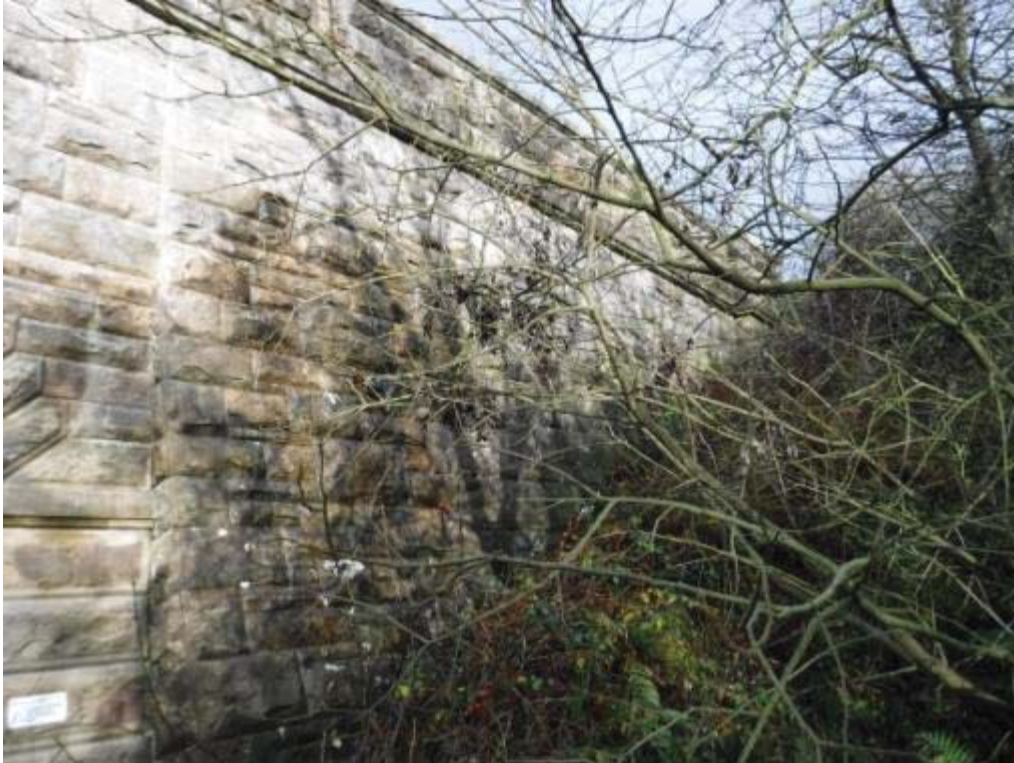
Photo No.87 - S/E wing wall: View.
