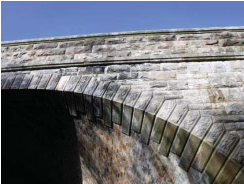
Photo No.50 - South spandrel: Typical example of the condition.
