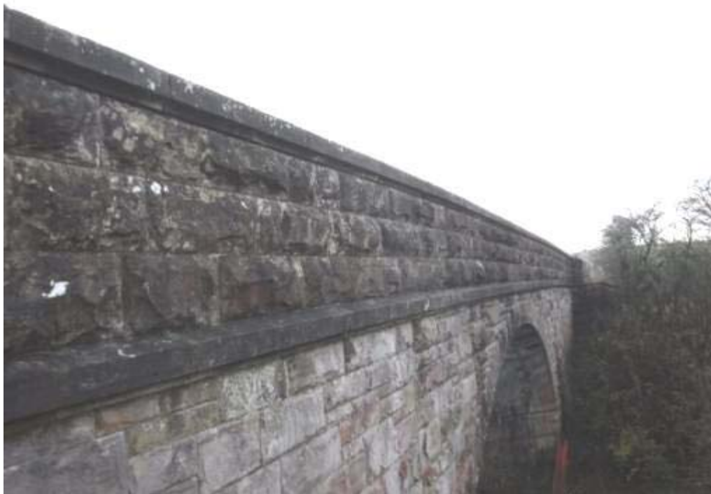
Photo No.116 - North outer parapet: View.
