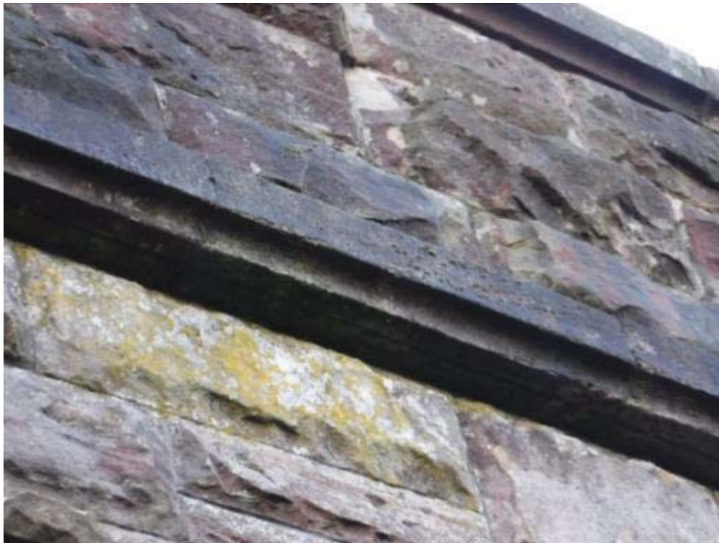
Photo No.156 - String course: Typical example of the condition.
