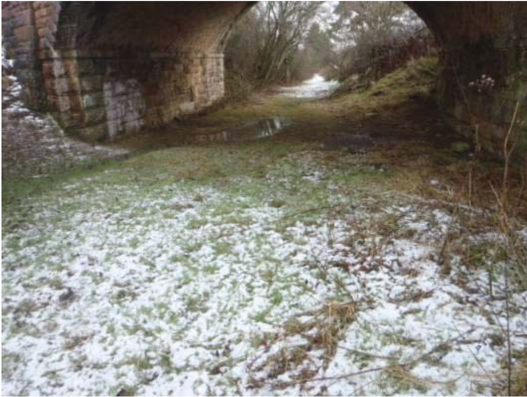
Photo No.2: Area under the structure: Typical example of the condition.
