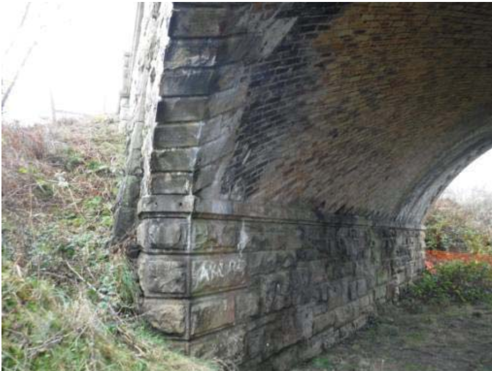
Photo No.150 - West springer course: View.
