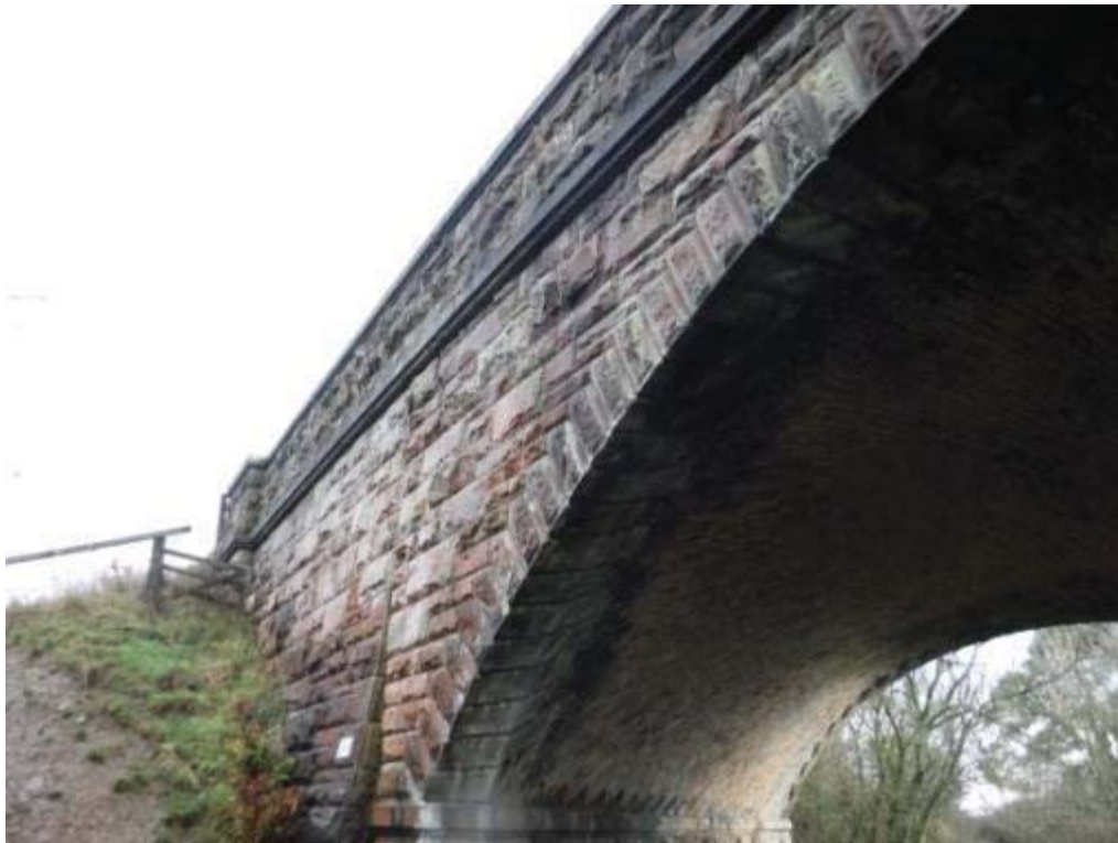
Photo No.36 - North spandrel: N/E view.
