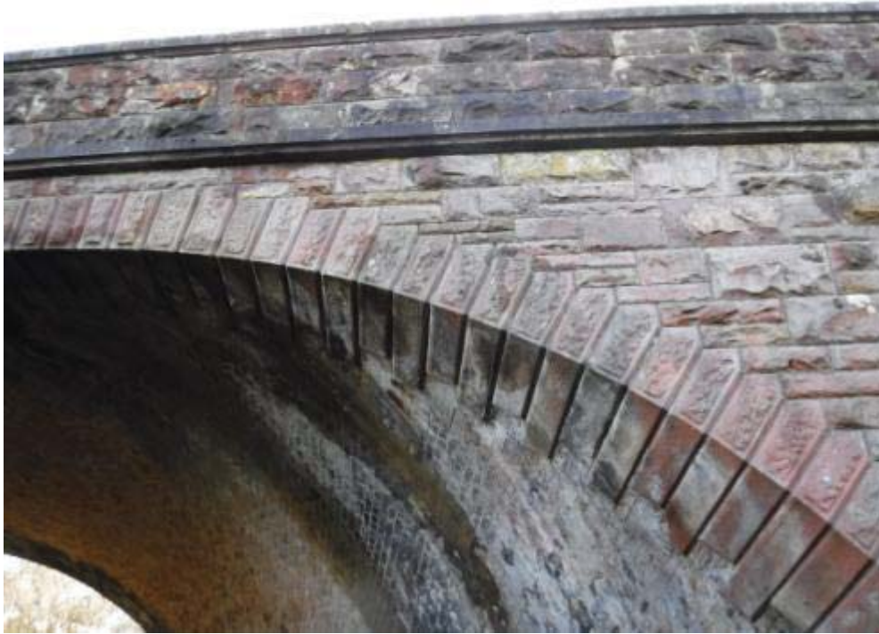
Photo No.45 - North spandrel: Typical example of the condition.
