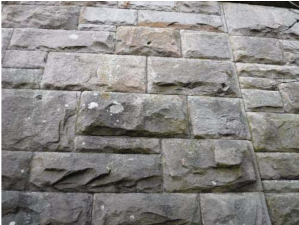
Photo No.98 - S/W wing wall: Typical example of the condition.
