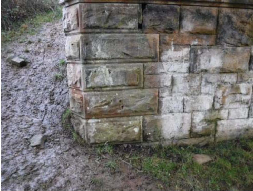
Photo No.57 - East abutment: Typical example of the condition.
