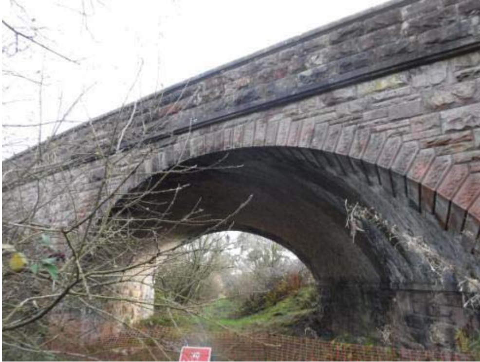
Photo No.7 - Arch ring soffit: Profile.
