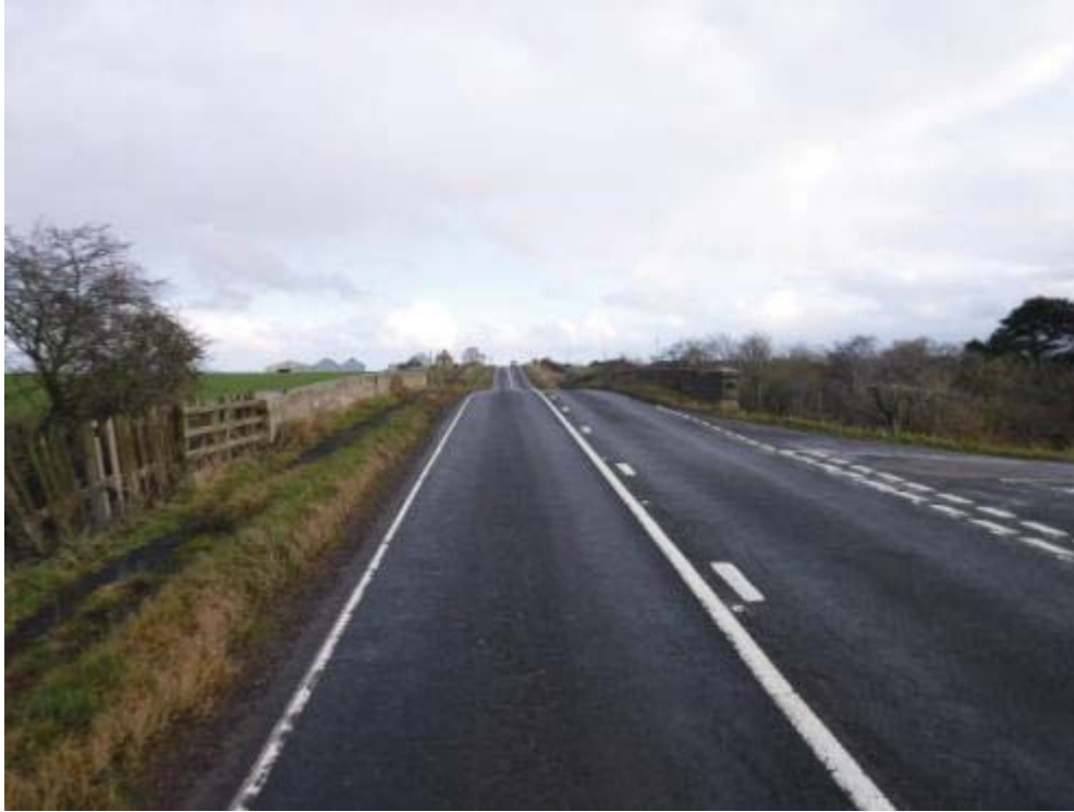
Photo No.3 – View: Across the structure looking east.
