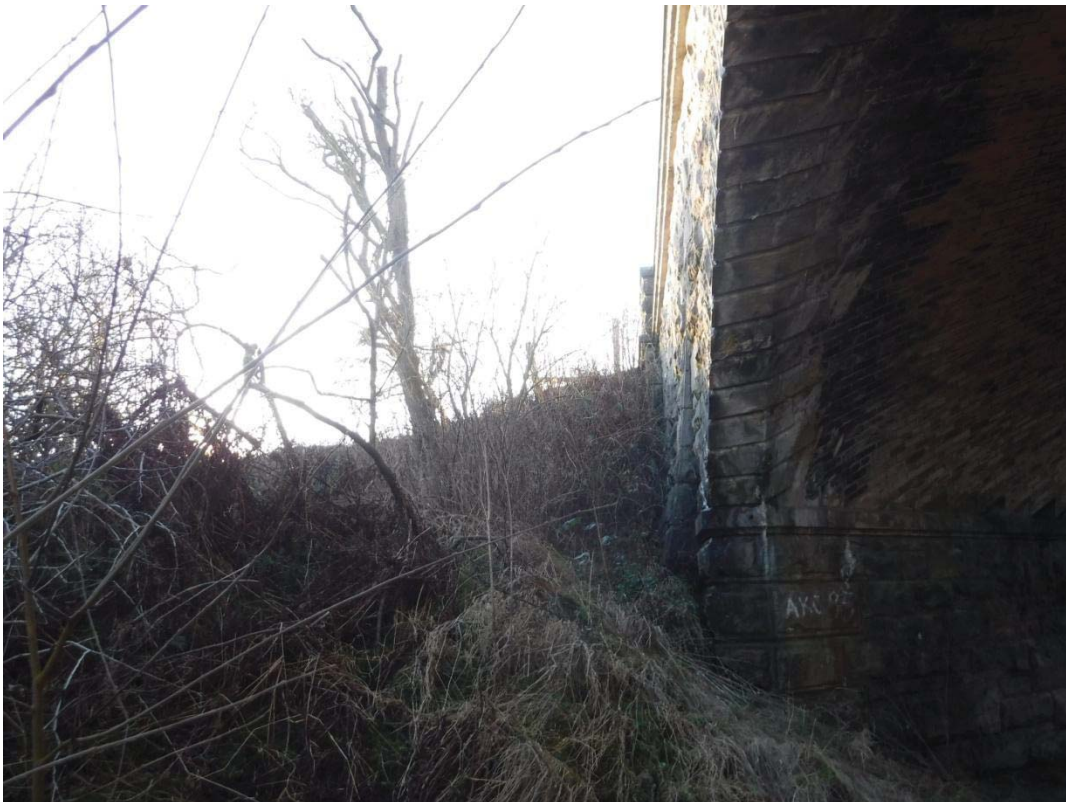
Photo No.7: Vegetation: Typical example.
