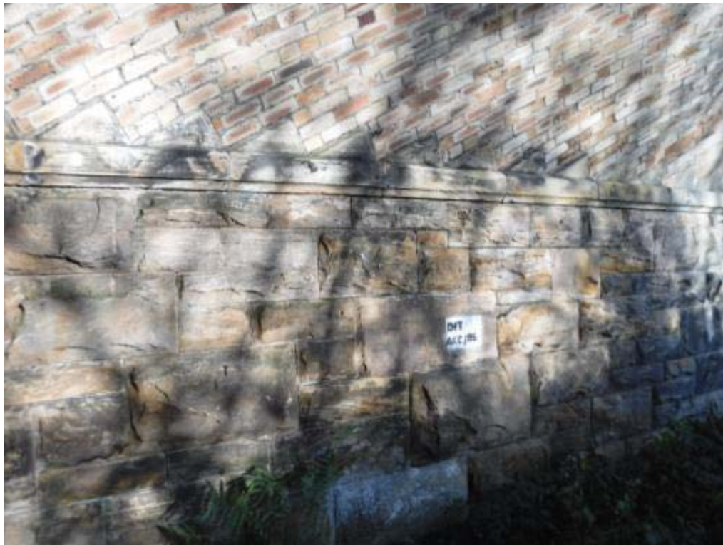
Photo No.60 - East abutment: Typical example of the condition.
