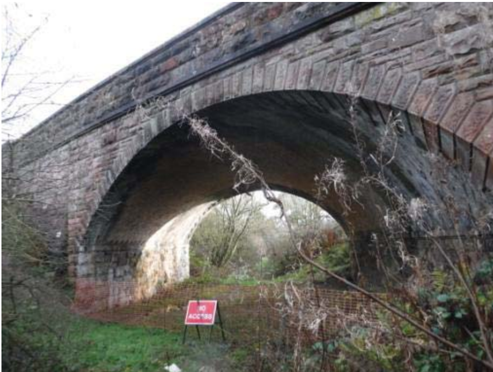
Photo No.158 - Area under the structure: Typical example.
