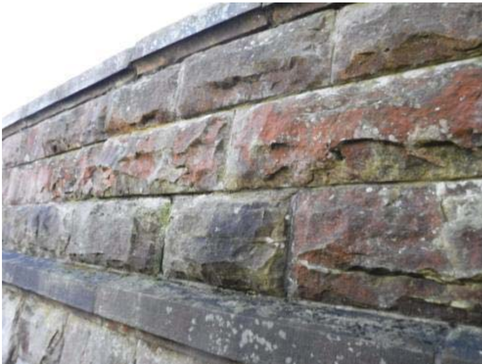
Photo No.118 - North outer parapet: Oversailing stonework at the N/W end.
