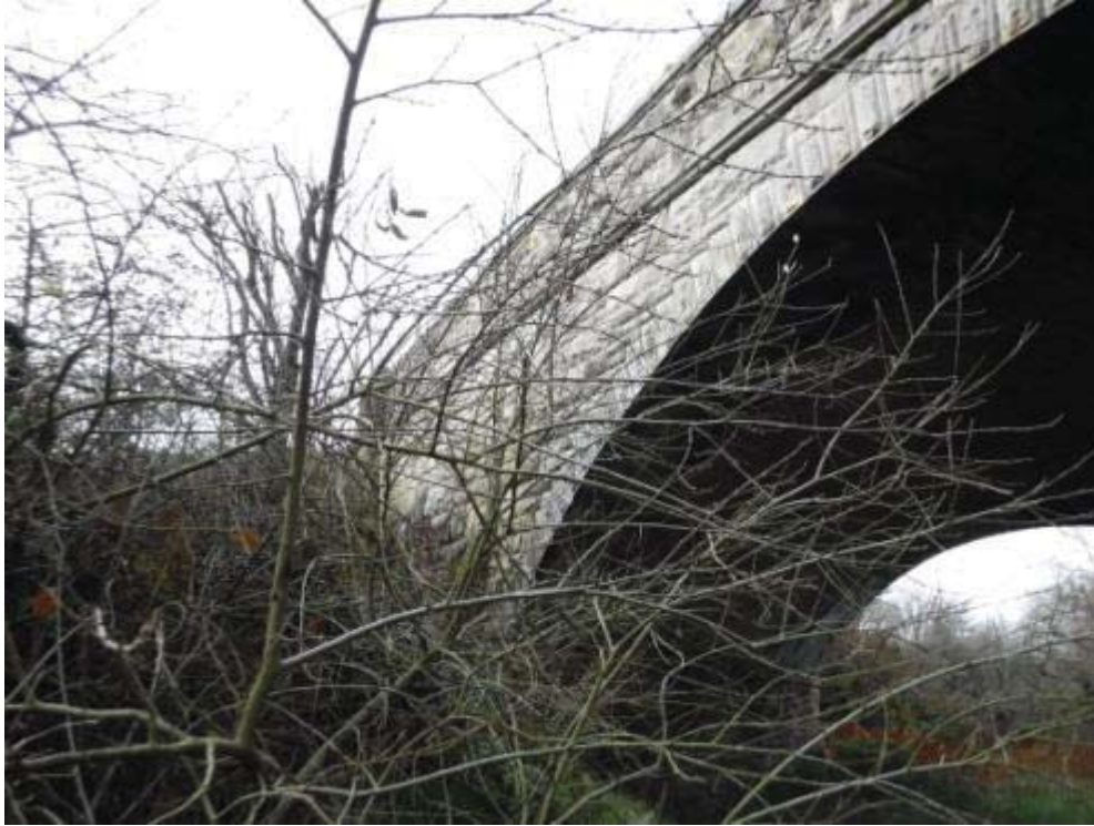
Photo No.47 - South spandrel: S/W view.
