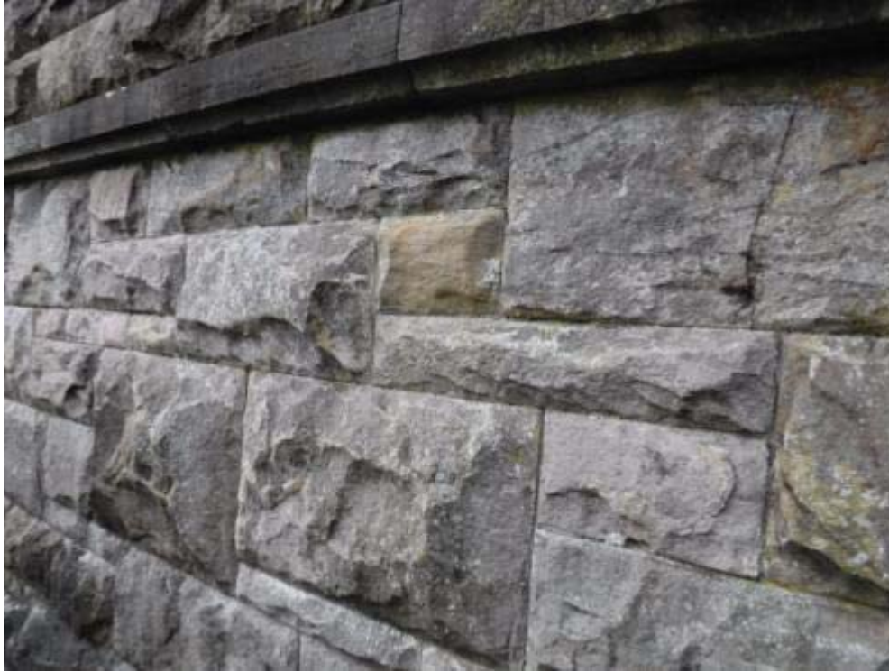
Photo No.89 - S/E wing wall: Typical example of the condition.
