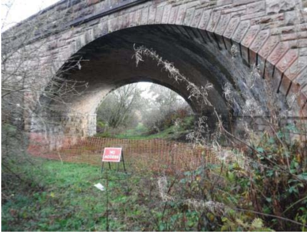
Photo No.25 - North arch ring face: View.
