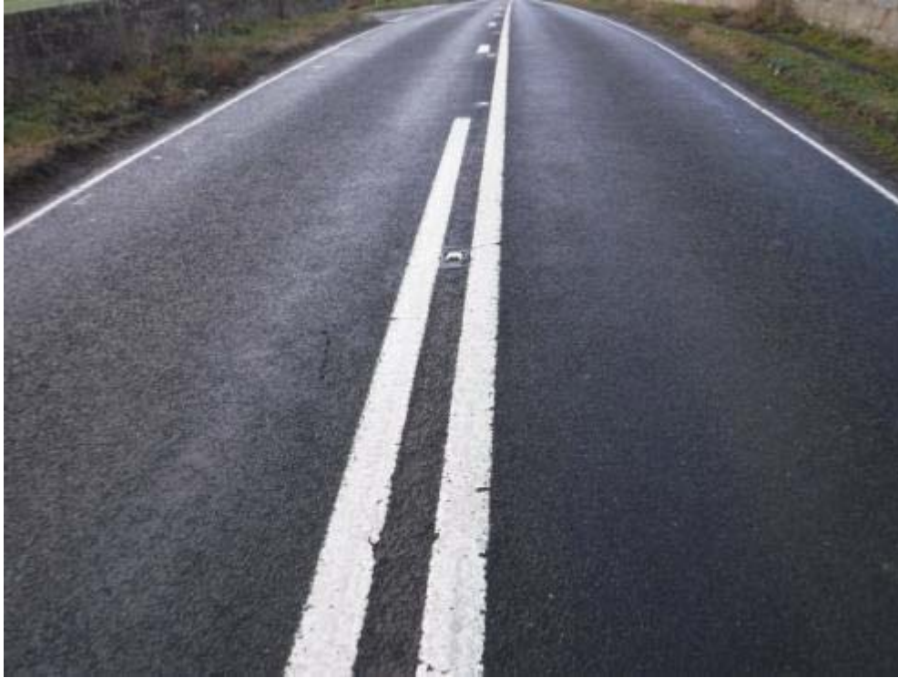
Photo No.163 - Road surface: Typical example of the condition.
