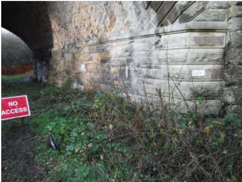
Photo No.62 - East abutment: Typical example of the condition.
