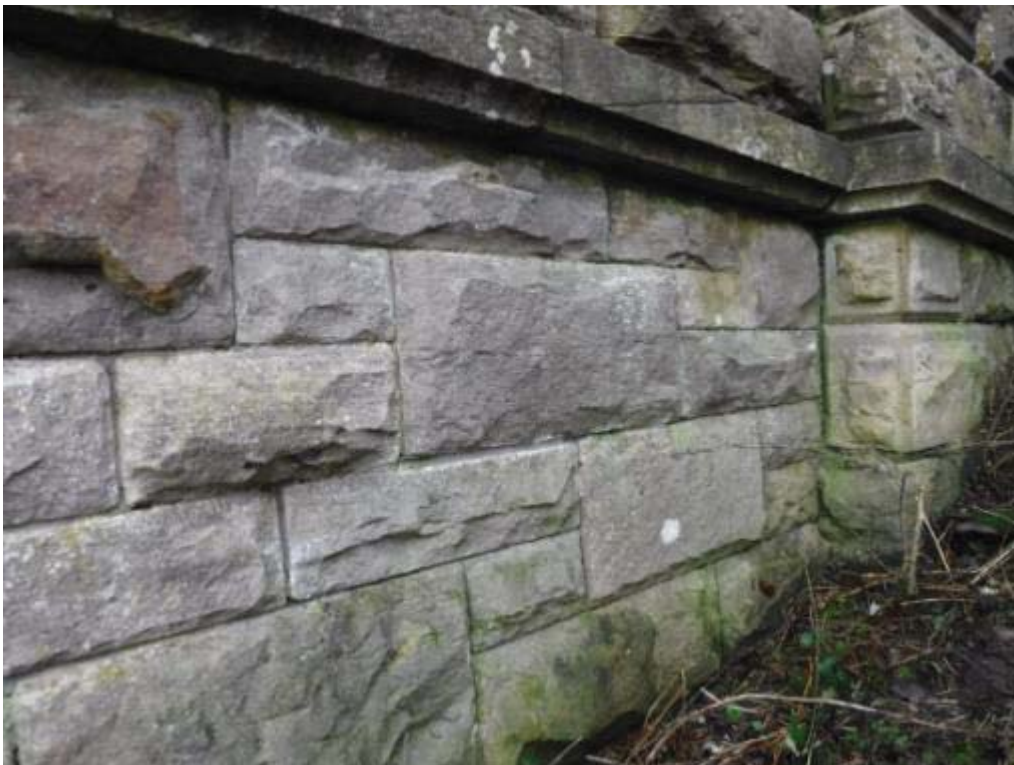
Photo No.88 - S/E wing wall: Typical example of the condition.
