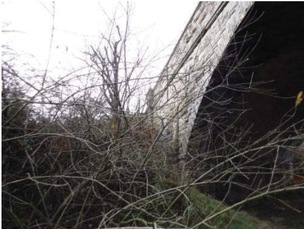
Photo No.94 - S/W wing wall: View
