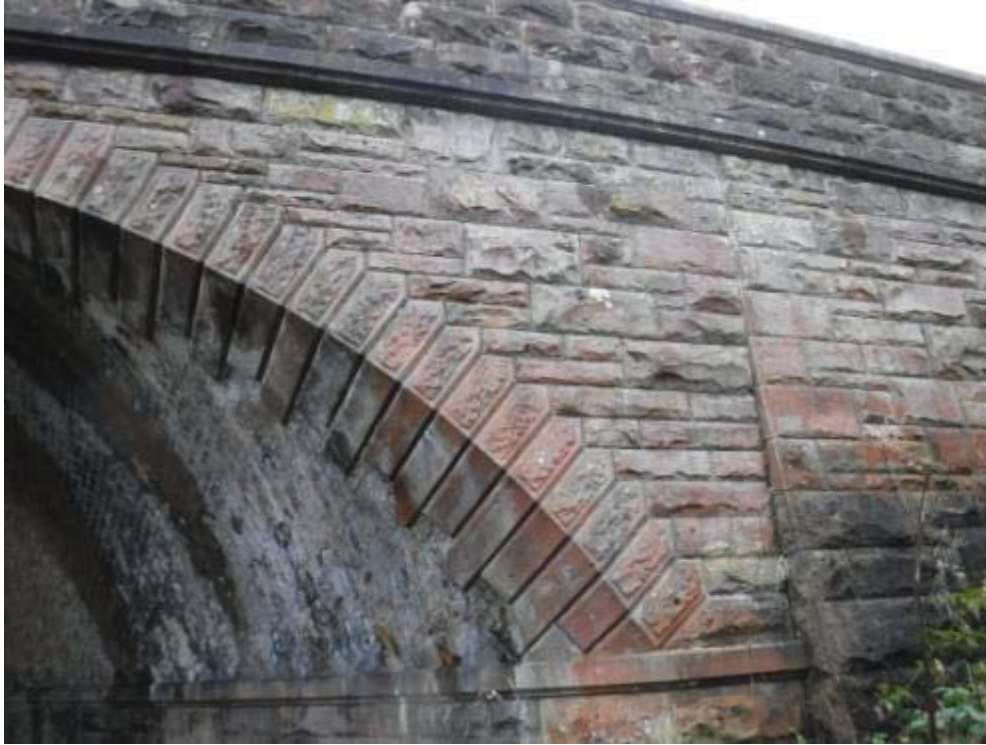
Photo No.37 - North spandrel: N/W view.
