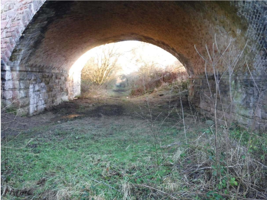
Photo No.8: Area under the structure: Typical example.
