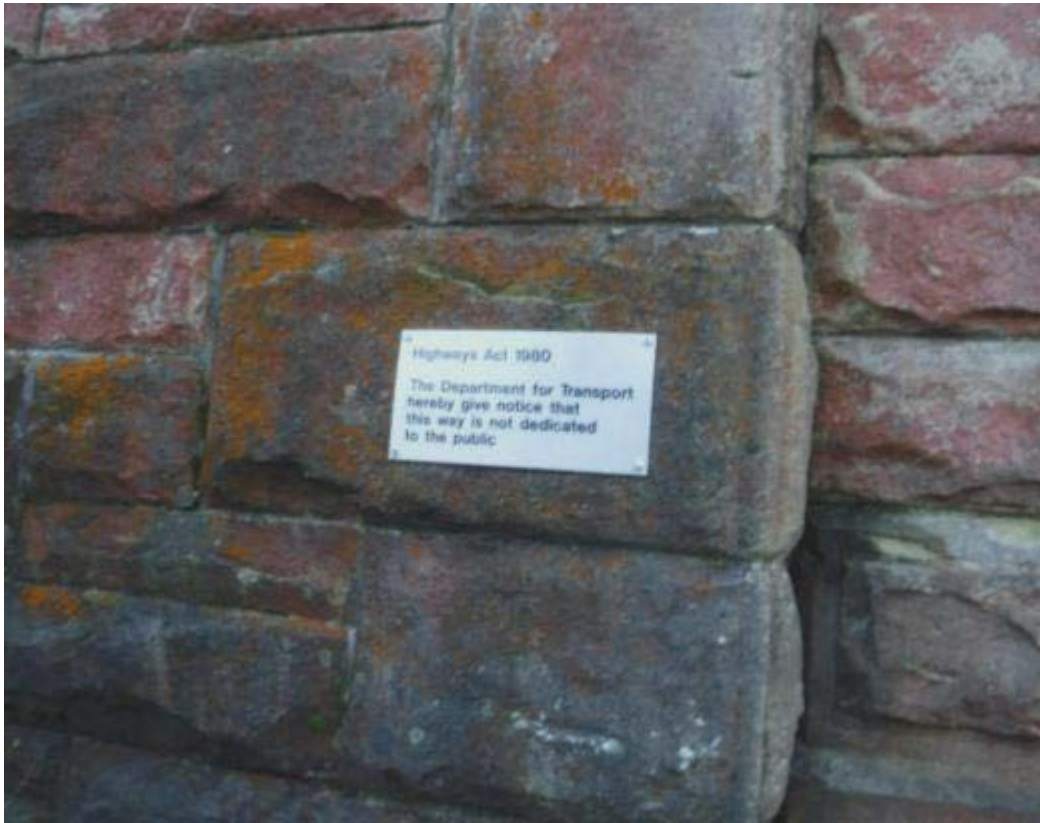
Photo No.4: Non - Dedication plate: Typical example of the condition.
