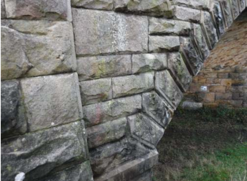
Photo No.53 - South spandrel: Typical example of the condition.
