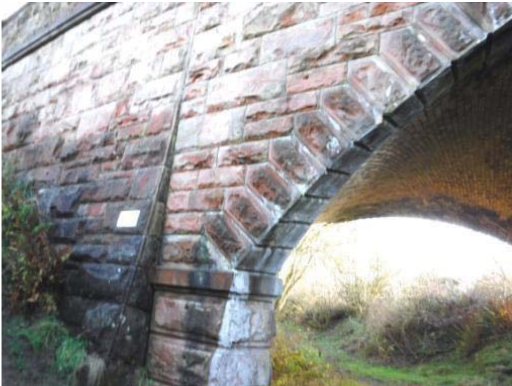
Photo No.34 - North arch ring face: Typical example of the condition.
