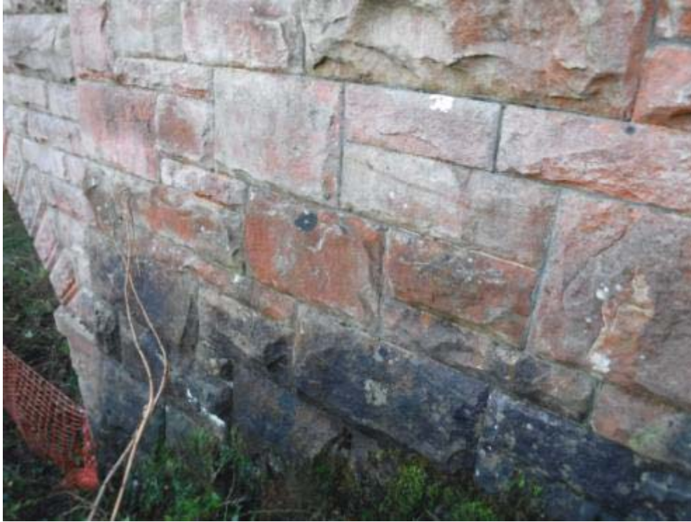
Photo No.85 - N/W wing wall: Typical example of the condition.
