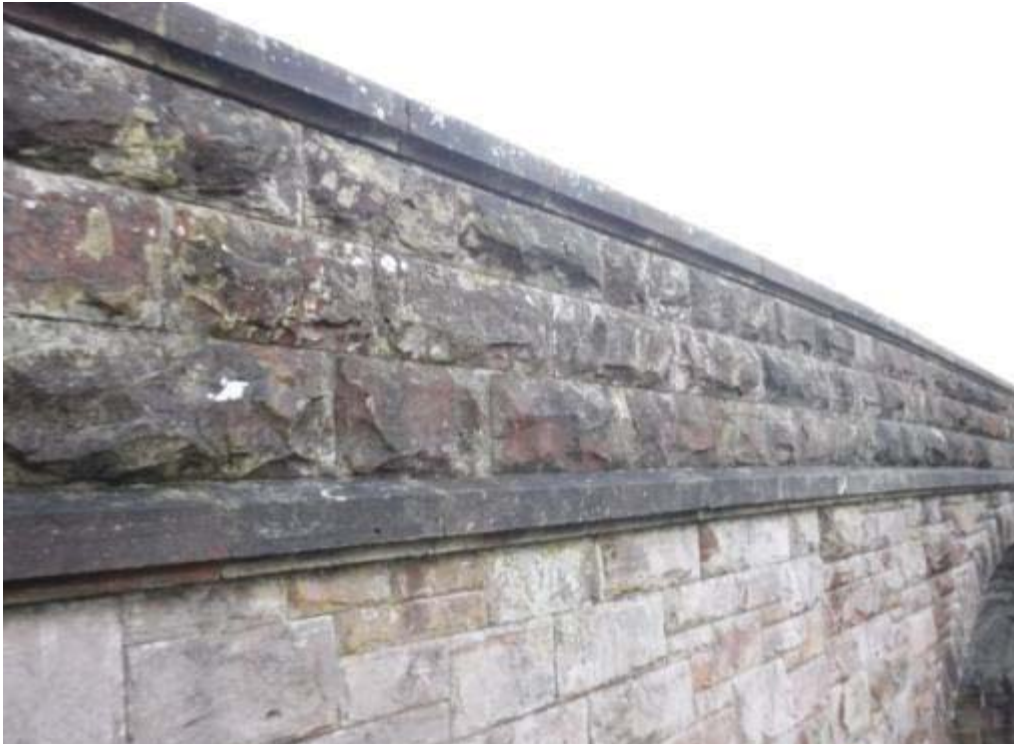
Photo No.123 - North outer parapet: Typical example of the condition.
