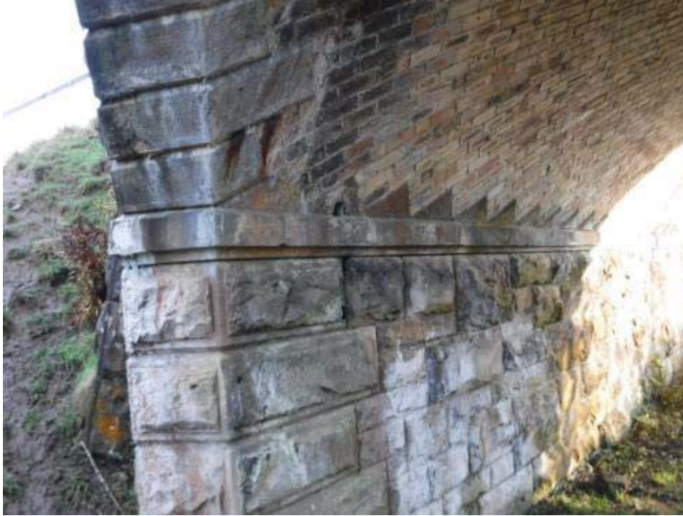
Photo No.149 - East springer course: Typical example of the condition.
