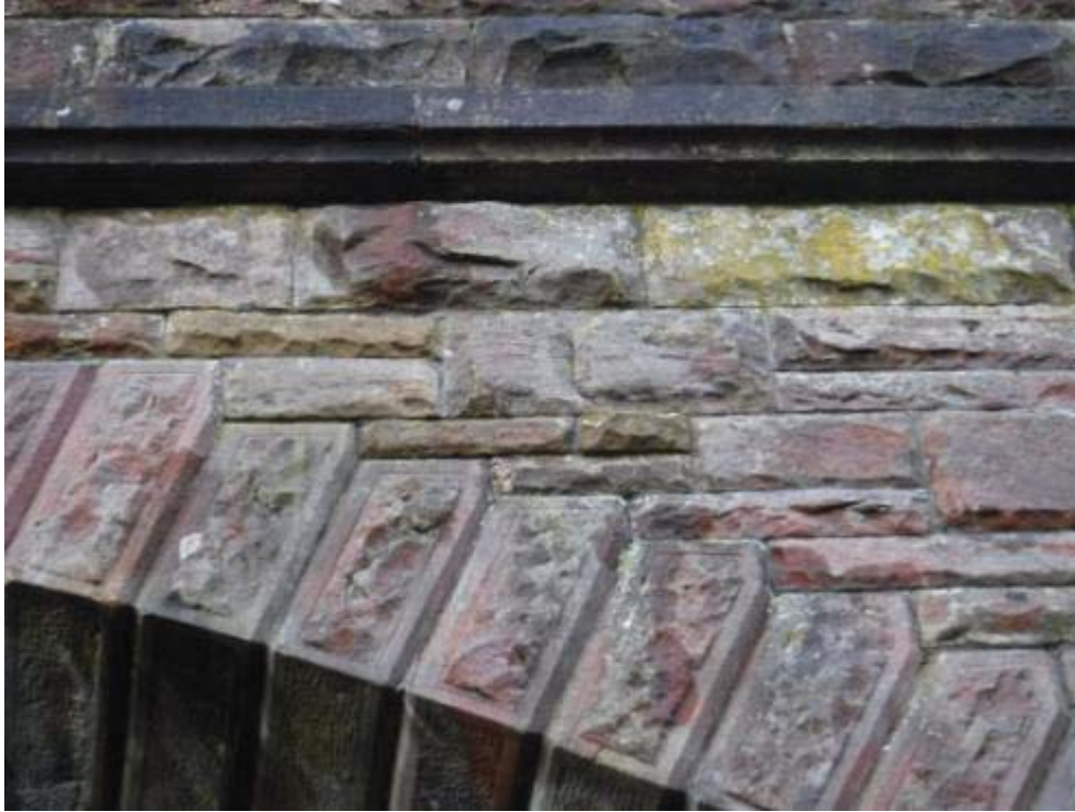
Photo No.39 - North spandrel: Previous stonework repairs at the N/W elevation.
