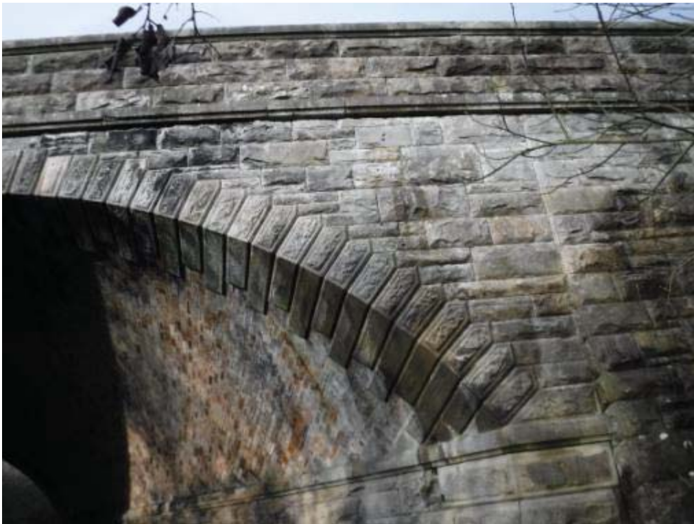
Photo No.46 - South spandrel: S/E view.
