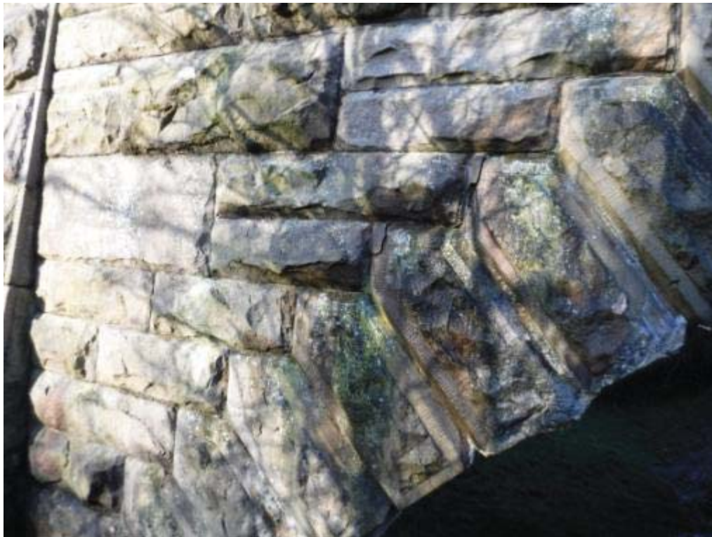
Photo No.18 - South arch ring face: Typical example of the condition.
