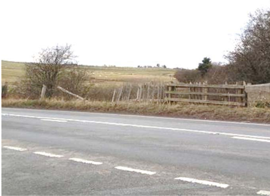
Photograph 16: general condition of the northwest fence line
