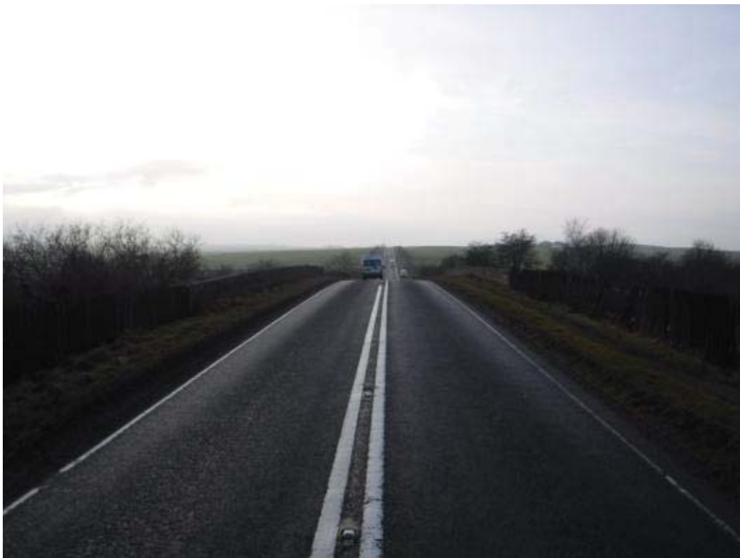
Photo No.5: View: Across Structure.
