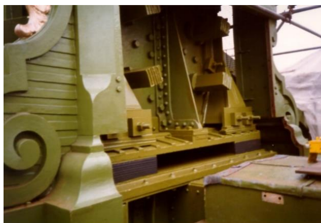
Figure 6.11: Tower top saddle showing replacement elastomeric bearings (Source: AECOM)
