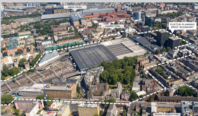
Aerial showing the Euston Area, Draft Euston Planning Brief (2020), Camden Council
