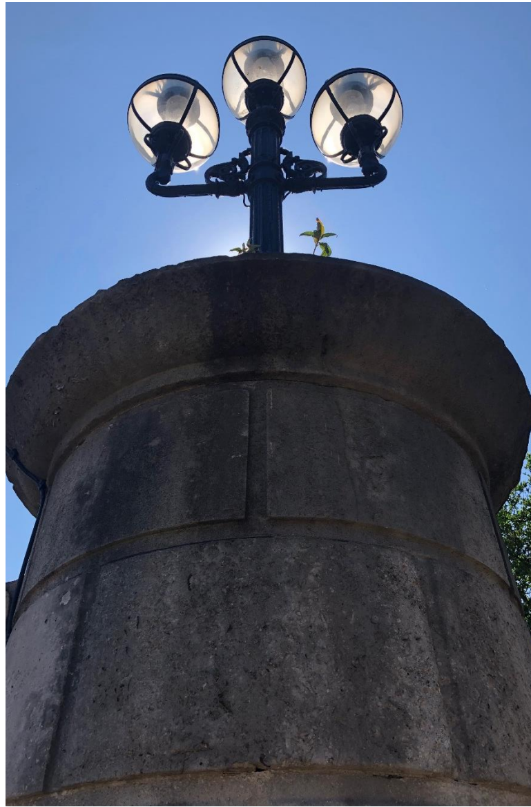
Portland stone bridge pier and lamp
