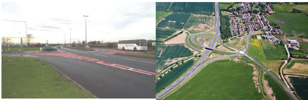
Figure 9 Long Newton Junction before and after the intervention
