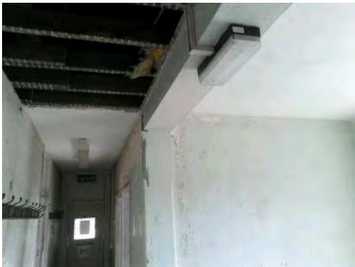
Sample 26: Building 142. First Floor. 104. Textured coated plasterboard ceilings above stairs and end of corridor
