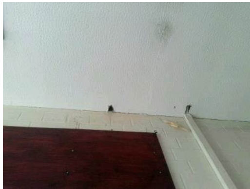
Ref. Sample 3: Building 142. Ground Floor. 004. Textured coated plasterboard ceiling
