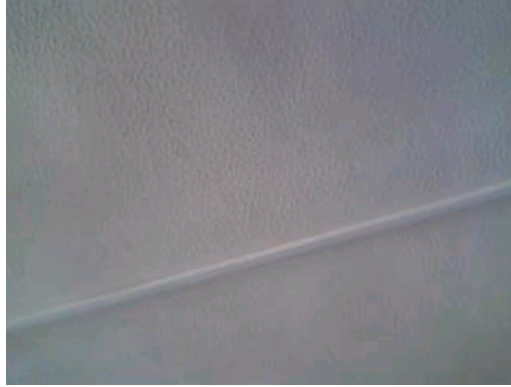
Ref. Sample 76: Building 165. First Floor. Room 39. Textured coating to ceiling
