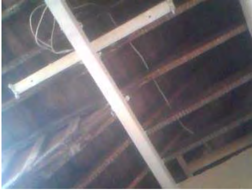
Ref. Sample 112: Building 165. Second Floor. Room 67. Textured coating to wooden beam
