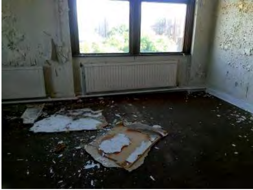
Sample 38: Building 142. First Floor. 115. Cement panels beneath windows
