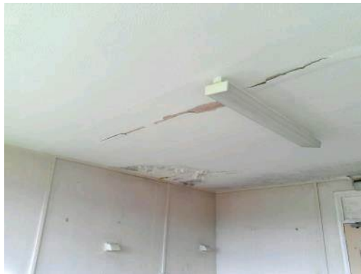
Sample 37: Building 142. First Floor. 114. Textured coated ceiling and associated debris to floor
