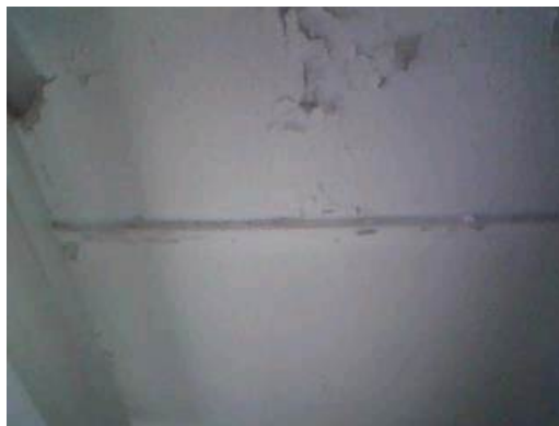
Sample 76: Building 165. First Floor. Corridor 4. Textured coating to ceiling
