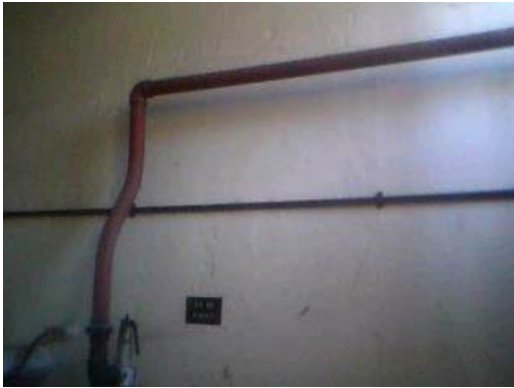
Sample 3: Building 165. Ground Floor. Boiler House. Residue to walls
