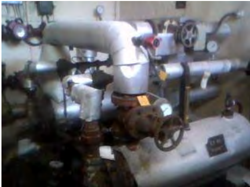
Sample 5: Building 165. Ground Floor. Boiler House. Gaskets to pipework
