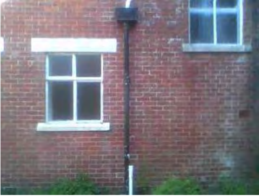
Sample 59: Building 165. External. Courtyard. Cement downpipe
