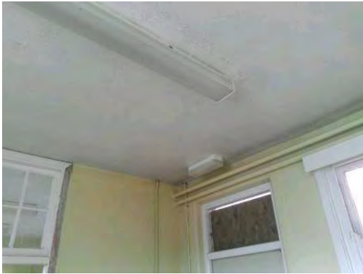
Sample 2: Building 142. Ground Floor. 001. Textured coated plasterboard ceiling
