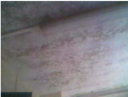
Ref. Sample 94: Building 165. First Floor. Room 53. Textured coating to ceiling
