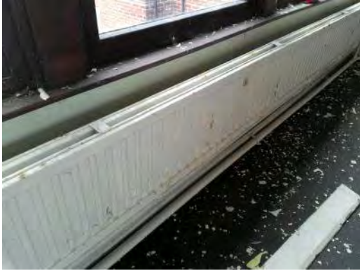
Sample 28: Building 142. First Floor. 109. Cement panels beneath windows
