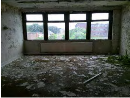
Sample 35: Building 142. First Floor. 113. Cement panels beneath windows
