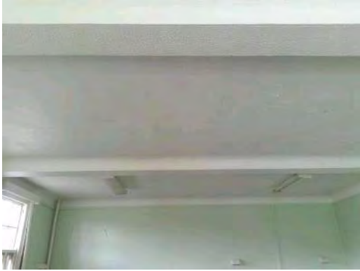
Sample 11: Building 142. Ground Floor. 013. Textured coated plasterboard ceiling
