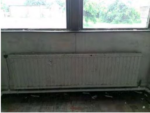
Sample 23: Building 142. Ground Floor. 019. Cement panelling beneath windows
