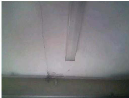
Sample 83: Building 165. First Floor. Toilets 40. Textured coating to ceiling
