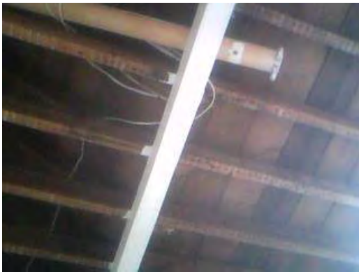
Sample 112: Building 165. Second Floor. Room 64. Textured coating to wooden beam
