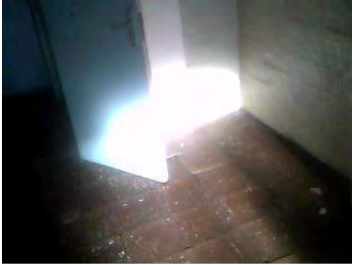
Sample 35: Building 165. Ground Floor. Room 22. Floor tiles
