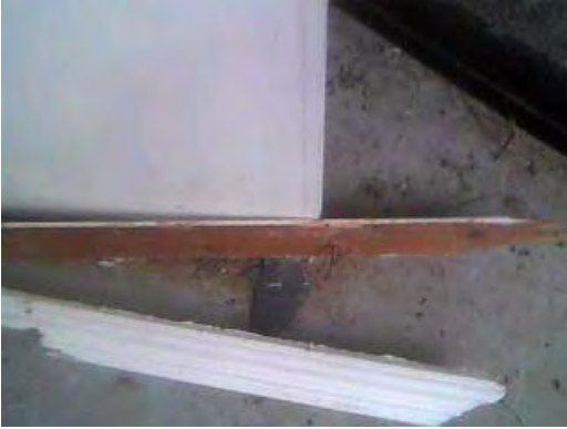
Sample 119: Building 165. Second Floor. Room 72. Cement tile debris
