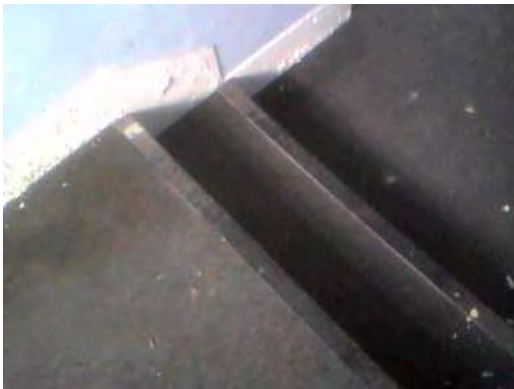
Sample 77: Building 165. First Floor. Corridor 4. Stair nosing
