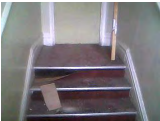
Sample 75: Building 165. First Floor. Toilets 34. Stair nosing
