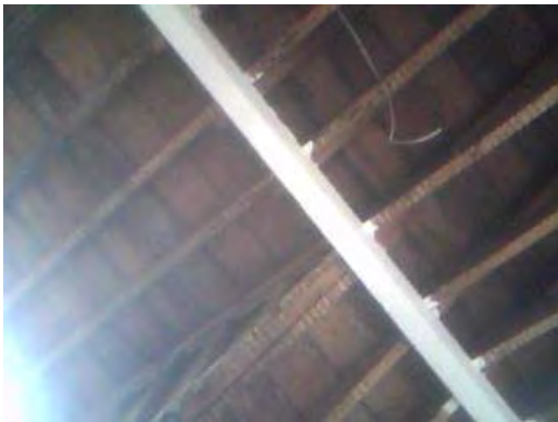
Sample 115: Building 165. Second Floor. Room 69. Textured coating to wooden beam
