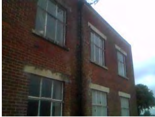
Sample 132: Building 165. External. Main Building. Cement downpipes
