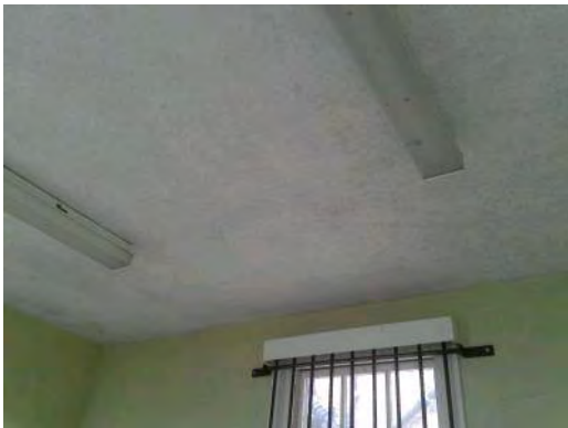
Sample 3: Building 142. Ground Floor. 003. Textured coated plasterboard ceiling
