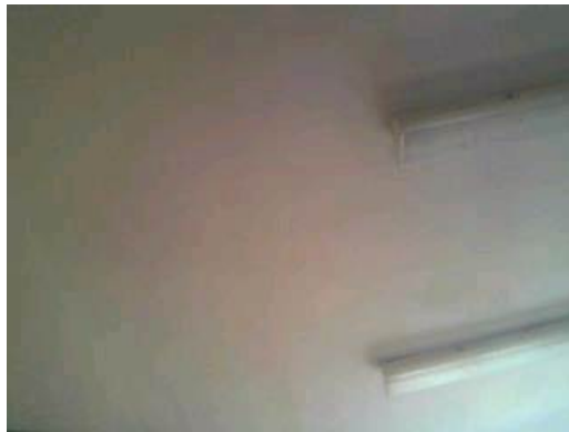
Ref. Sample 100: Building 165. First Floor. Room 59. Textured coating to ceiling
