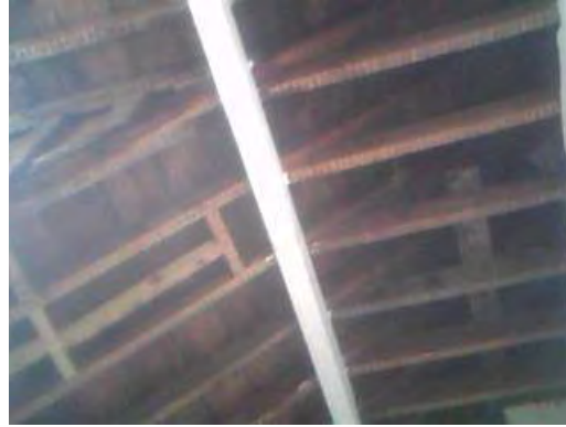
Ref. Sample 112: Building 165. Second Floor. Room 73. Textured coating to wooden beam
