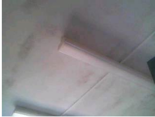
Ref. Sample 94: Building 165. First Floor. Room 52. Textured coating to ceiling
