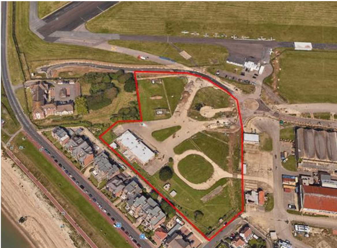
Figure 2. Plan view of the area surveyed within red line boundary.
