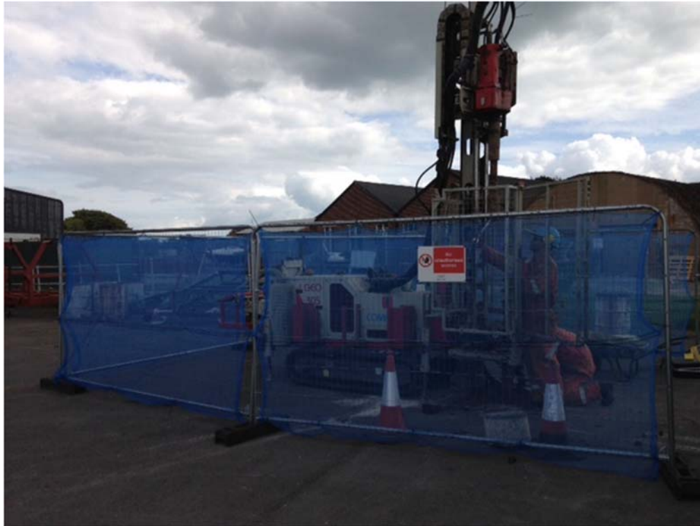
Borehole installation at CELBH04
