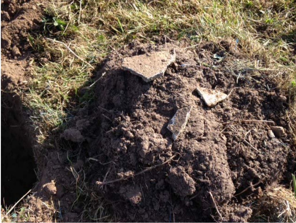
Asbestos containing materials identified within shallow soils at the hand pit location to the south of Implacable Road
