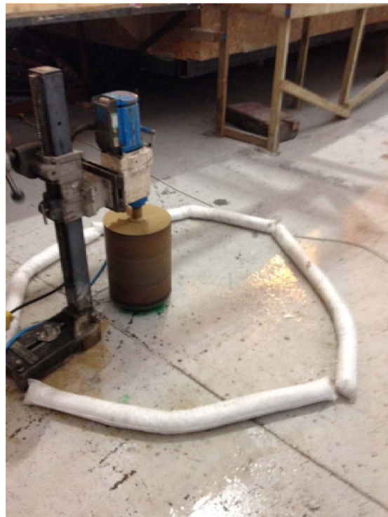
Concrete coring inside of Dunning Hanger
