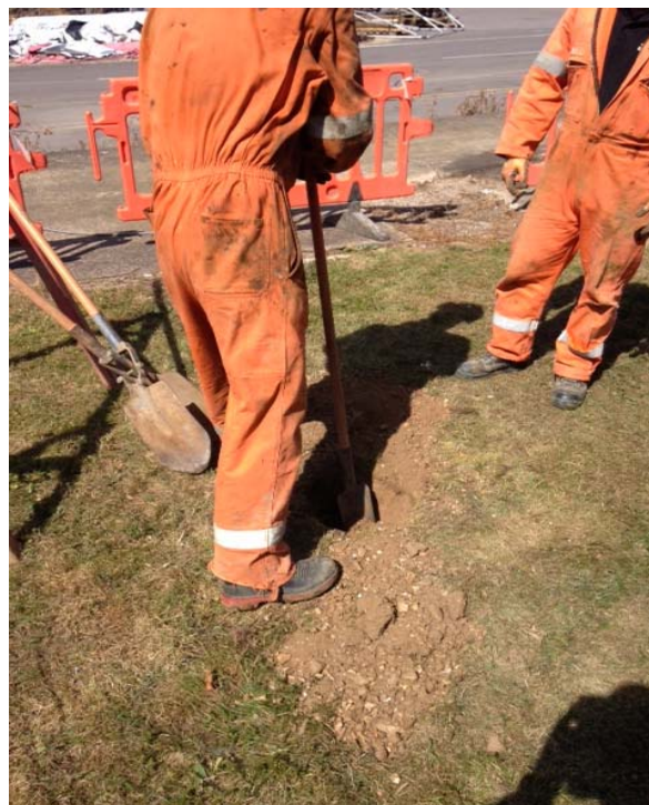
Hand pitting within former vehicle refueling area
