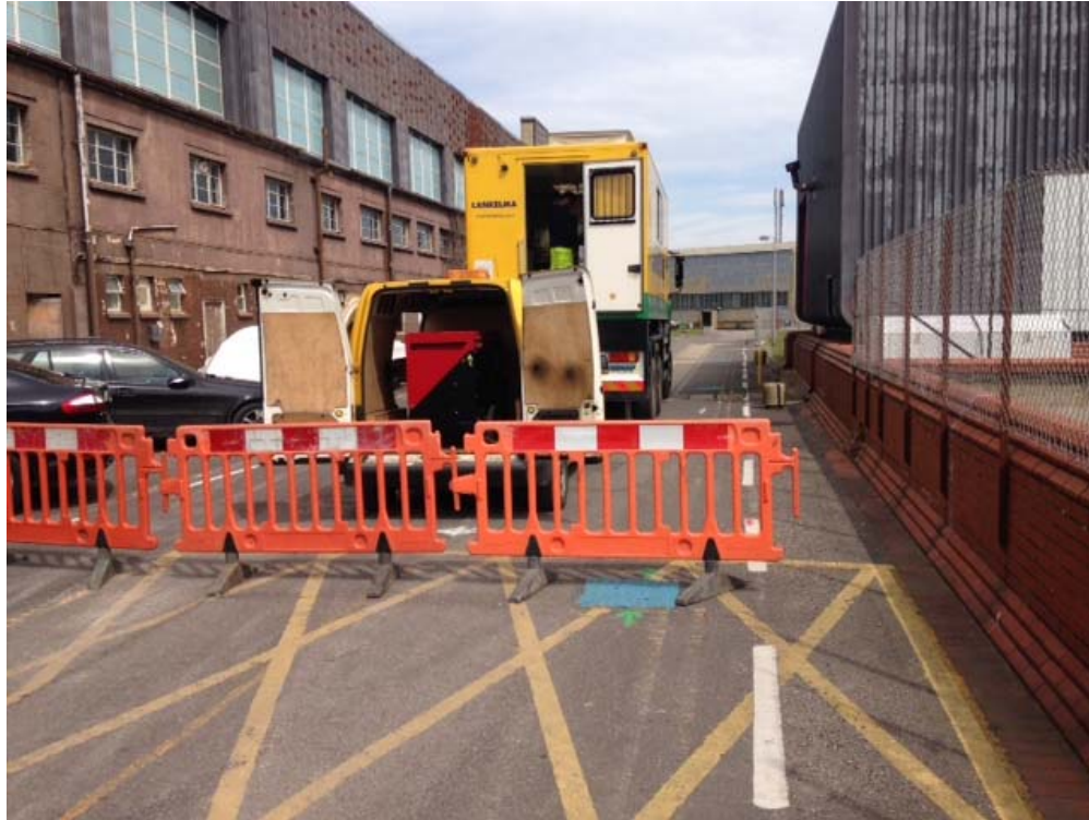
MIP testing at location MIP11 between Dunning Hanger and the Boiler House
