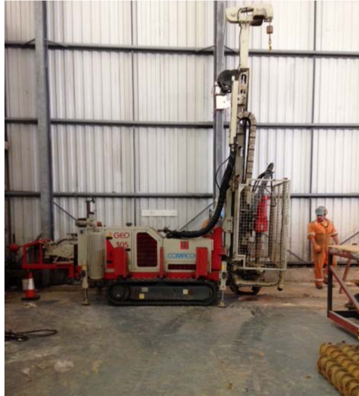
Borehole installation at CELBH02 within Dunning Hanger
