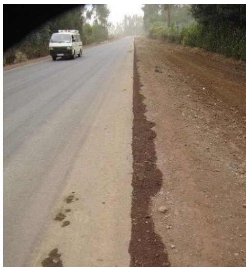
Figure 6-5: Infiltration of water through a permeable surfacing
