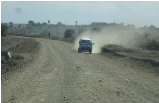
Dusty and rough due to oversize material
