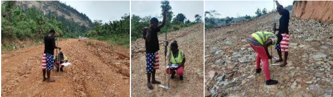
Figure 8 DCP Test being carried out at the Experimental Sections
