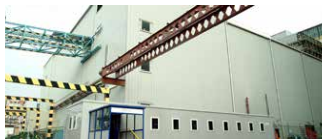
Magnox Reprocessing Plant - Sellafield
