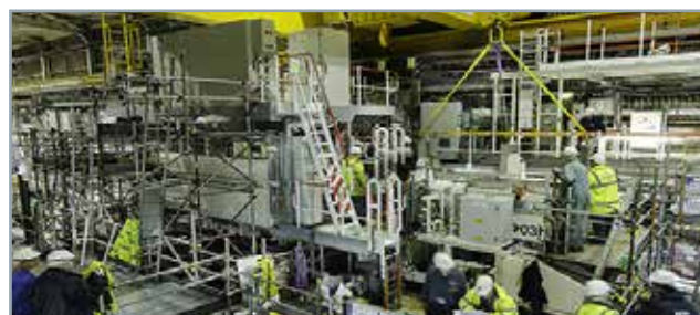
Emptying machine installation at the MSSS
