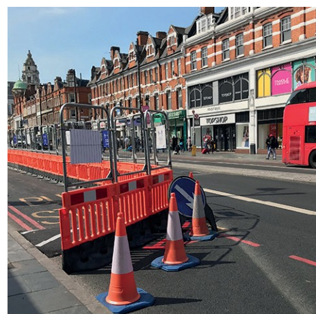
Figure 33: Footway widening outside station entrance – London
