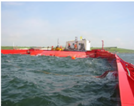
“Wave Dragon” – wave turbine installation- recommended colour above the water is yellow. (Photos courtesy Wave Dragon Ltd).
