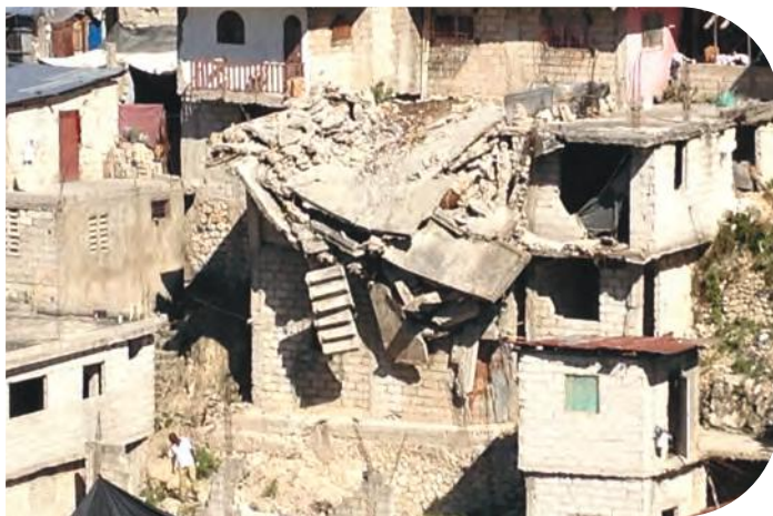
Infrastructure damage caused by the earthquake in Haiti in 2010. Photo credit: Matthew Hunt
