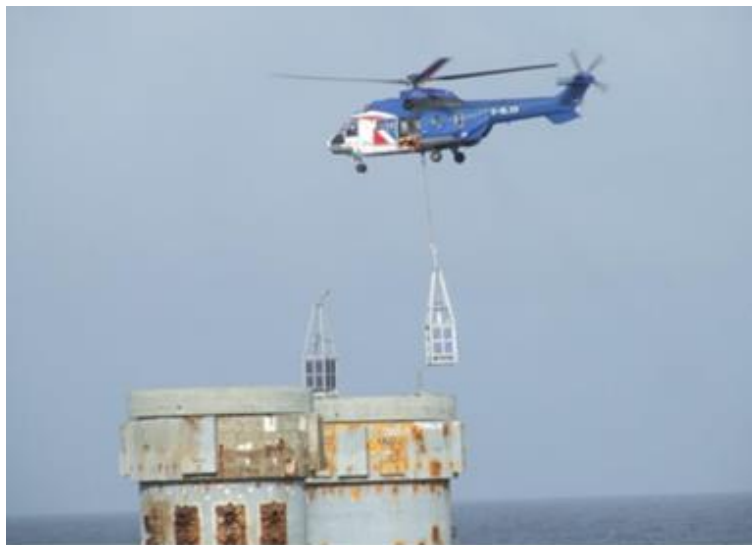
Figure 2-3 AtoN deployment via helicopter
