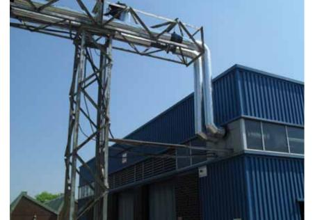
Replacement of insulation to the external high temperature hot water heating system at Boiler House 7, MOD Donnington © CarillionEnterprise
