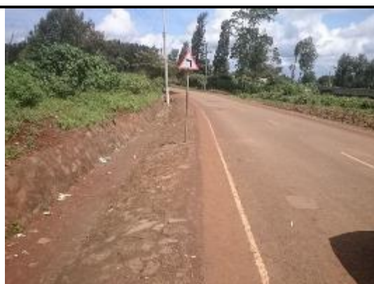
Figure 2-3: Good – Drain lining connected to edge of surfacing
