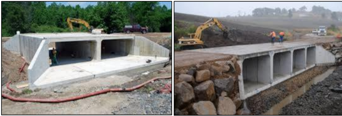
Figure 2-8: Monolithic structure – box culvert
