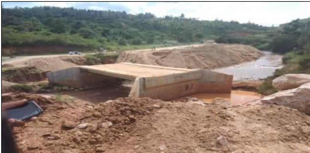
Figure 10: A new bridge under construction (Kiamara junction bridge to Gitugi)
