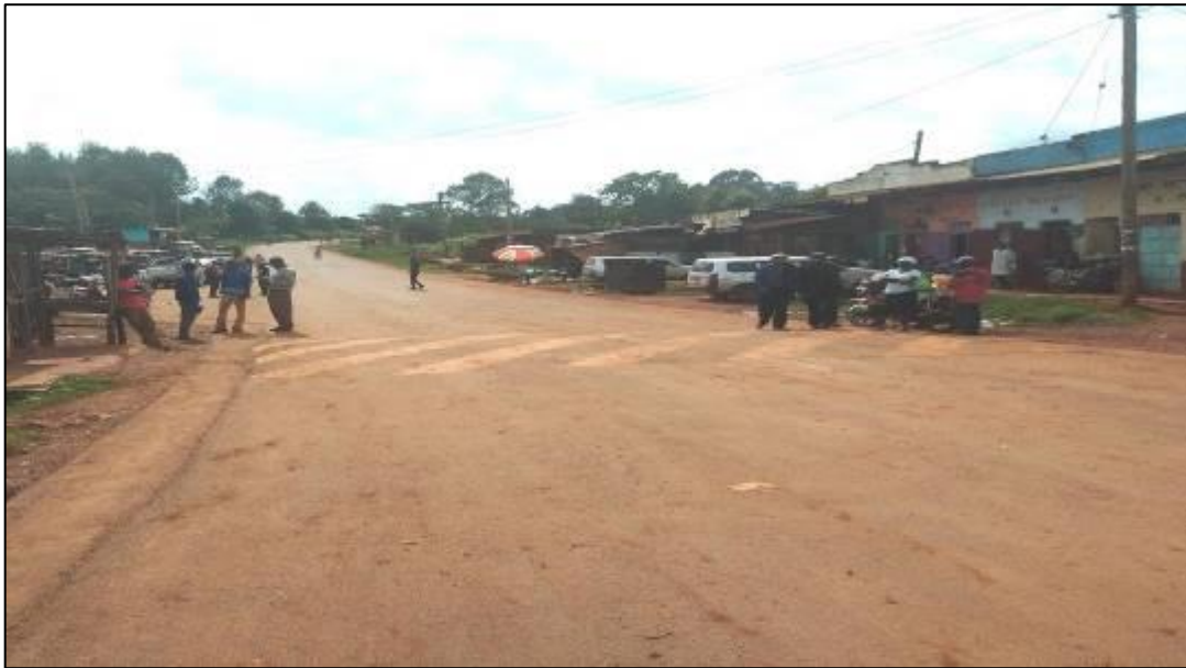
Figure 4: Gitugi-Kiamara Road Upgrading
