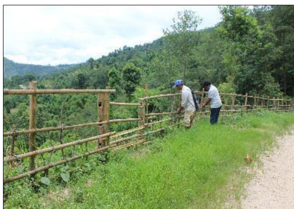
Photo 2: Low Cost Fence erection at Site #1, 2018
