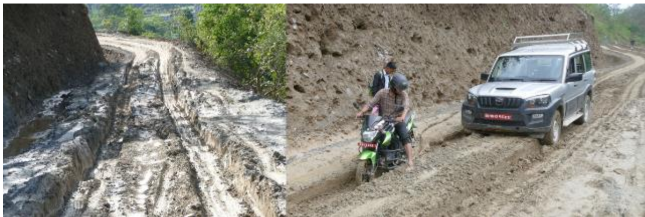
Figure 15 Muddy section close to Bhoredovan on the section to Khahereghat
