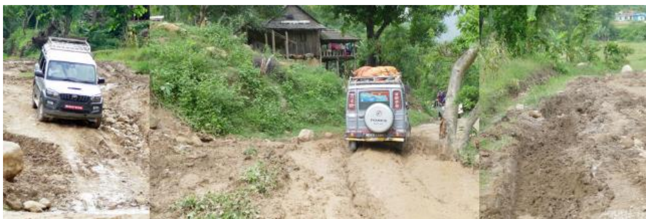
Figure 30 Muddy sections of the road caused by water running onto the road
