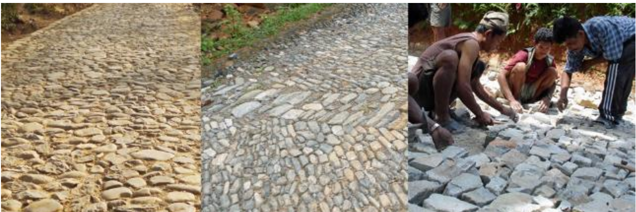
Figure 22 Different cobblestone sections in 2012 (left) and 2019 (centre) and laying cobblestones in 2009
