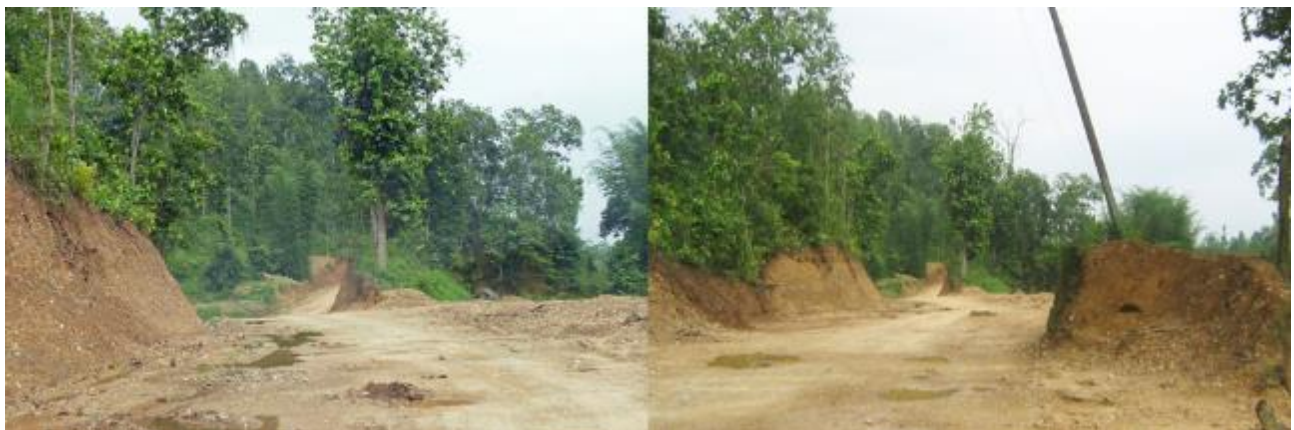
Figure 23 Recently widened section of the road close to Bhimasthan
