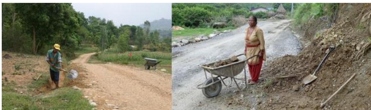
Figure 17 DRSP lengthworker in 2009 (left). Lady voluntarily clearing landslip into a side drain in 2019 (right)
