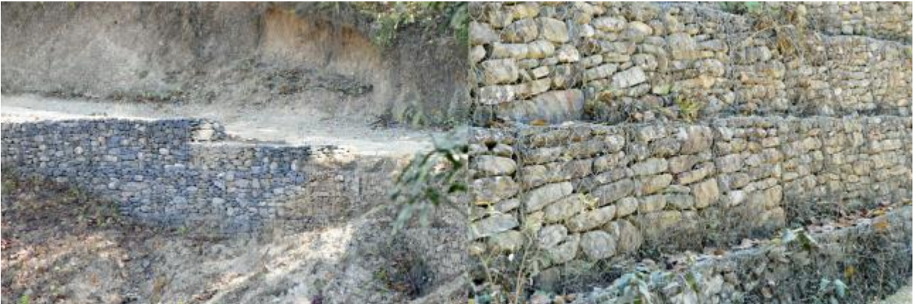
Figure 26 Retaining walls made with stone gabions
