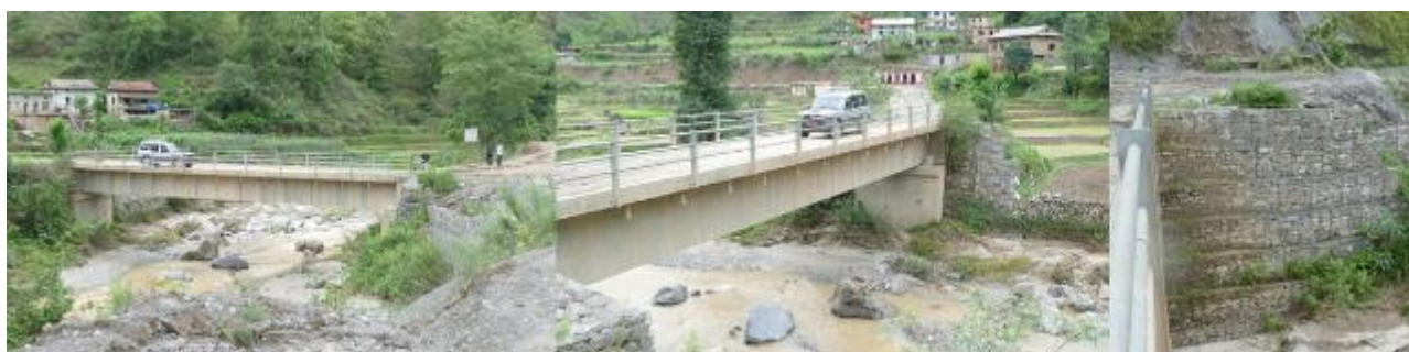
Figure 13 Jhiu Khola bridge at Bhoredovan
