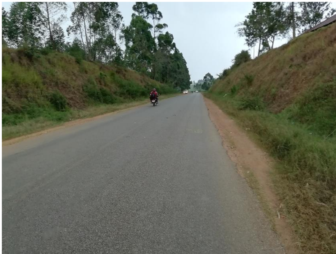
Figure 11 Good-performing inverted Double Surface Dressing on Ishaka - Katunguru
