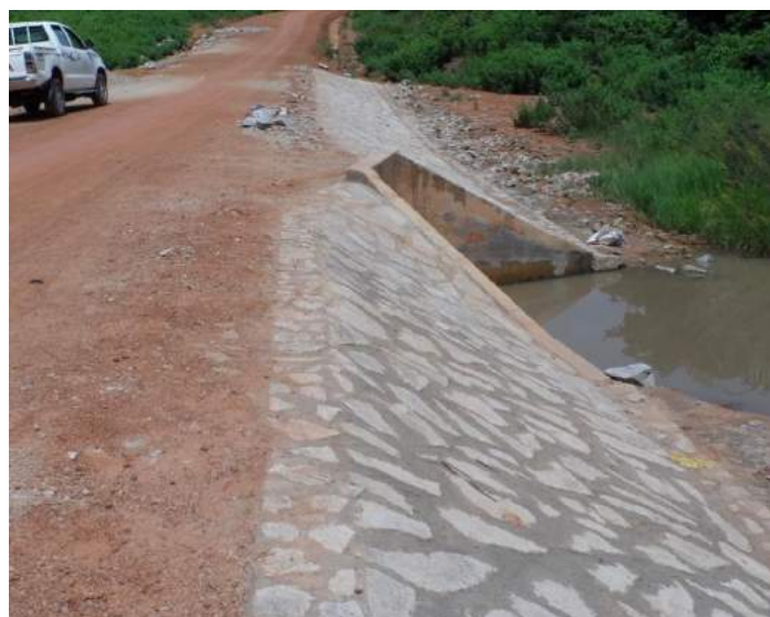
Figure 20 Grouted stone embankment protection of erodible material
