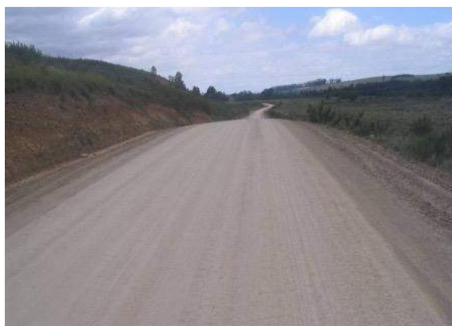
Figure 7 Typical gravel road showing shaped structure and gravel wearing course
