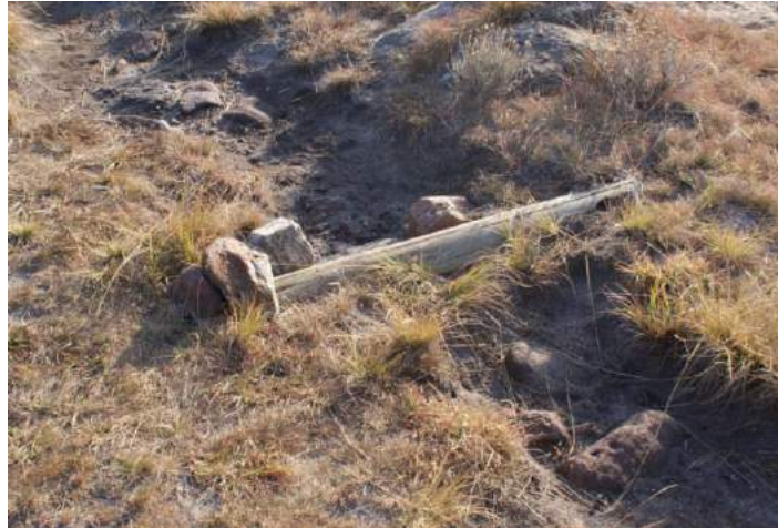
Figure 33 Log scour check
