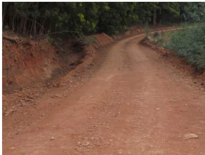
Figure 6 Typical engineered earth road showing shaped structure and side drains
