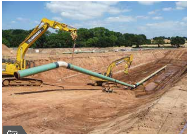
Gas main diversion, Phase One Area North, 2018.
