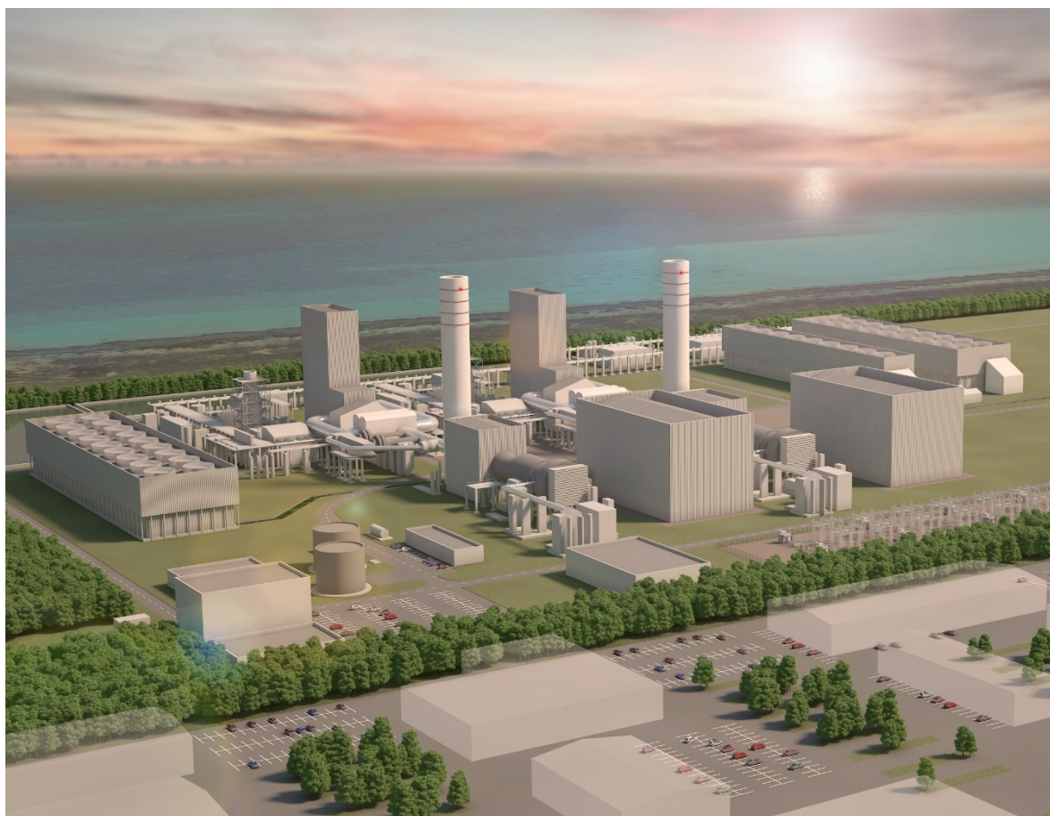
Figure 1. Typical impression of two 1x1 H-Class CCGTs with post-combustion carbon capture
