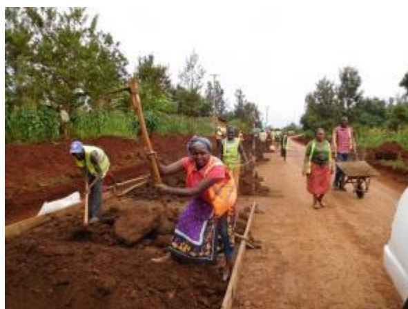
Fig 1. Women employed in labour-intensive road construction in Kenya, 2016
