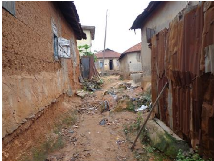
Figure 6: Poor access road to dwellings in Moniya, a slum community in Akinyele LGA
